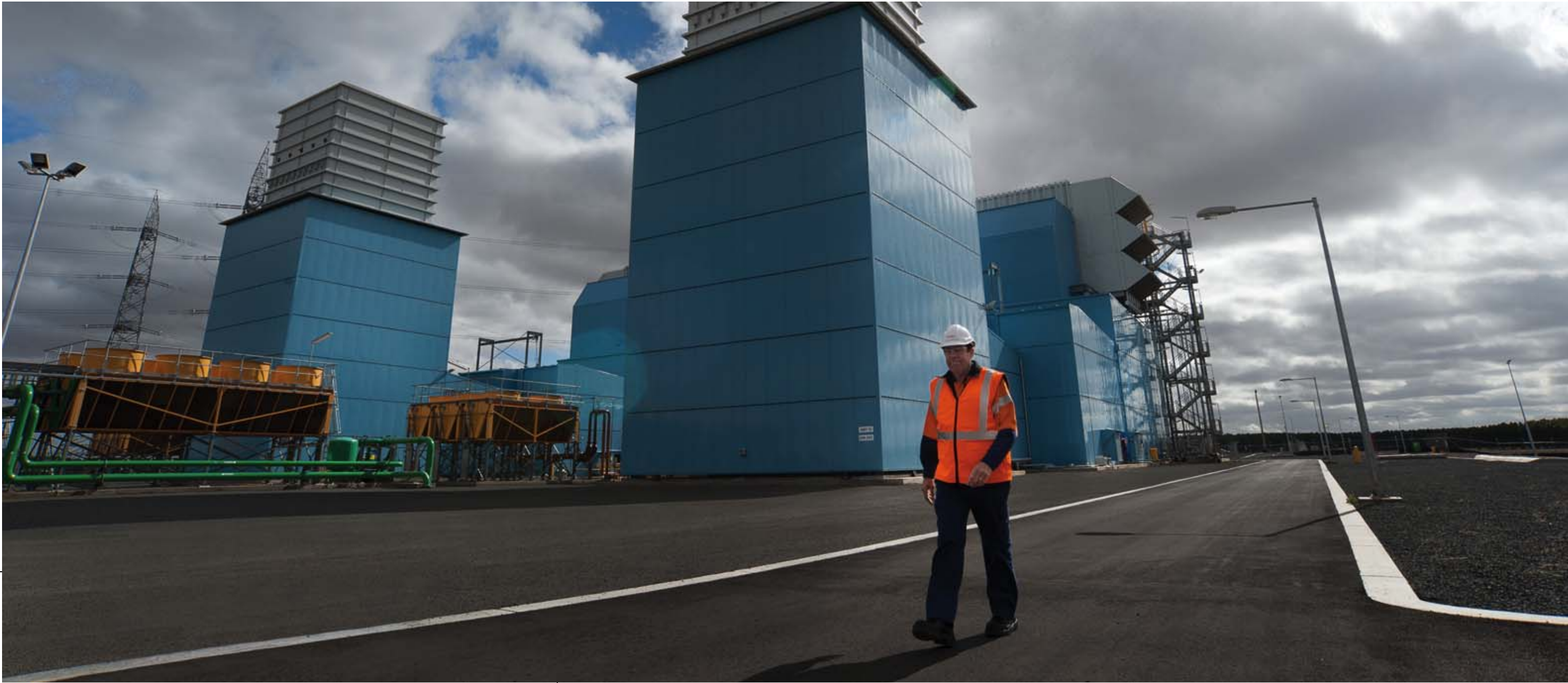
Mortlake Power Station (Origin Energy)
