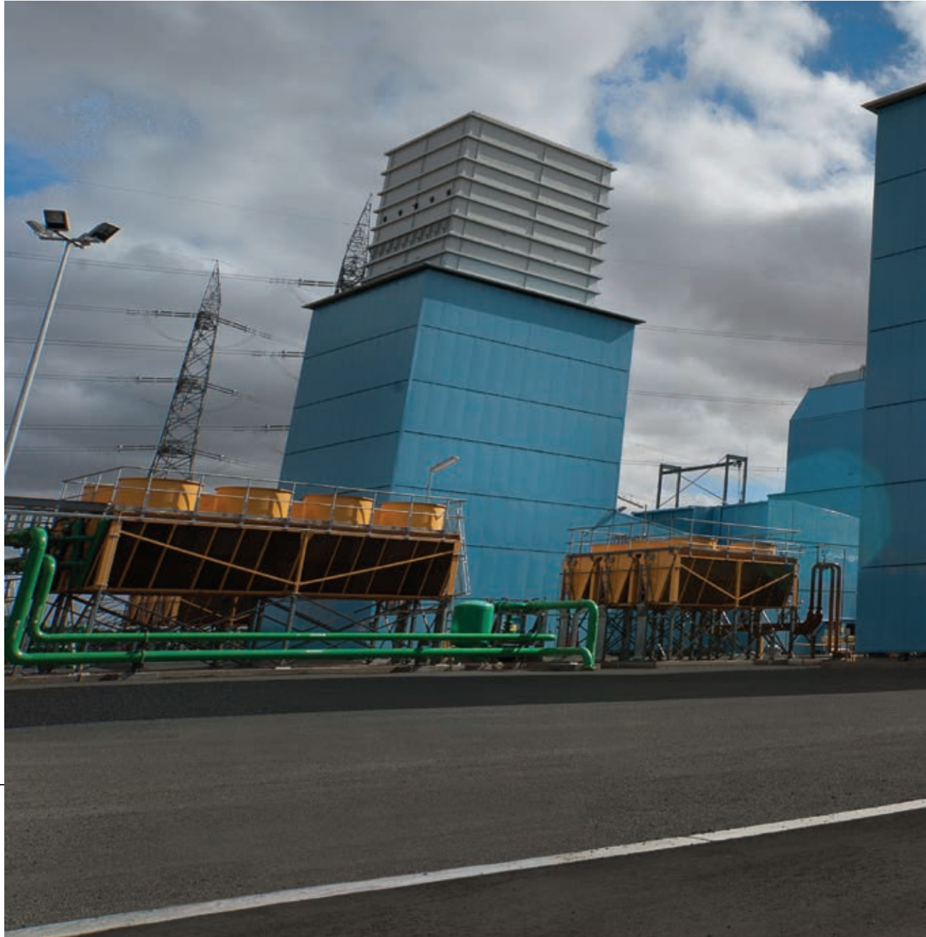
Mortlake Power Station (Origin Energy)
