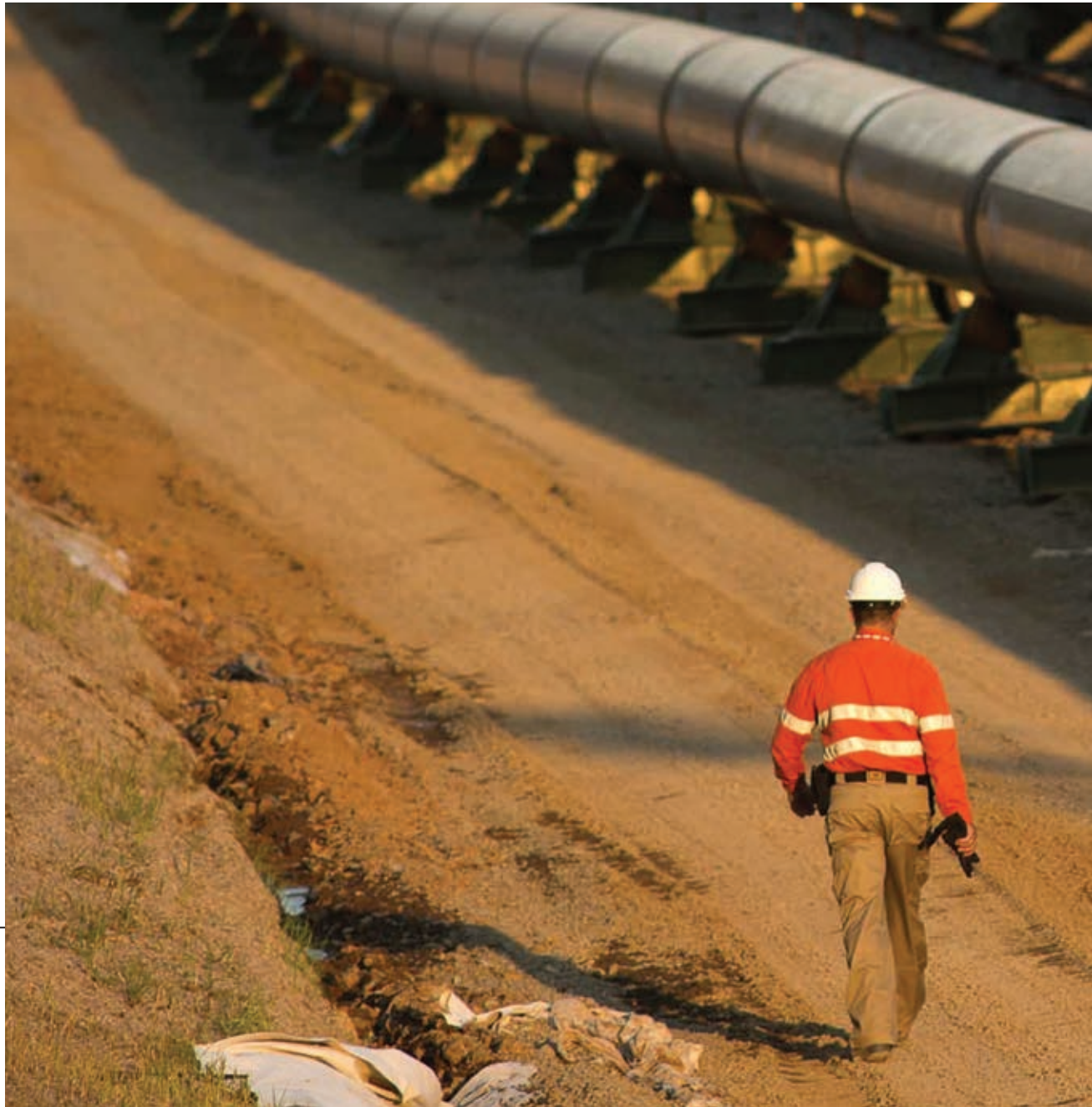
Construction of the QCLNG Pipeline (BG Group)
