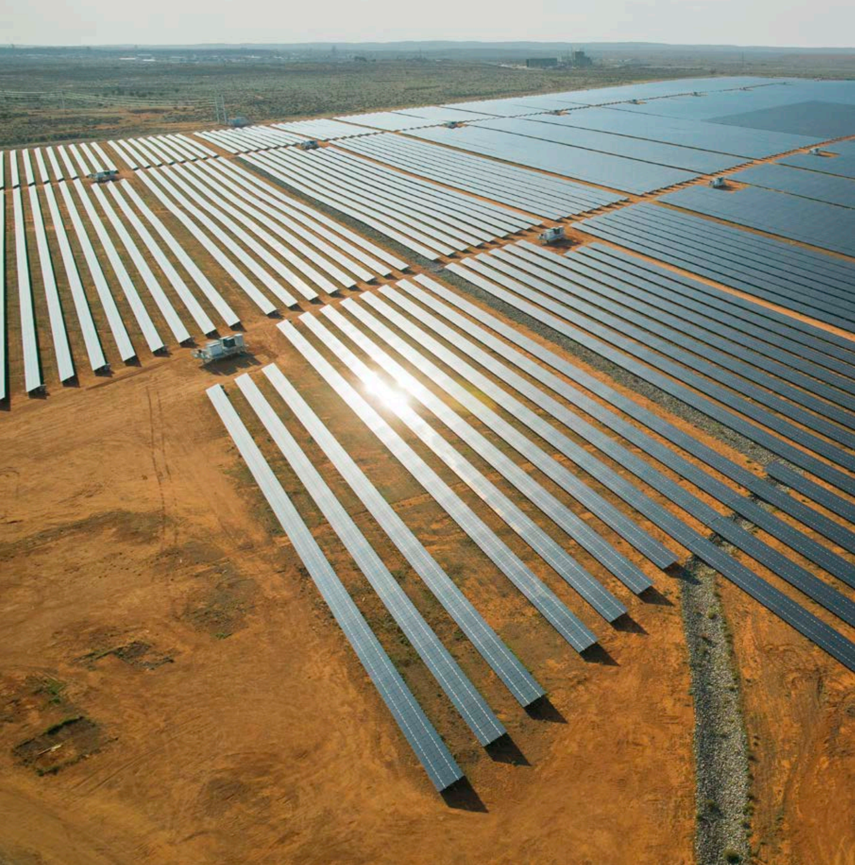
AGL Energy's Broken Hill Solar Plant (image courtesy of AGL Energy)
