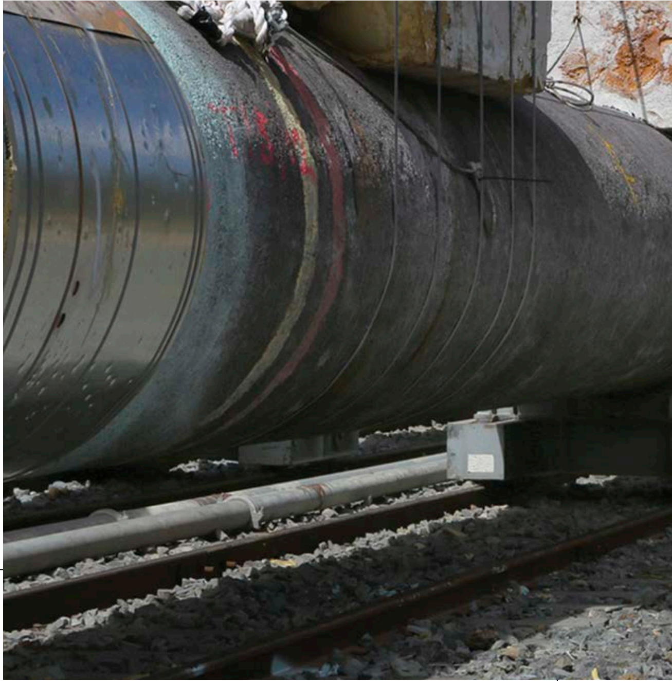
Construction of the Wallumbilla–Gladstone Pipeline (image courtesy of BG Group)
