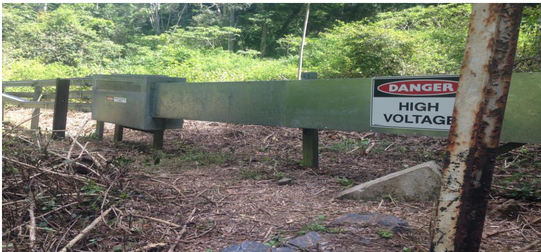
Figure 2-1: Directlink galvanised steel tray
