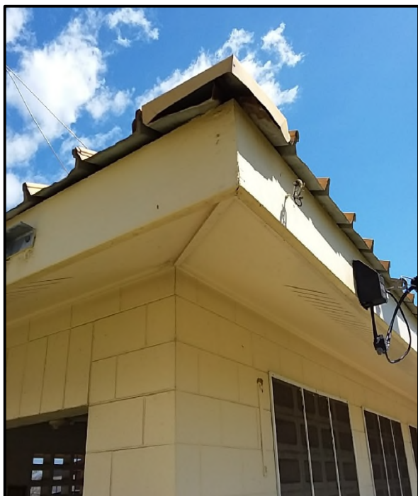
Block 4 – Roofline in disrepair, lack of flashing, uneven ceiling
