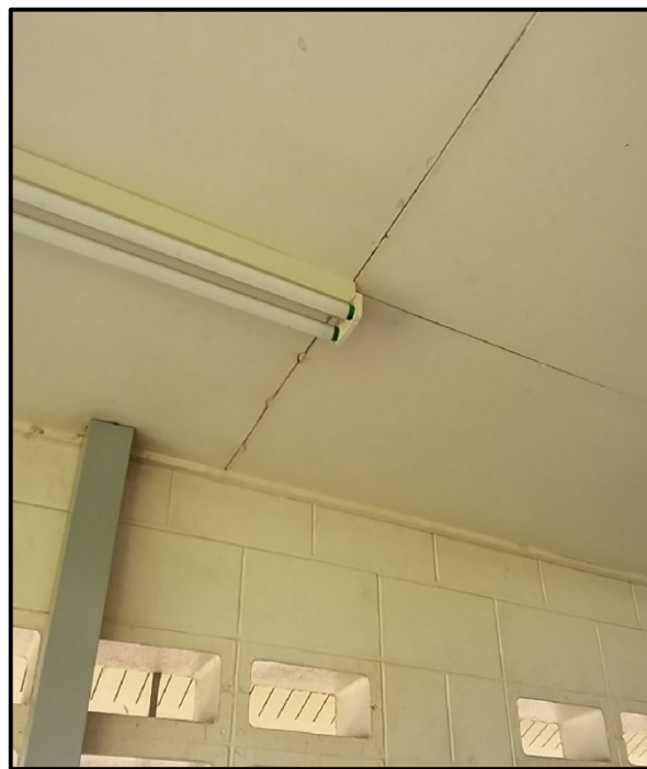
Block 4 – Ceiling panels pulling apart and coming away from beams
