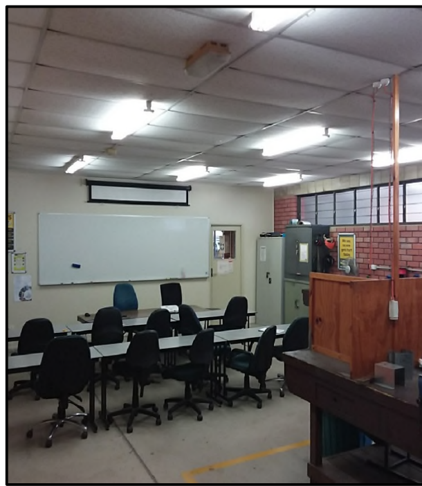
Block 1 Training Room – Warped ceiling tiles across all training rooms show signs of age and disrepair
