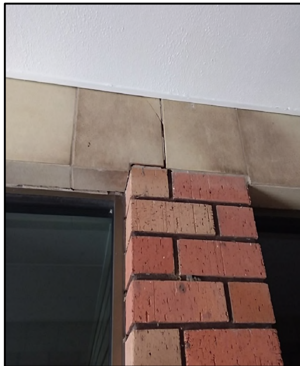
Block 1 – Vertical cracking in tiles & brick work
