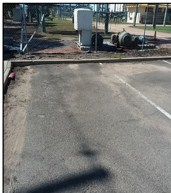
External – Car parking areas show disrepair, considerable cracking, broken guttering and uneven surfaces
