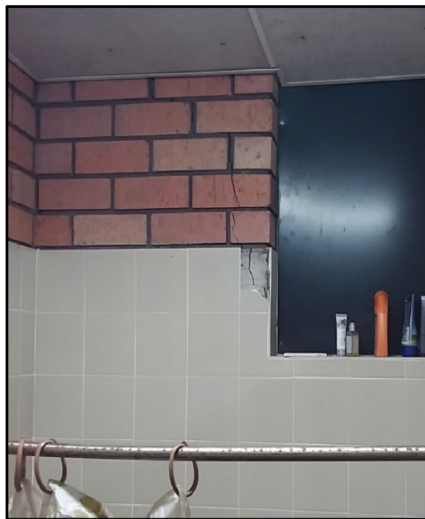
Block 1 Amenities – Vertical cracking down brick walls indicate slab movement
