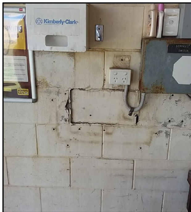
Block 4 – Disrepair on brick work from requirements over time. Rust in electrical switchboard, considerable wear across this building
