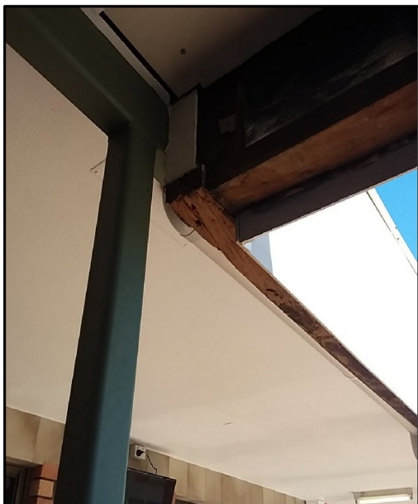
Block 1 - Timber rot within structural support beams from termite damage
