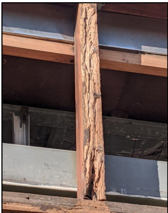
Block 1 - Timber rot within structural support beams from termite damage
