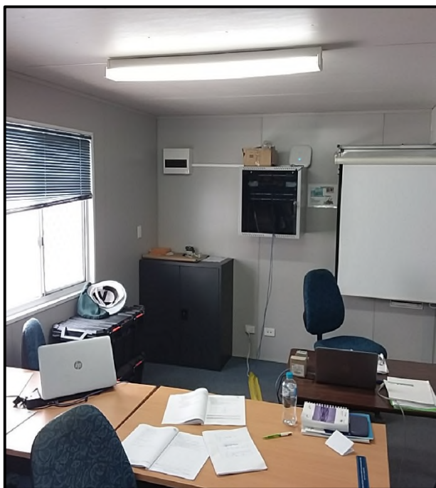
Block 2 Demountable – Training room shared with noisy comms rack and electrical switchboard. Ceiling starting to bow
