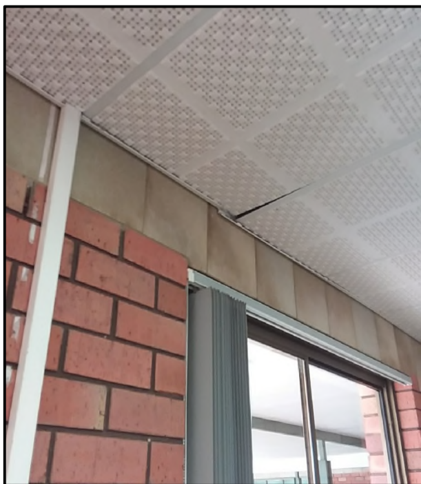
Block 1 Office – Cracks causing ceiling damage and misalignment
