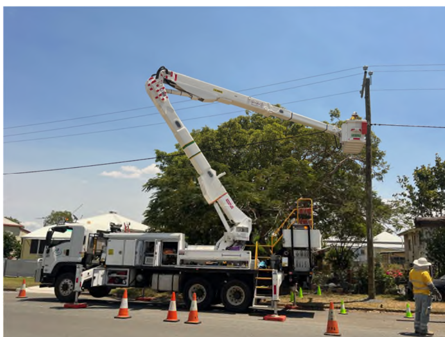
Figure 1: Example EWP in operation
