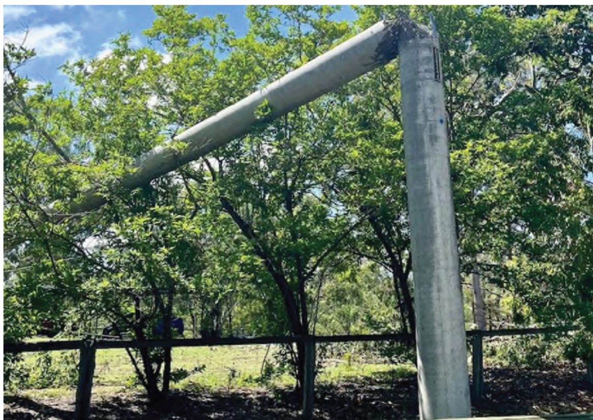
Figure 3: A concrete pole in Energex's distribution area snapped due to the force of the storms
