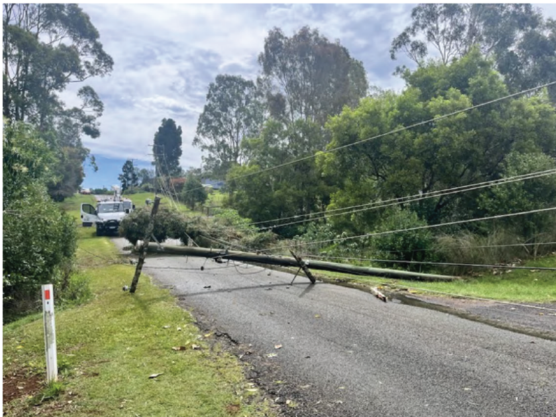
Figure 2: A fallen cross-arm in Beechmont
