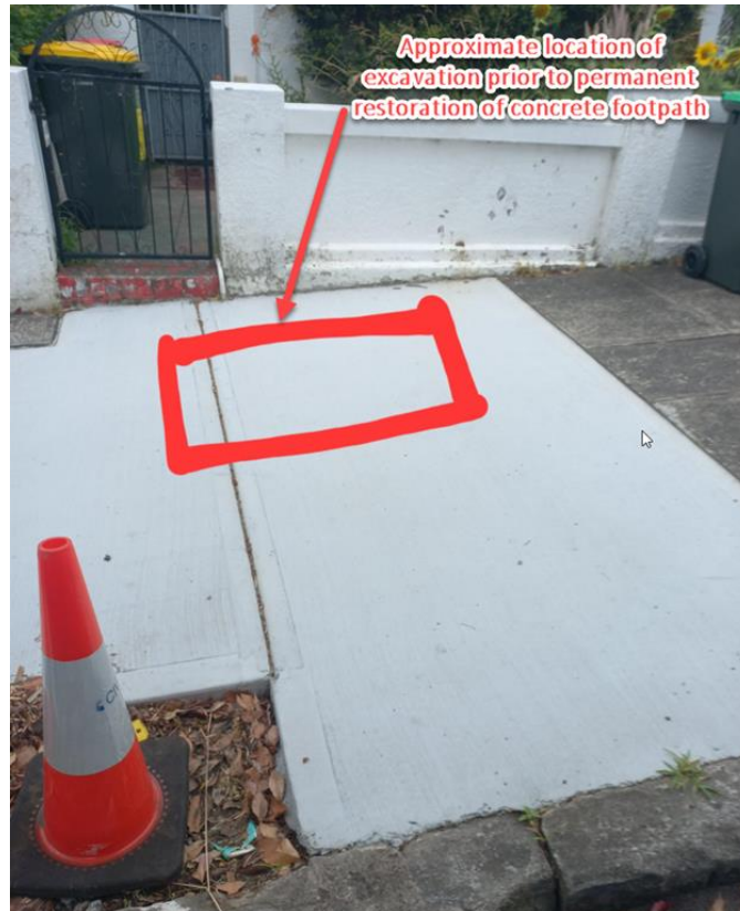
Figure 2–2: Permanent restoration undertaken by local council
