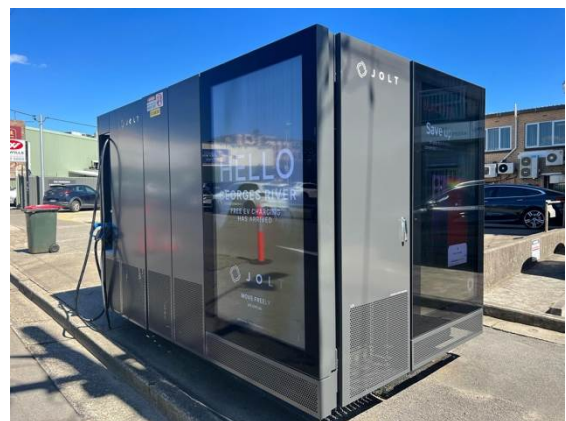
Jolt – Treacy St, Hurstville (25 kW DC with CCS2 and CHAdeMO plugs) Note only one plug can be used at any one time
