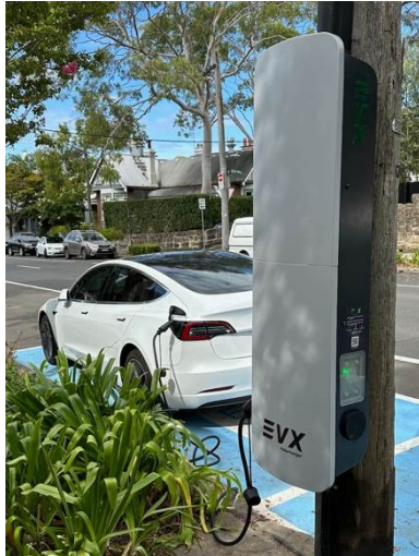
EVX – St Johns Rd, Glebe (dual 22 kW AC ports)
