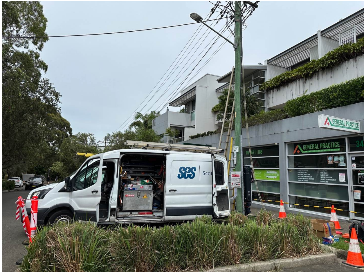
Figure 3 – EVX kerbside site being installed in Taylor St, Annandale, Inner West Council, NSW, December 2024. The site was installed and commissioned in approximately 4 hours. Kerbside chargers can be installed by independent Licenced Electrical Contractors with Level 2 Credentials.
