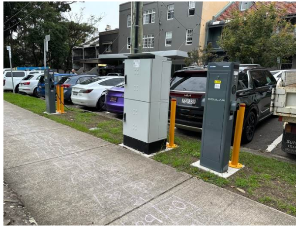
EVSE – Fowler St, Camperdown (four 22 kW AC ports across two bollards) Note the black power trunking cable on the adjacent DNSP pole
