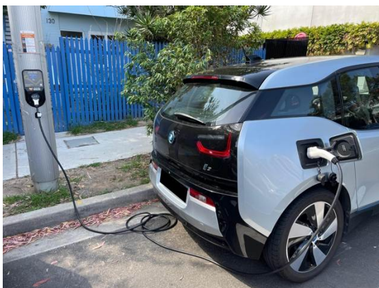
Council Smart Pole – Glenayr Ave, Bondi Beach (7 kW AC)
