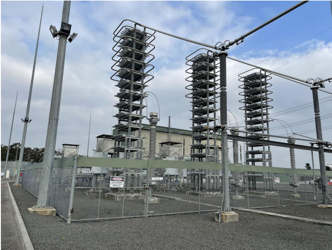
Figure 2.3 Basslink's AC filters
