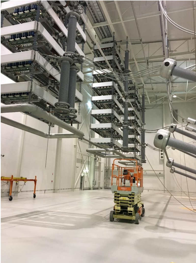
Figure 2.2 Basslink's Thyristor Valve Hall
