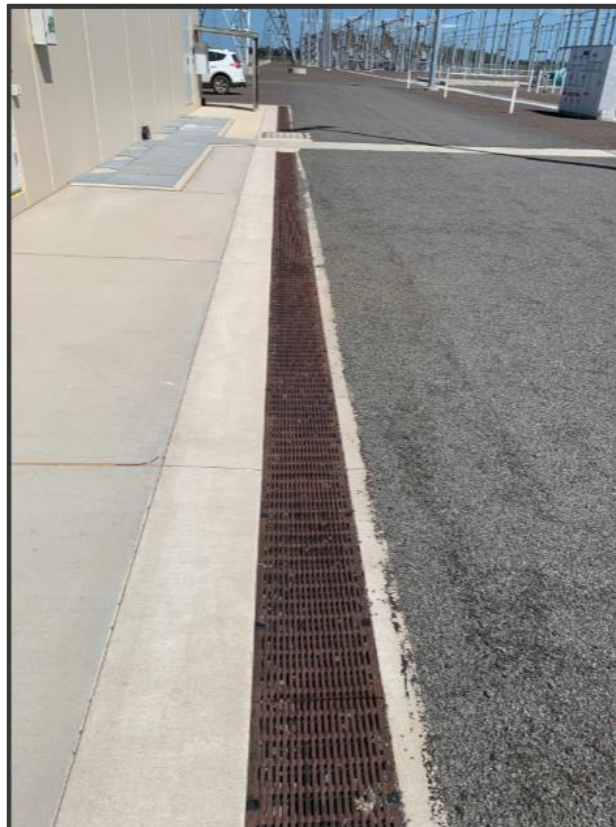
Figure 3: Typical sealed road
