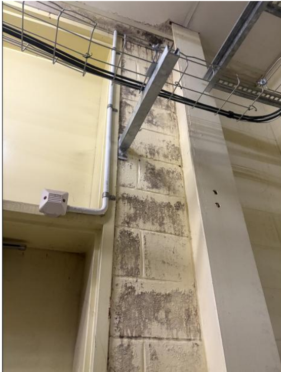
Figure 22: Poor condition of Walls and Ceilings at LY
