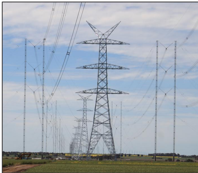
Figure 33: A 500kV tower with ERS bypasses on either side of the tower
