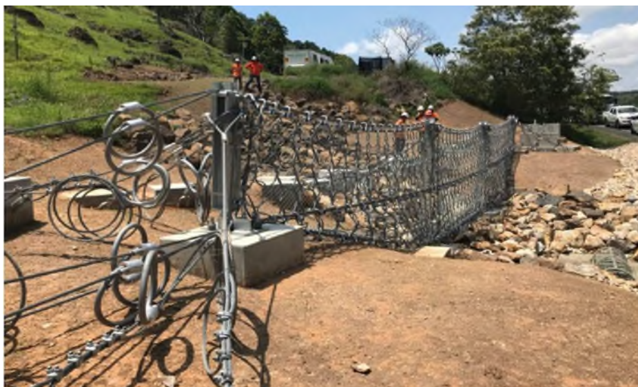
Figure 28: Example of Debris Flow Barrier Construction
