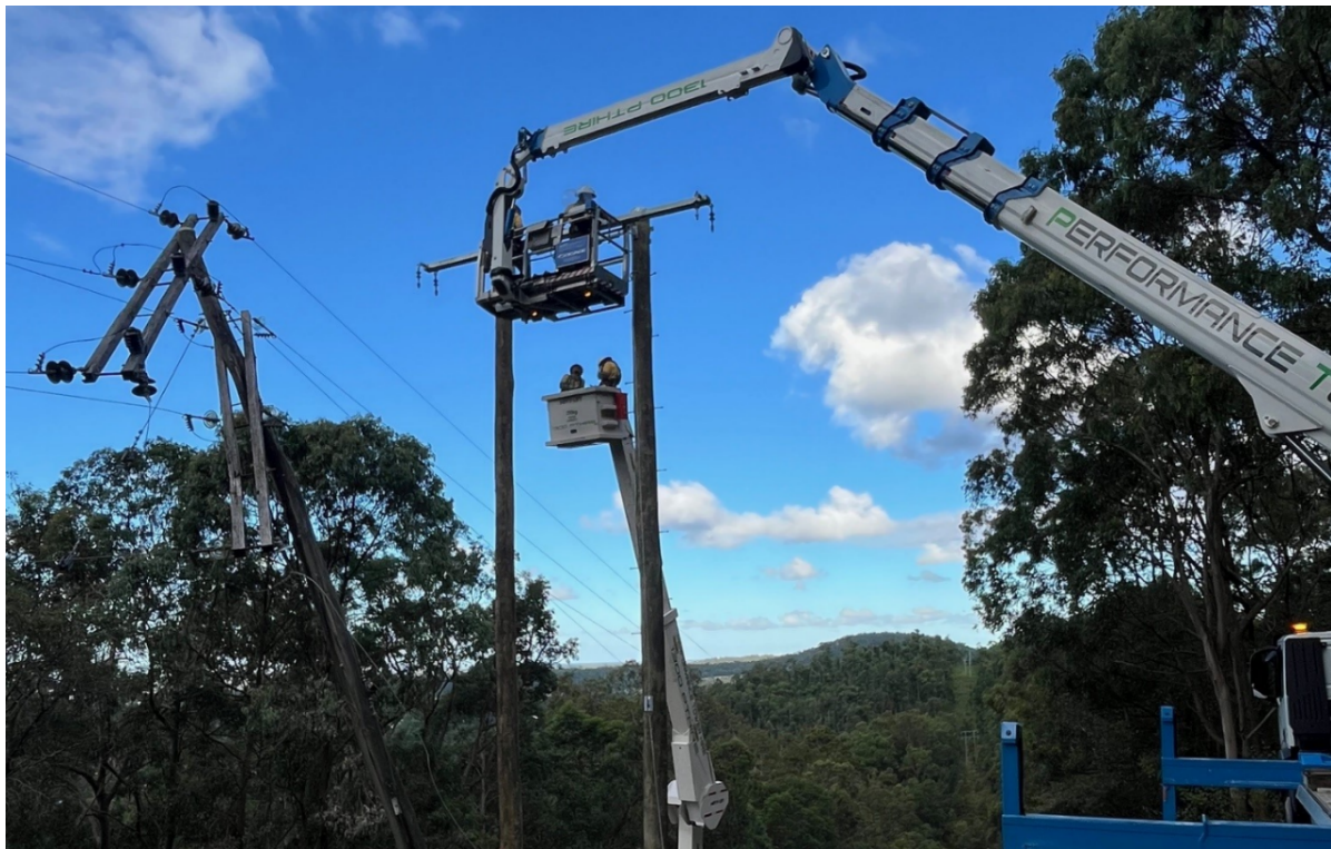
Figure 4: Broken crossarm replacement in Upper Coomera
