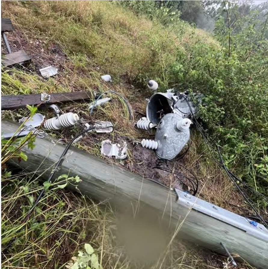
Figure 5: Pole down and smashed transformer in the Scenic Rim
