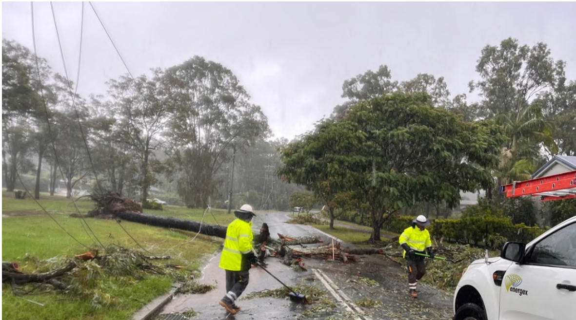
Figure 4: Broken crossarm replacement in Upper Coomera
