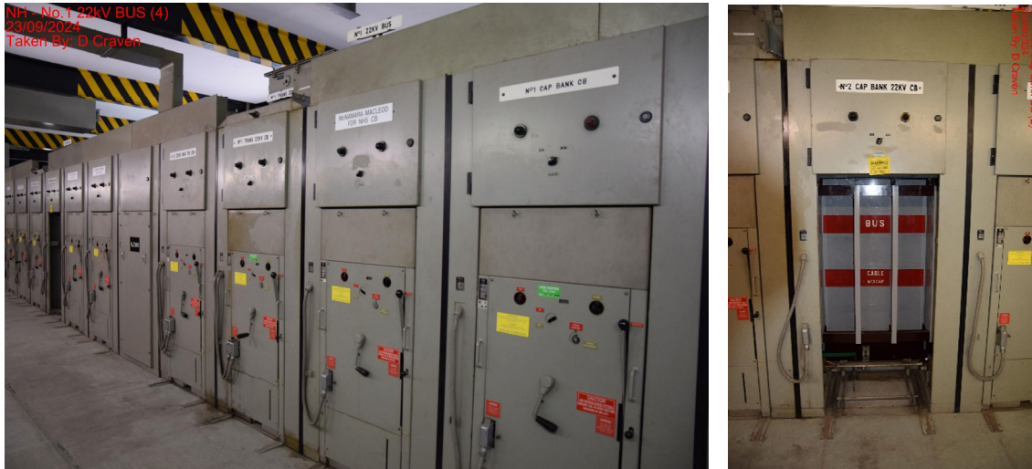
Figure 14 | NH ZSS 22kV Sprecher & Schuh Switchboard
