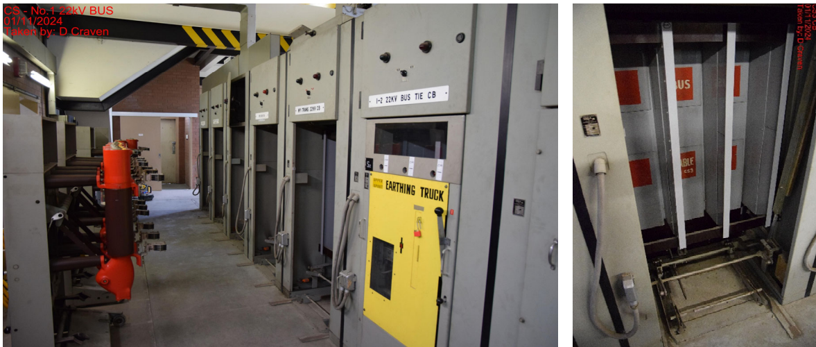
Figure 12 | CS ZSS 22kV Switchboard.
