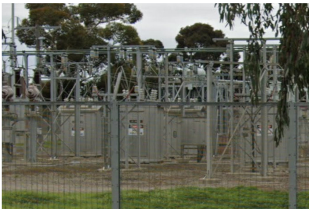
Figure 8 | CN ZSS 22kV CBs in switchyard and similar type.
