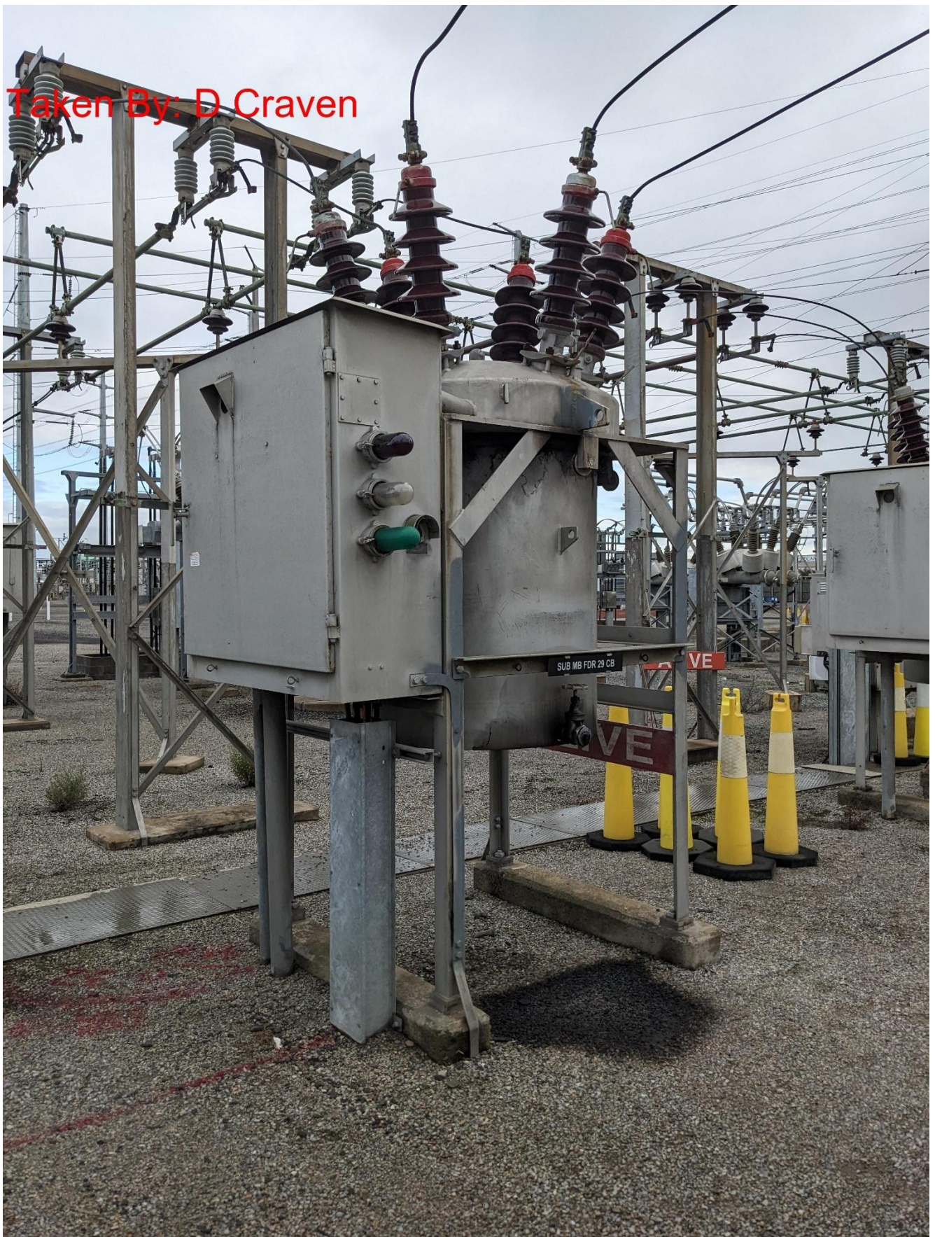
Figure 2-2: 22kV Oil Filled Circuit Breaker EMAIL/WR 345GC Type (MB29)
