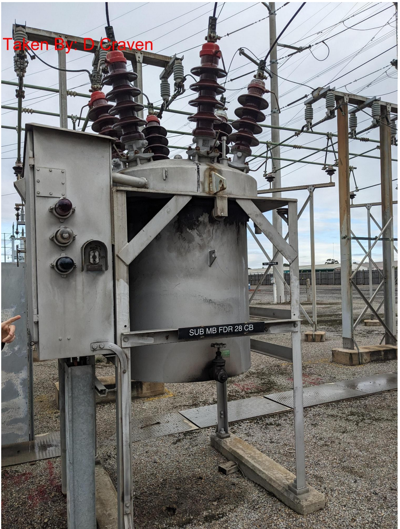
Figure 2-1: 22kV Oil Filled Circuit Breaker EMAIL/WR 345GC Type (MB28)
