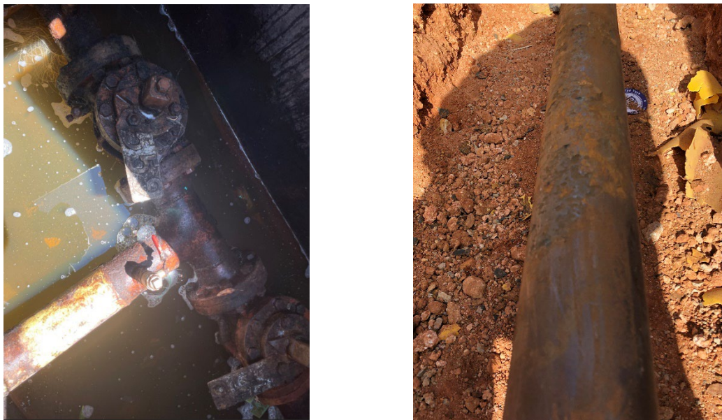
Figure 2.7: Example of corroded steel mains
