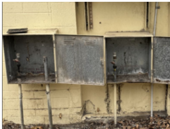
Figure 2.13: Example of redundant services where meter has been removed and live service remains
