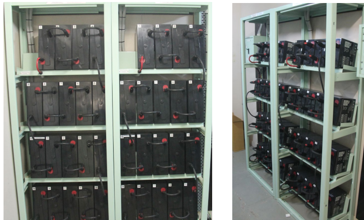
125VDC Batteries
