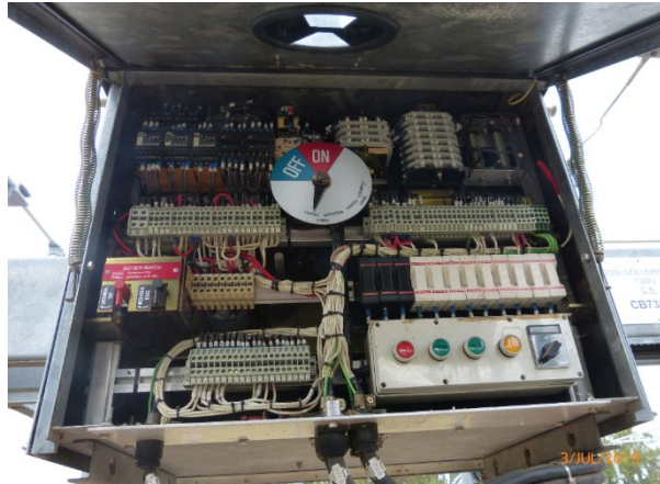
Figure 25 - CB mechanism box
