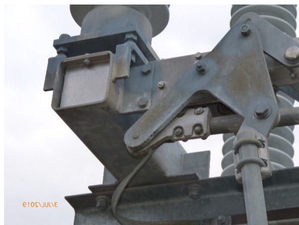
Figure 17 - Corrosion repair on bus section disconnecter.
