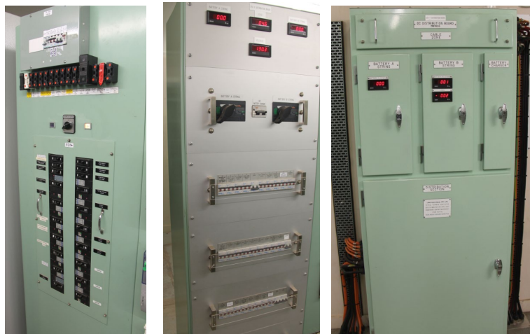
AC and DC distribution boards
