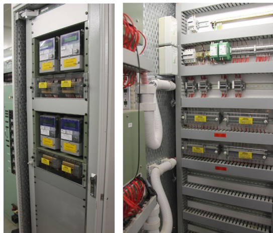
Metering panels at T013 Chinchilla
