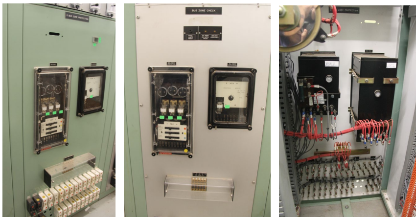
132kV Bus zone protection and control panels
