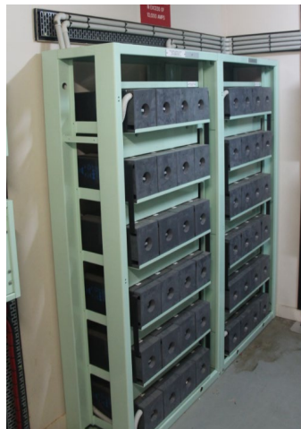
48VDC Batteries
