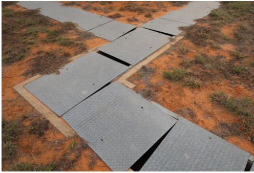
Figure 33 - Cable trenches
