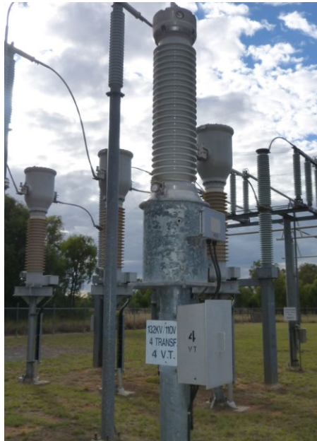
Figure 16 - A Ph. CVT and the new CT's behind.
