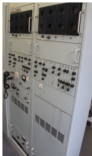
PLC equipment for Feeder 7168 and 7183
