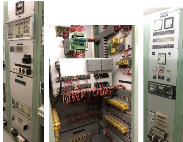
Feeder 3/1 7168 protection and Control & Auxiliary panel
