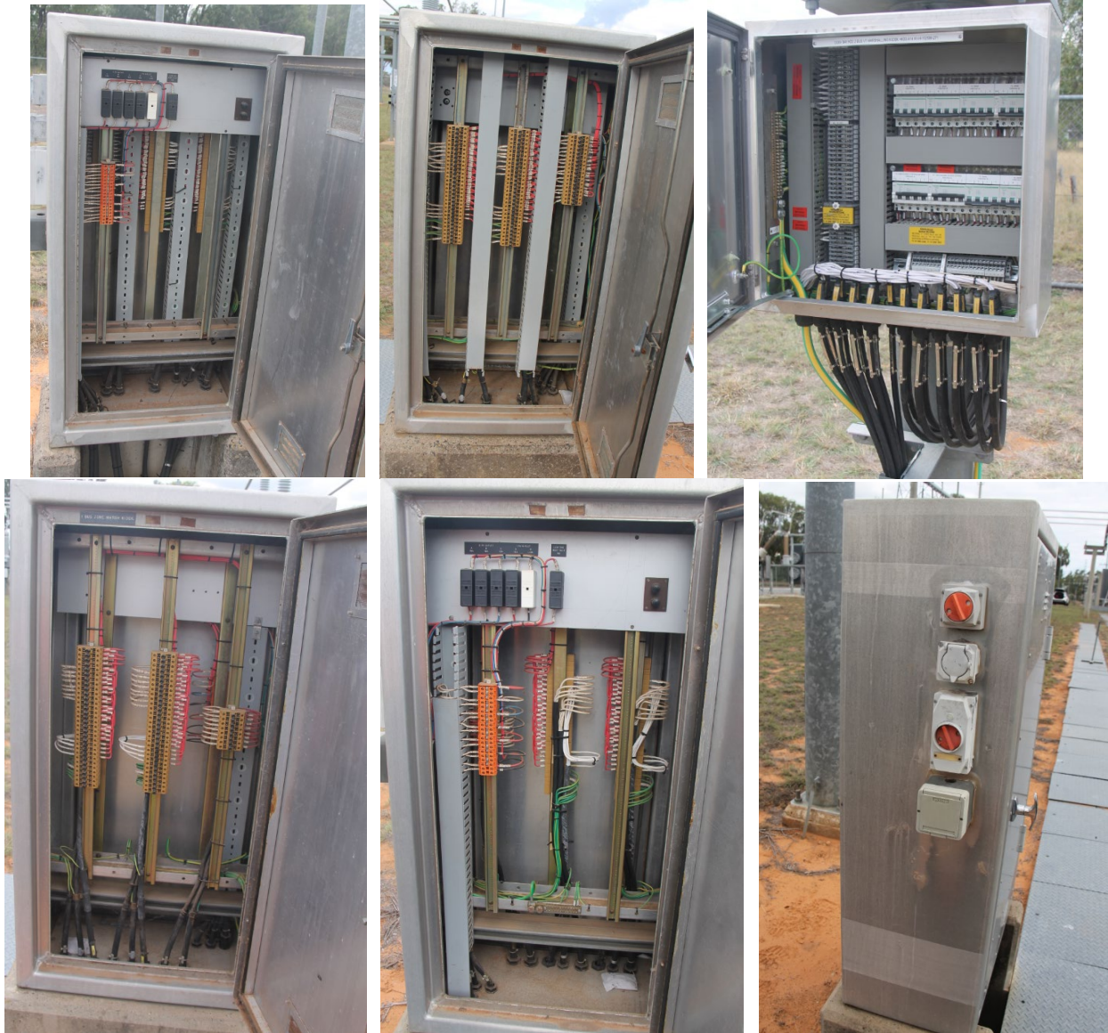
132kV bus zone marshalling kiosk and VT cubicle
