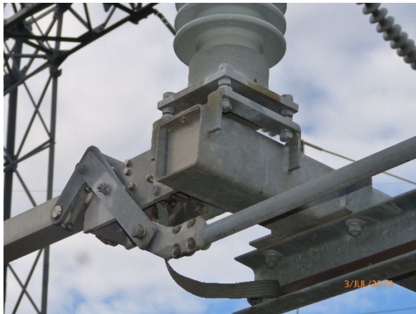
Figure 18 - Corrosion repair on bus section disconnecter.
