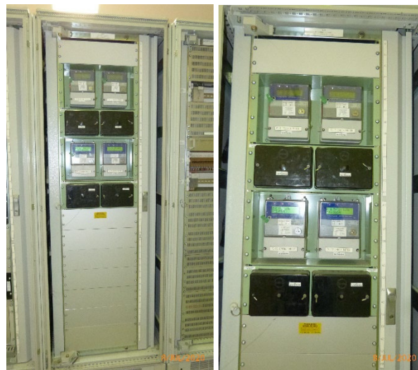
Figure 8 – Alan Sherriff Substation Typical Revenue Metering Panels
