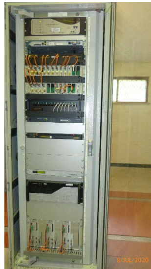
Figure 10 – Alan Sherriff Substation OpsWAN Panel
