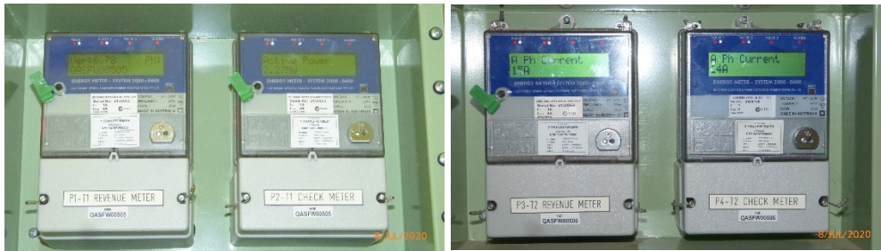
Figure 9 – Alan Sherriff substation typical revenue meters
