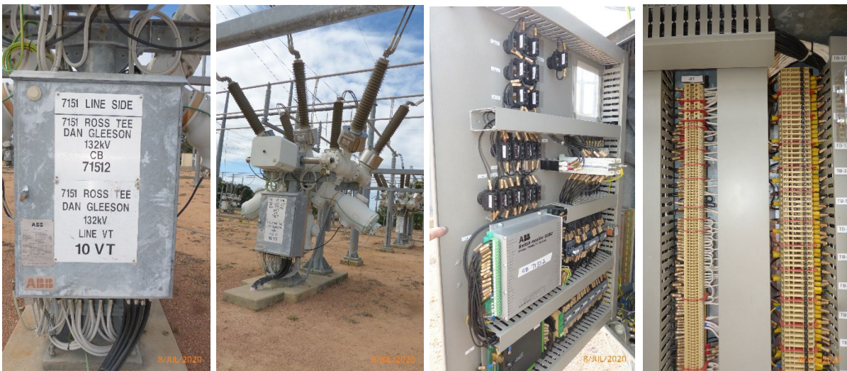
(b) 132kV Feeder 7151 – PASS-M0 Switchgear Control / Marshalling Cubicle (+D04-A10)
