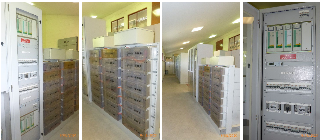
Figure 12 – Alan Sherriff Substation 125VDC Batteries and Chargers
