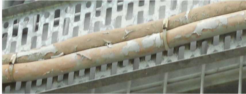
Figure 18: Year 2020 photograph of the orange PVC multicore cables showing paint flaking off the already faded outer PVC insulation.
