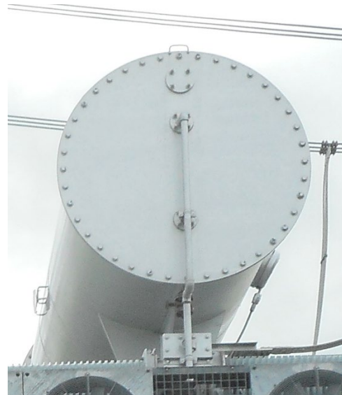
Figure 36: (LHS) Shows OLTC conservator end of the main conservator tank. (RHS) Main tank and cooler bank end of the main conservator tank. Note the single desiccant breather pipe.
