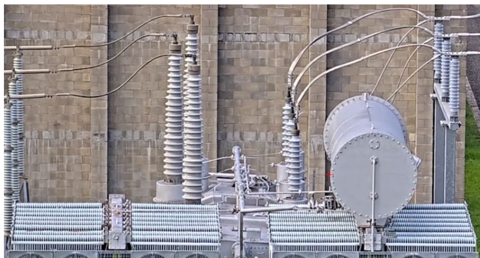
Figure 6: Transformer bushings and main oil conservator condition. Photograph taken using the substation remote monitoring camera system.
