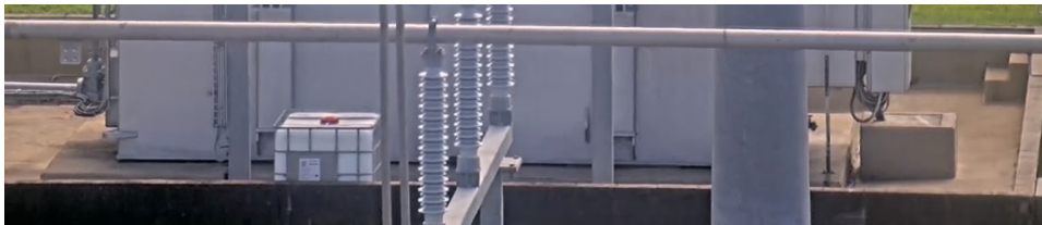
Figure 11: The concrete plinth and surrounding apron of the transformer main tank also appears to be clean / dry from oil residue. Photograph taken using the substation remote monitoring camera system.
