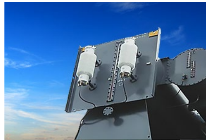
Figure 35: Operation of a Drycol breather and the typical physical mounting of such breathers on power transformer conservators.
