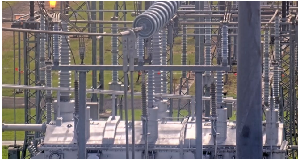
Figure 5: Transformer 110kV side showing overall condition on the lid. Photograph taken using the substation remote monitoring camera system.
