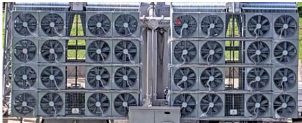
Figure 12: Transformer Cooler Bank cooling fans. Photograph taken using the substation remote monitoring camera system.
