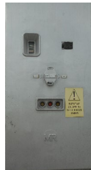
Figure 19: Reinhausen Tap Changer Control Cubicle.
