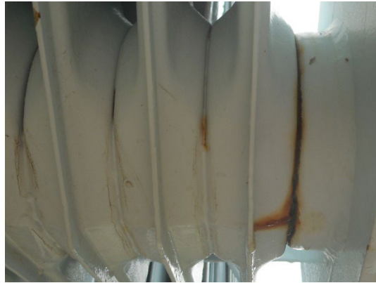
Figure 7: Transformer cooler bank radiator panel corrosion from 2020. Need to confirm if that corrosion has reappeared.
