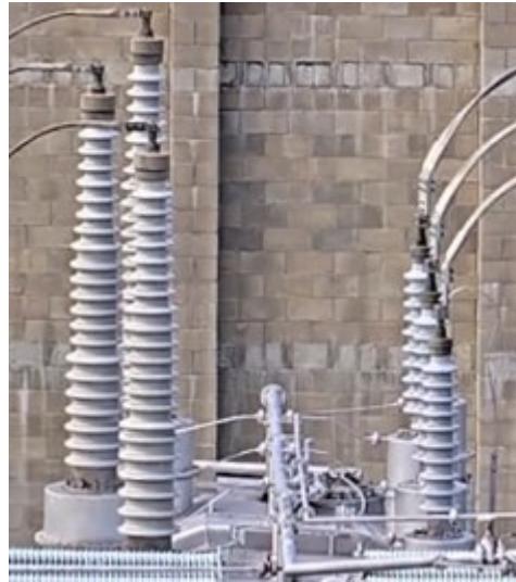
Figure 21: View of transformer HV and LV SRBP bushings. Photograph taken using the substation remote monitoring camera system.
