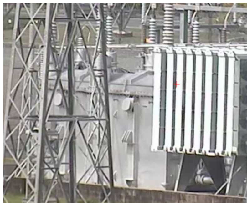
Figure 4: Transformer 275kV side showing overall condition. Photograph taken using the substation remote monitoring camera system.
