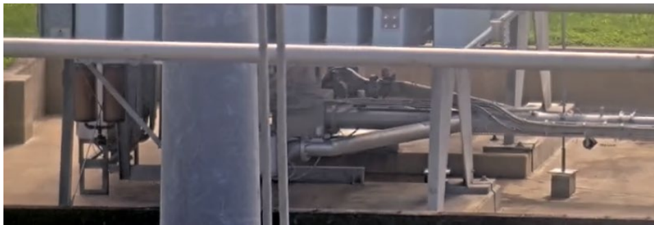
Figure 10: Side view under cooler bank does not show any significant signs of oil leaks on the concrete surfaces. Photograph taken using the substation remote monitoring camera system.
