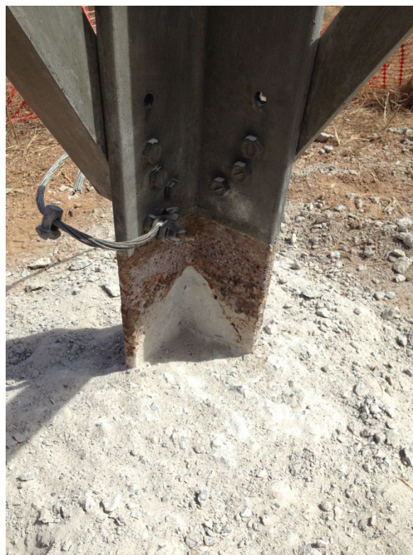
Tower leg of STR-1498 showing large cracks radiating from the tower leg and the corrosion visible once the concrete cap has been removed
