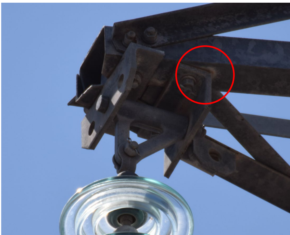
Conductor Attachment Bracket with Corrosion at Interface STR-1481
