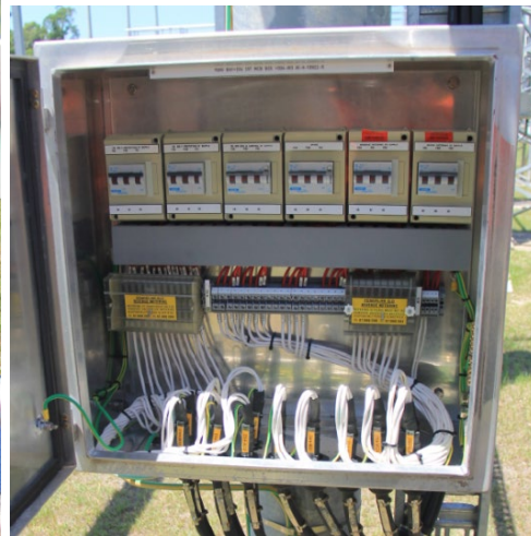
110kV Bay =D04 Feeder 794 marshalling kiosk and VT box
