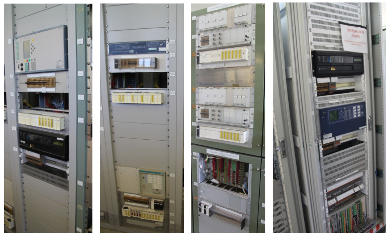
5 Transformer 275/110kV protection and control panel
