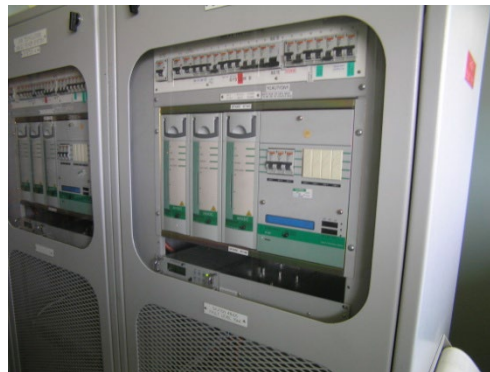
50VDC Batteries and charger
