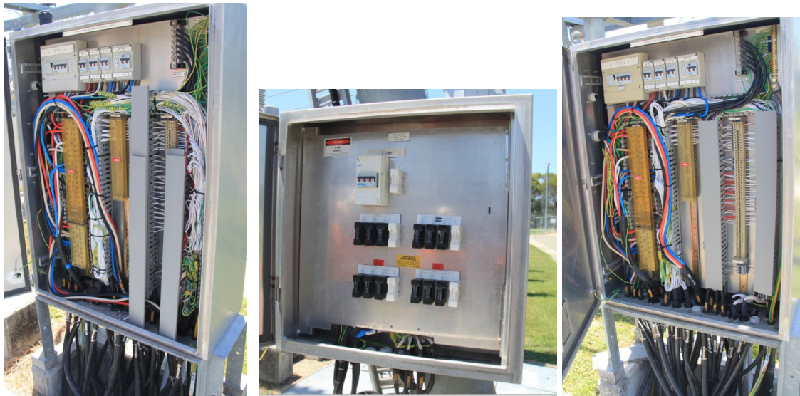
=D20 and =D721 Feeder 758 and 757 marshalling kiosks and VT box
