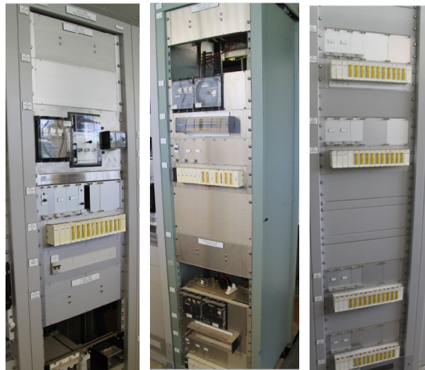
275kV 1 & 2 Bus protection and CB fail bus trip panel
