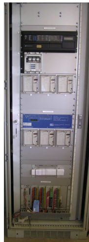
275kV 4 CAP protection and control panel
