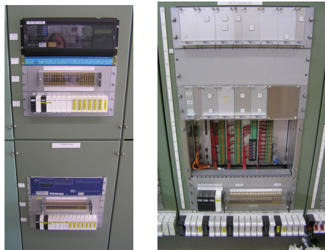
Fdr 794 protection and control panel
