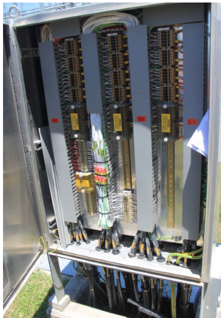
110kV Bay =D04 Feeder 794 marshalling kiosk and VT box
