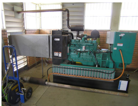
On site diesel generator
