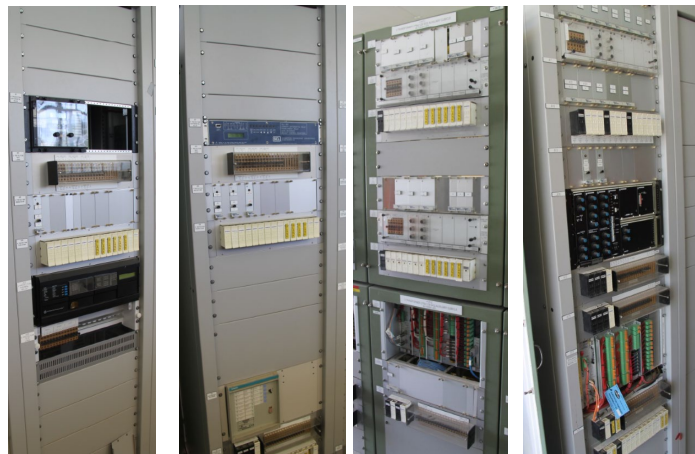
3 Transformer 275/110kV protection and control panel
