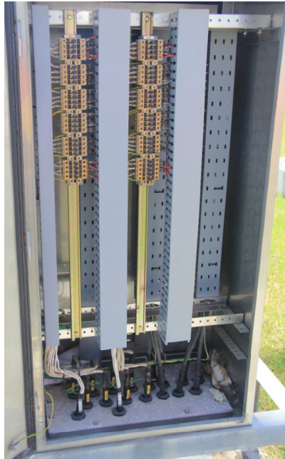
275kV bus protection marshalling kiosk
