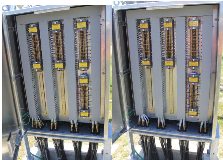
110kV Bay =D07 and =D08 Feeder 779 and 780 marshalling kiosk
