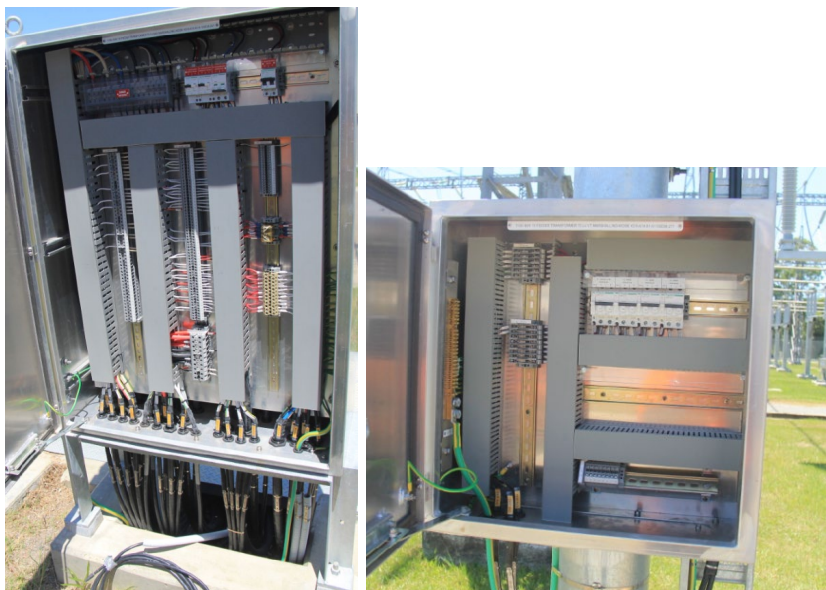
T5 LV marshalling kiosk and 110kV VT box
