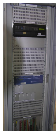
4T Protection and control panel
