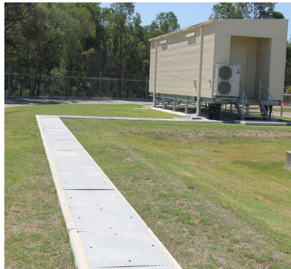
Substation trenches
