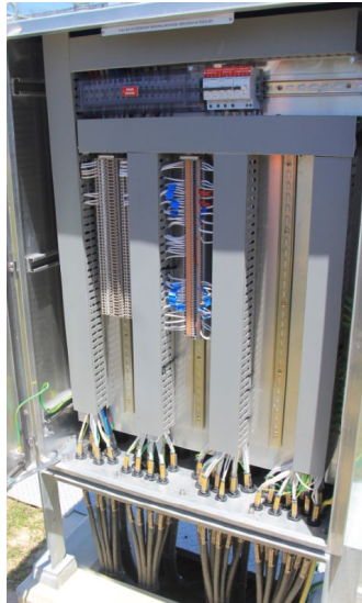
110kV Bay =D05 Feeder 706 marshalling kiosk
