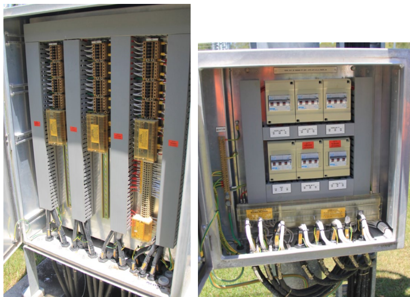
110kV Bay =D22 F839 marshalling kiosk
