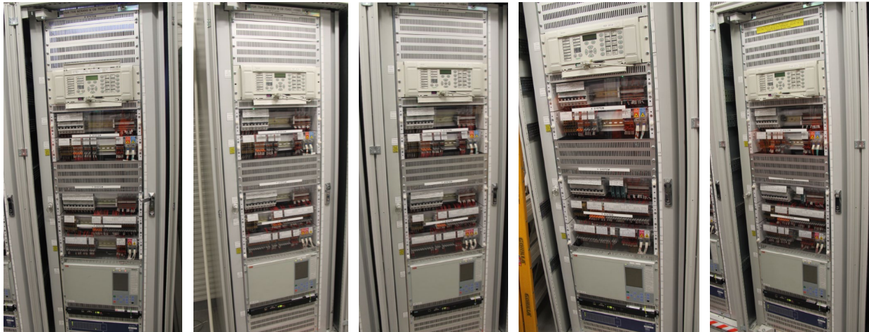
Feeder 706, 754, 755, 757 and 758 protection and control panel
