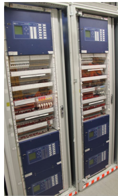
110kV Bus zone protection panels
