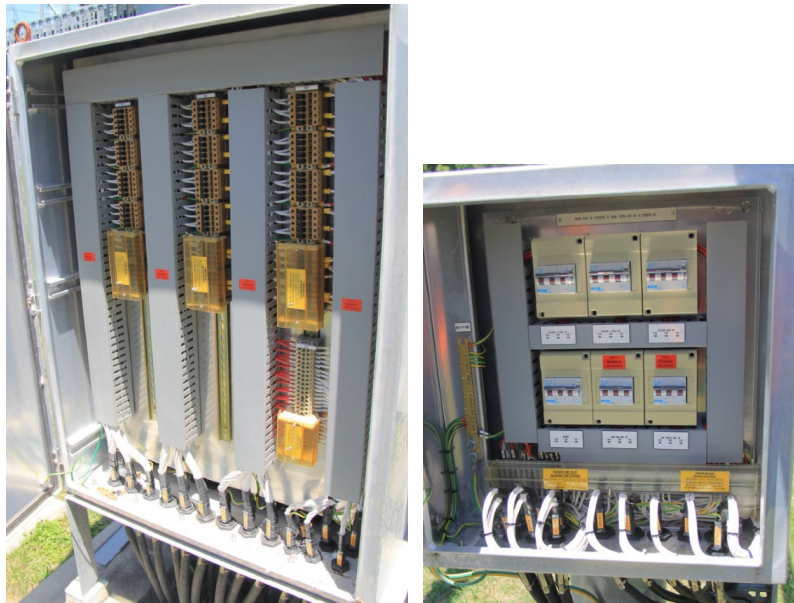
110kV Bay =D16 F838 marshalling kiosk and VT box
