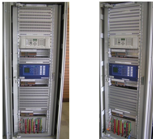
Feeder 779 and 780 protection and control panel
