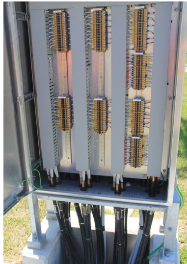
110kV bus coupler marshalling kiosk
