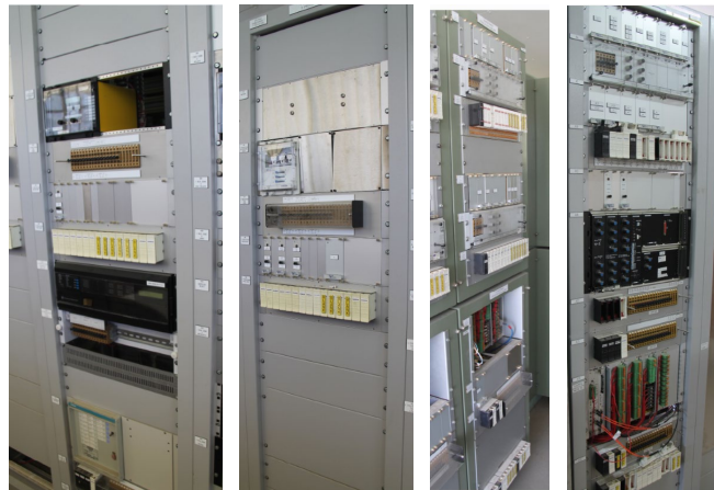
1 Transformer 275/110kV protection and control panel
