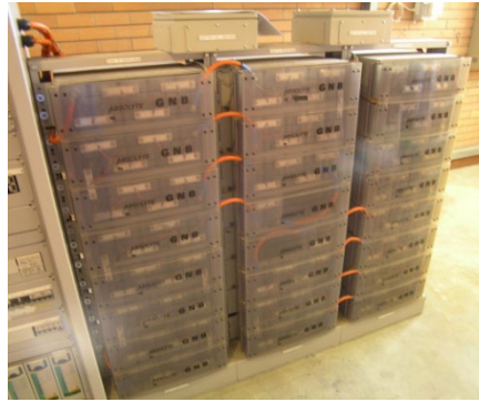
125VDC Batteries and charger
