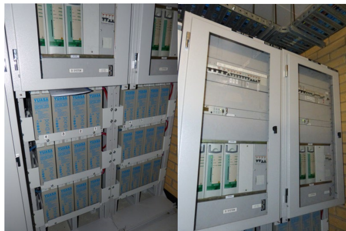
Building +T - 50VDC Batteries and Chargers Murarrie 275kV and 110kV DC Batteries and Chargers
