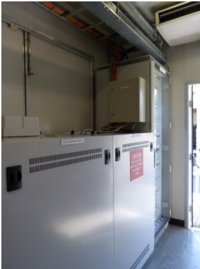
Building +A – 125VDC Batteries and Chargers
