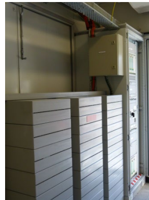
Building +5 - 125VDC Batteries and Chargers
