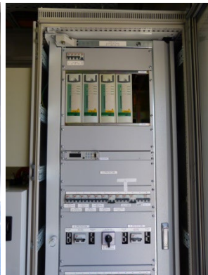
Building +C - 125VDC Batteries and Chargers
