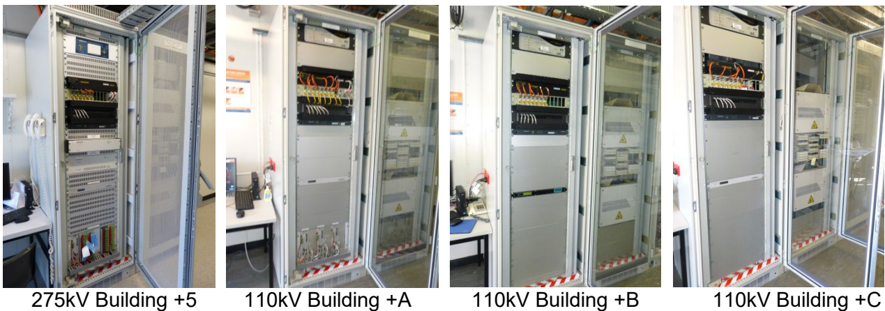
Figure 11 - Murarrie 275kV & 110kV Substation OpsWAN Systems and Equipment
