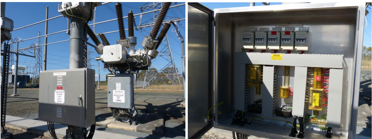
Figure 9 – Visual illustrations of a sample 110kV Conventional VT Kiosk
