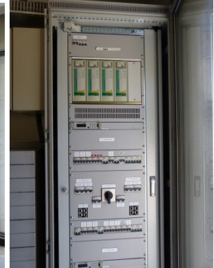
Building +5 - 125VDC Batteries and Chargers
