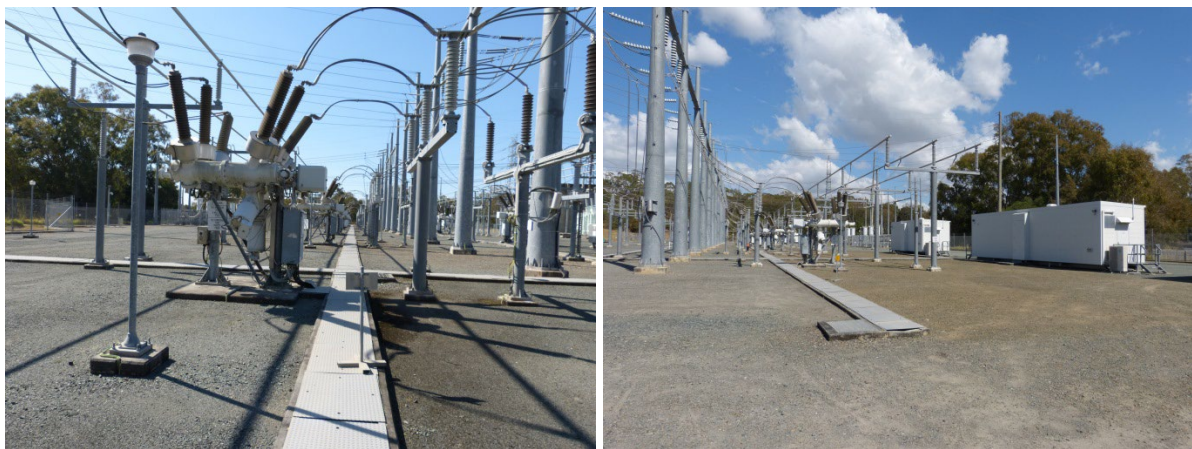
Figure 7 - Murarrie 110kV Cable Trenches
