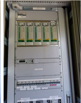
Building +B – 125VDC Batteries and Chargers
