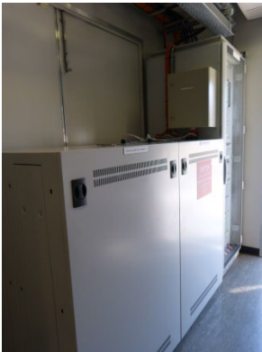
Building +C - 125VDC Batteries and Chargers
