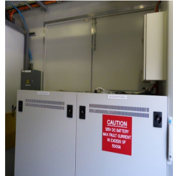
Building +B – 125VDC Batteries and Chargers
