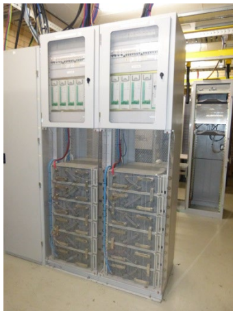
Building +T - 50VDC Batteries and Chargers
