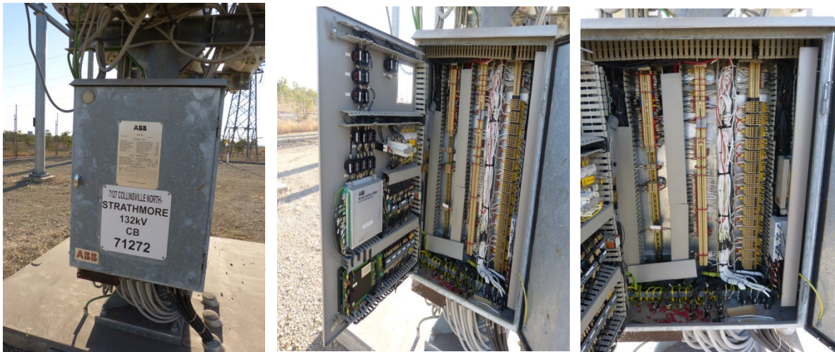
Figure 10 – Visual illustrations of a sample 132kV PASS-M0 Control Cubicle
