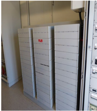
Building +5 – 125VDC Batteries and Chargers
