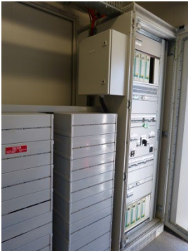
Building +5 – 125VDC Batteries and Chargers
