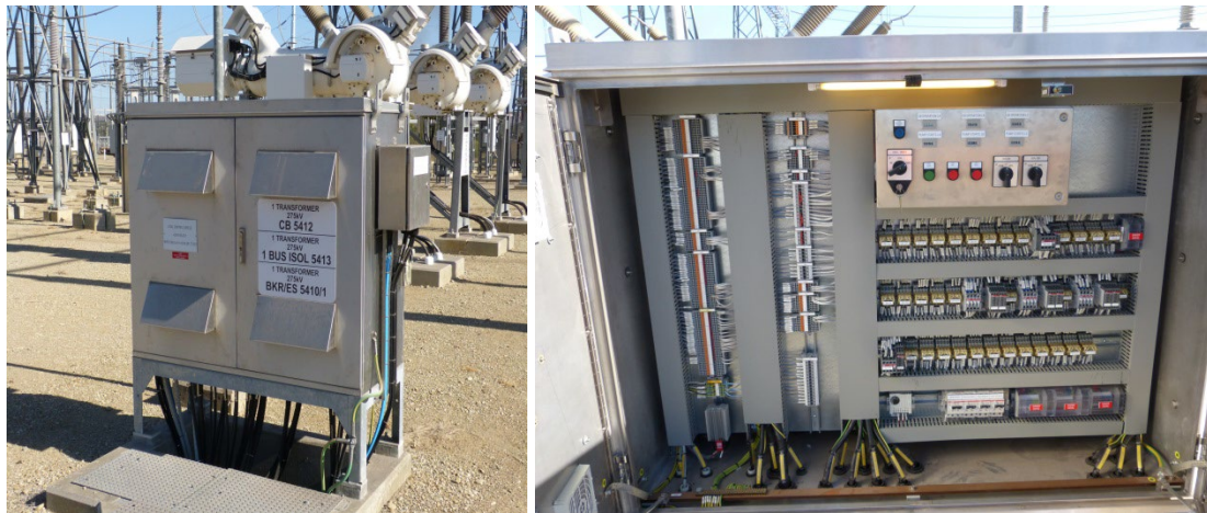
Figure 11 – Visual illustrations of a sample 275kV PASS-M0 Local Control Cubicle
