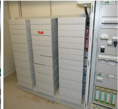
Building +6 – 125VDC Batteries and Chargers
