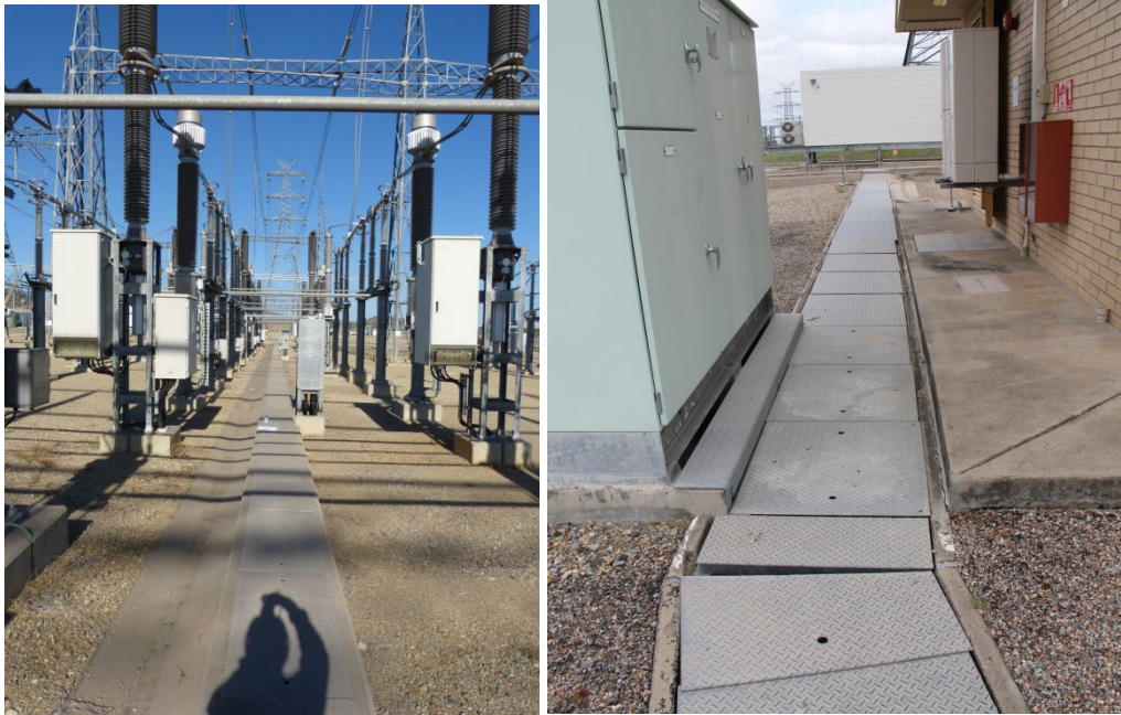
Figure 9 - Strathmore 275 kV Cable Trenches
