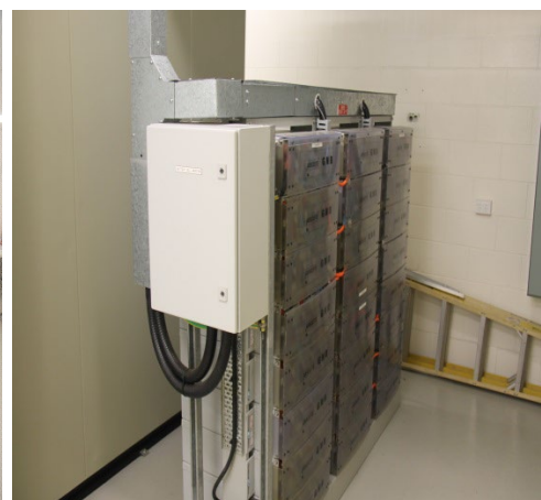
Building +4 (SVC) - 125VDC Batteries and Chargers
