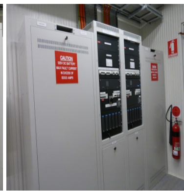
Building +9 - 125VDC Batteries and Chargers
