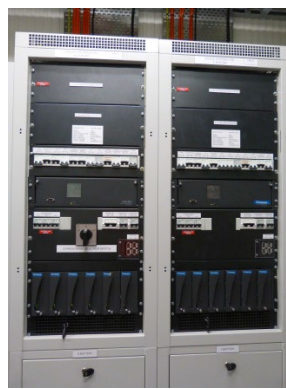
Building +9 - 125VDC Batteries and Chargers
