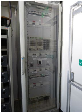
Building +E - 125VDC Batteries and Chargers
