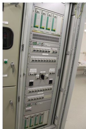
Building +4 (SVC) - 125VDC Batteries and Chargers
