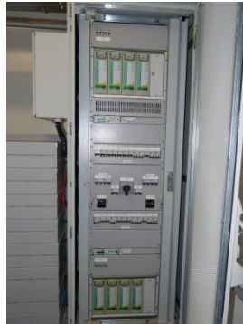
Building +6 – 125VDC Batteries and Chargers
