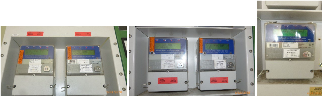
Figure 9 – Garbutt substation typical revenue meters
