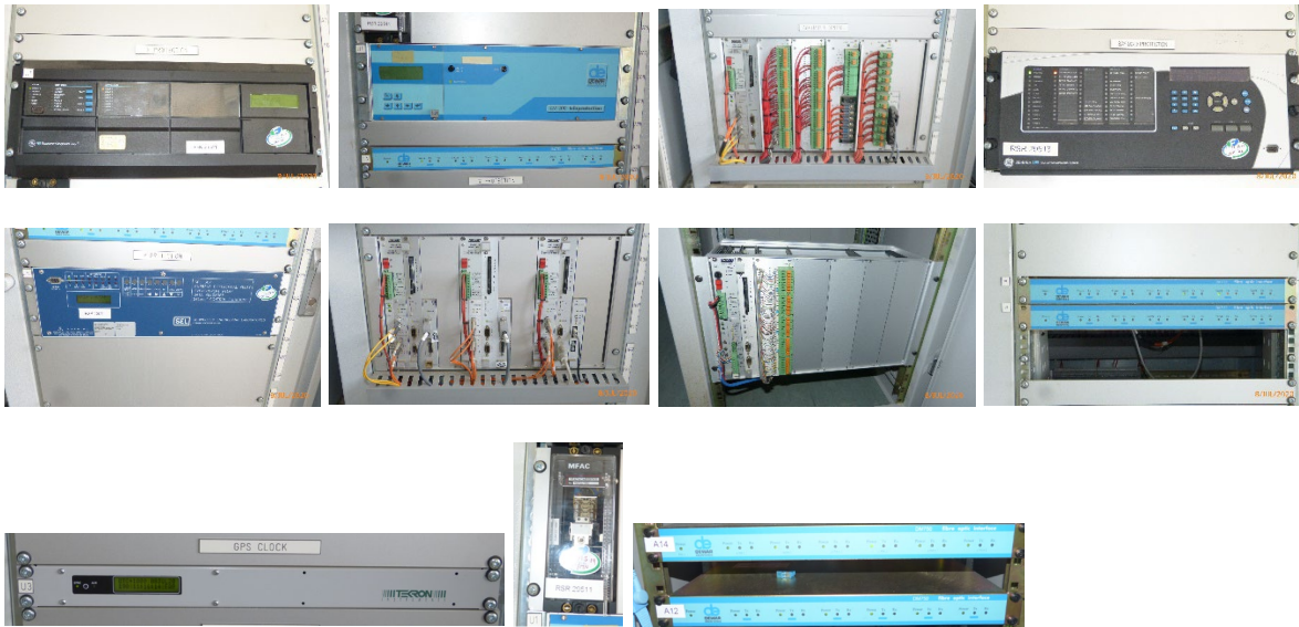
Figure 7 – Garbutt Substation Typical Indoor 132kV Secondary System Equipment
