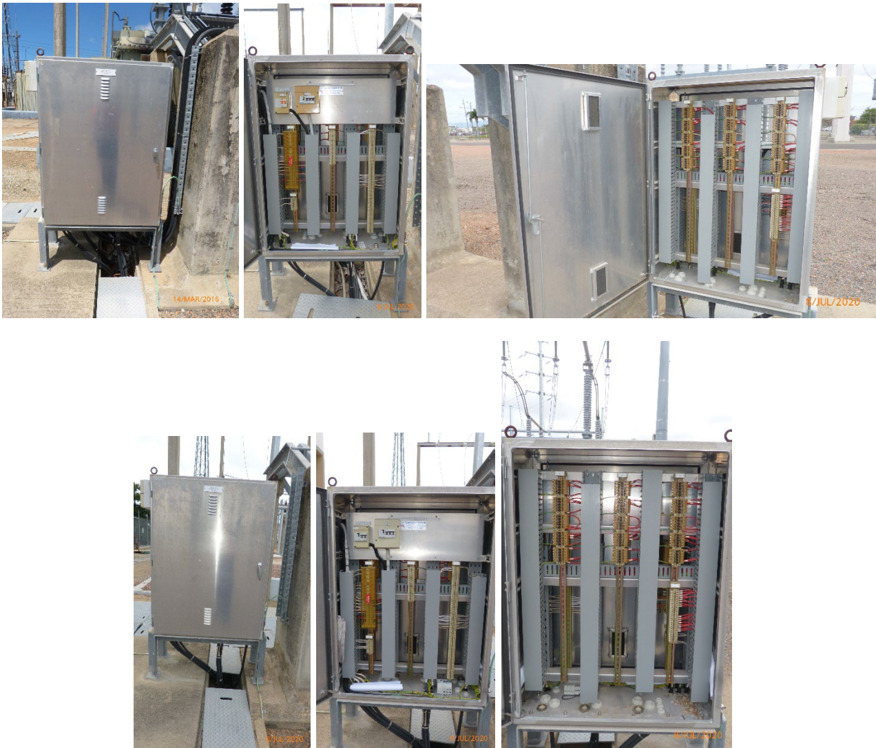
Figure 4 –132kV Outdoor Marshalling Cubicle Bay +D01-A10 (top) and +D03-A10 (bottom),
