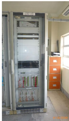
Figure 10 – 132kV Building OpsWAN and SCADA equipment
