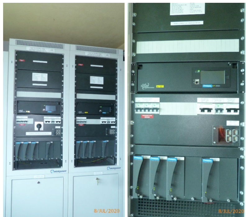
Figure 12 - 132kV Building +P – Chargers, Monitors, DC Distribution 2009, Batteries 2019
