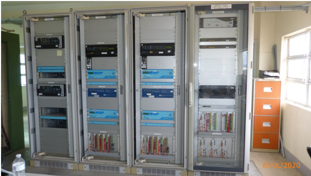
Figure 6 – 132kV Indoor Secondary Systems Cubicles
