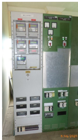
Figure 8 – Garbutt substation revenue metering panel
