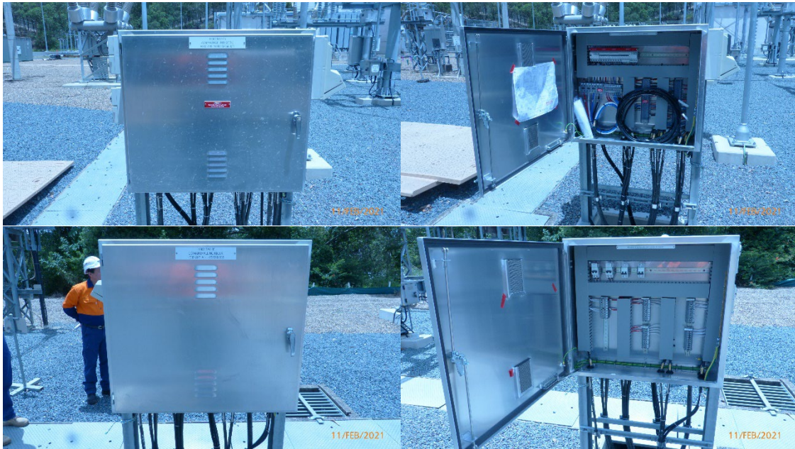
Figure 18. Bay 5 AC and DC Marshalling Kiosks +D05-A91, +D05-A92
