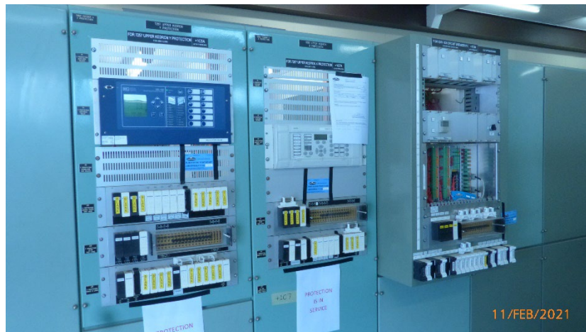
Figure 30. Feeder 7257 Control and Protection Panel [2021].
