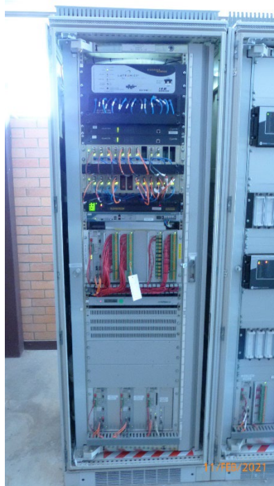
Figure 36. Ashgrove West Substation OpsWAN Panel
