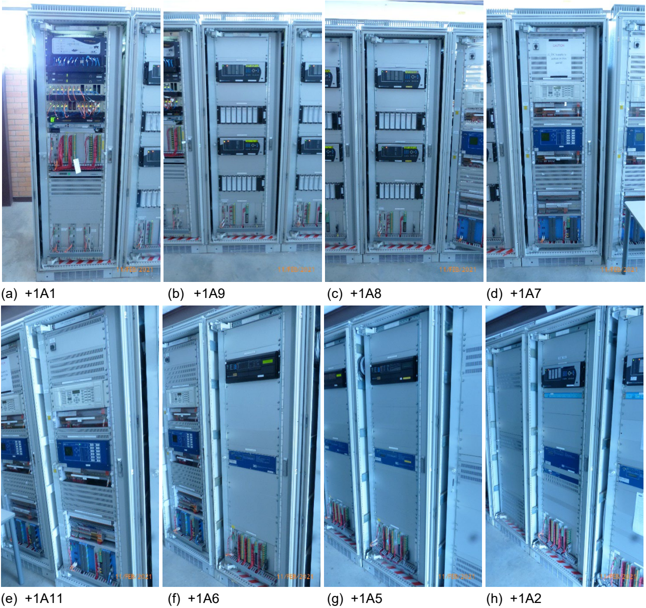
Figure 31. Typical Indoor Control and Protection Panels at Ashgrove West.
