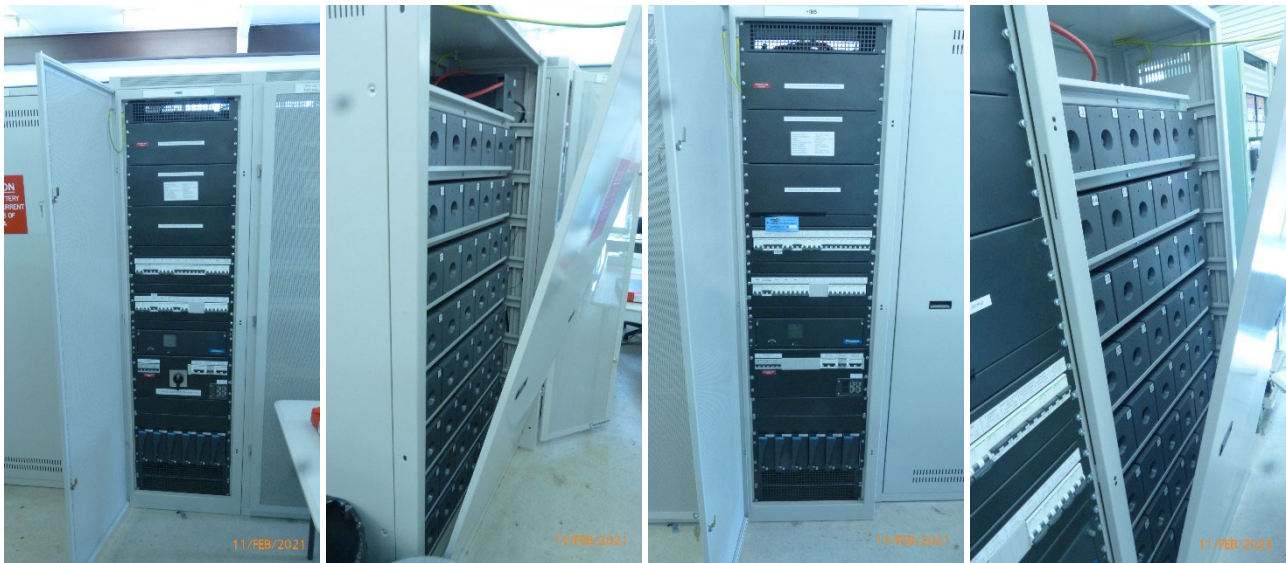
Figure 38. Ashgrove West Substation 125VDC Batteries and Chargers.
