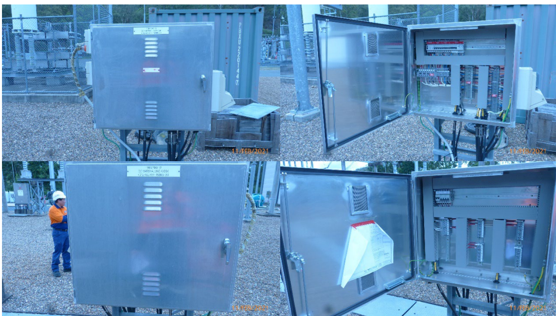
Figure 22. Bay 12 AC and DC Marshalling Kiosks +D12-A91, +D12-A92
