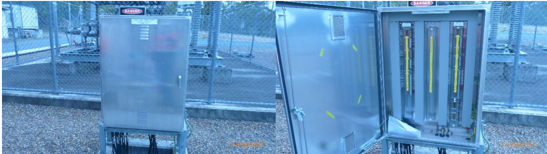
Figure 12. Transformer Interface Kiosk +U2-A10
