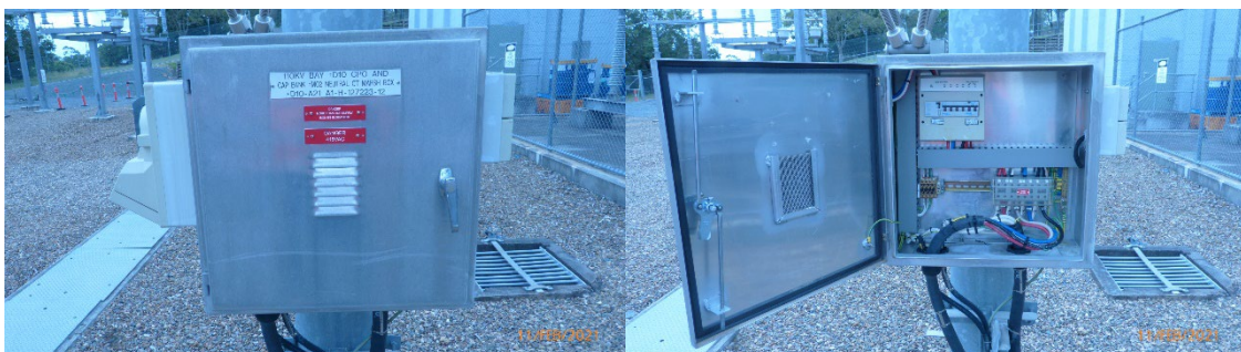
Figure 23. Bay 10 2Capacitor Marshalling Kiosk +D10-A21
