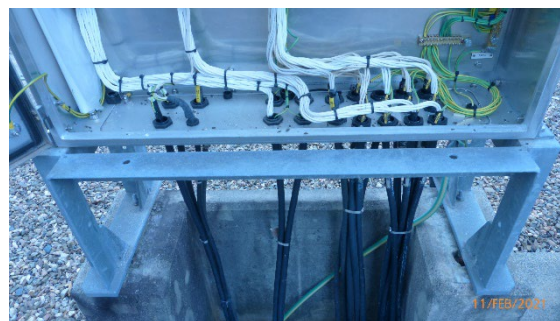
Figure 27. Cabling in 2 Bus VT Marshalling Kiosk +KD2-A5
