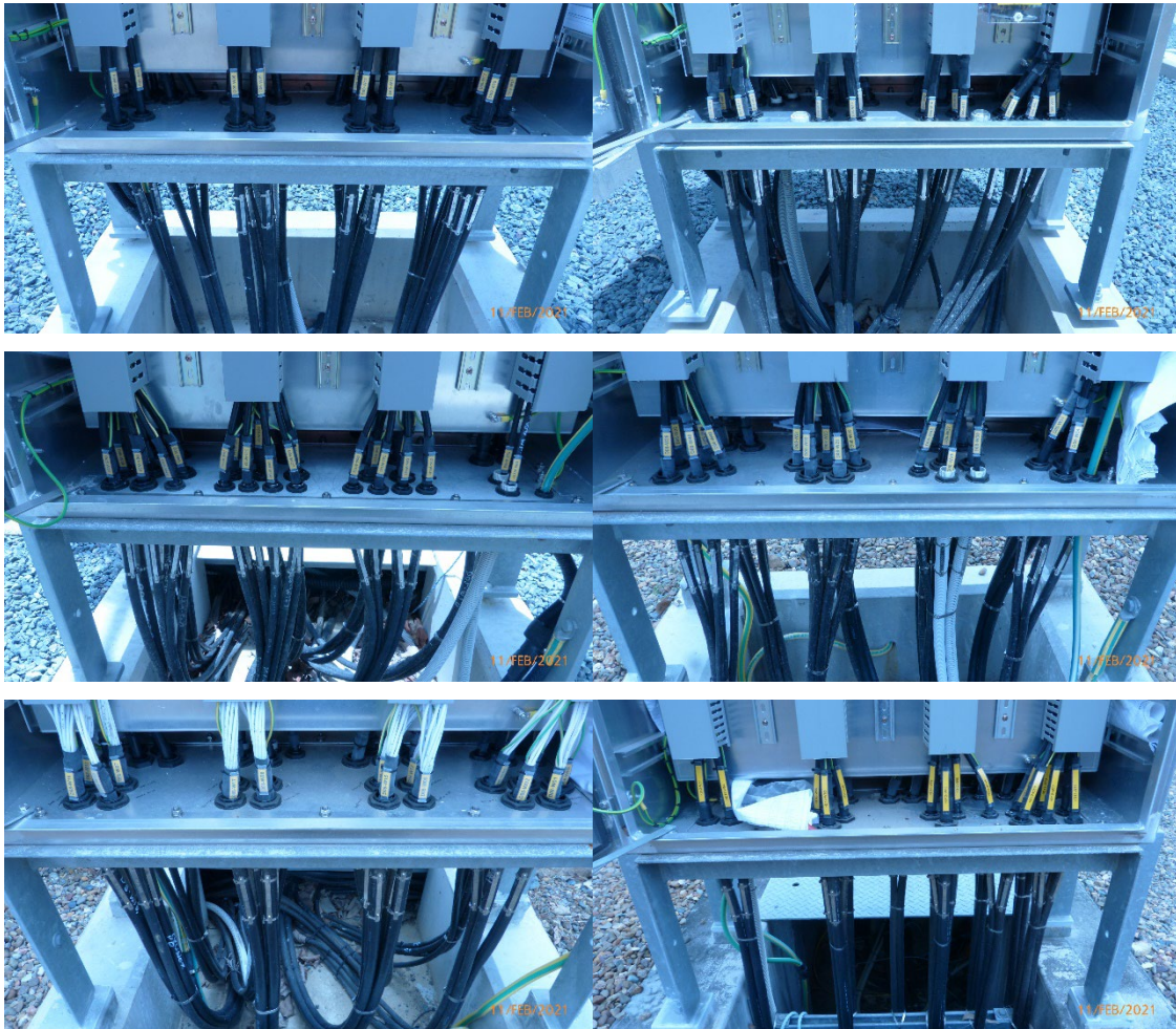
Figure 28. Cabling in Marshalling Kiosks replaced under CP.02355.
