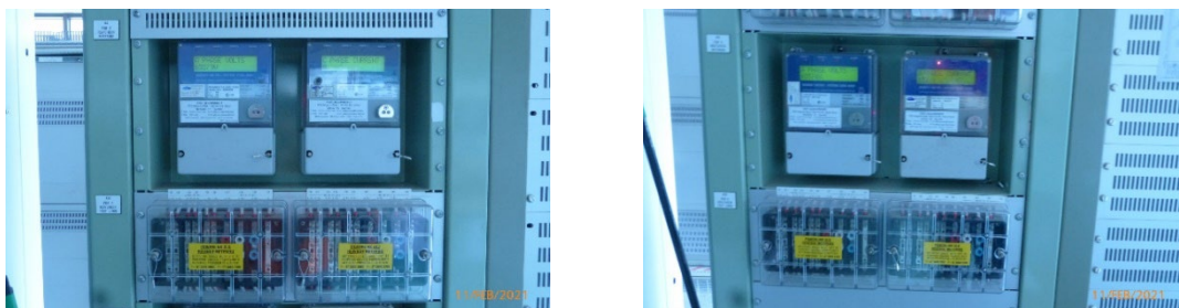
Figure 35. Ashgrove West Substation Revenue Meters
