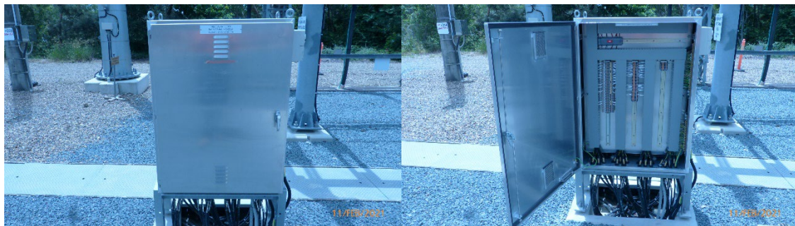
Figure 16. Bay 6 Marshalling Kiosk +D06-A10
