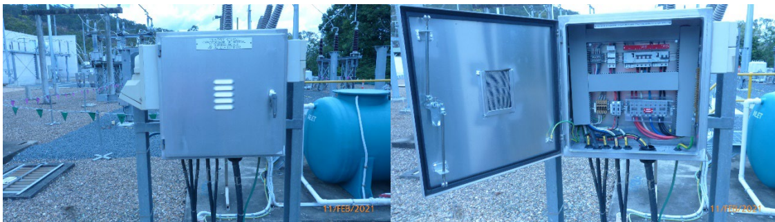
Figure 25. Bay 1 4Capacitor Marshalling Kiosk +D01-A21
