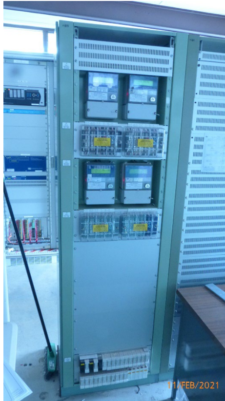
Figure 34. Ashgrove West Substation Revenue Meter Panel.
