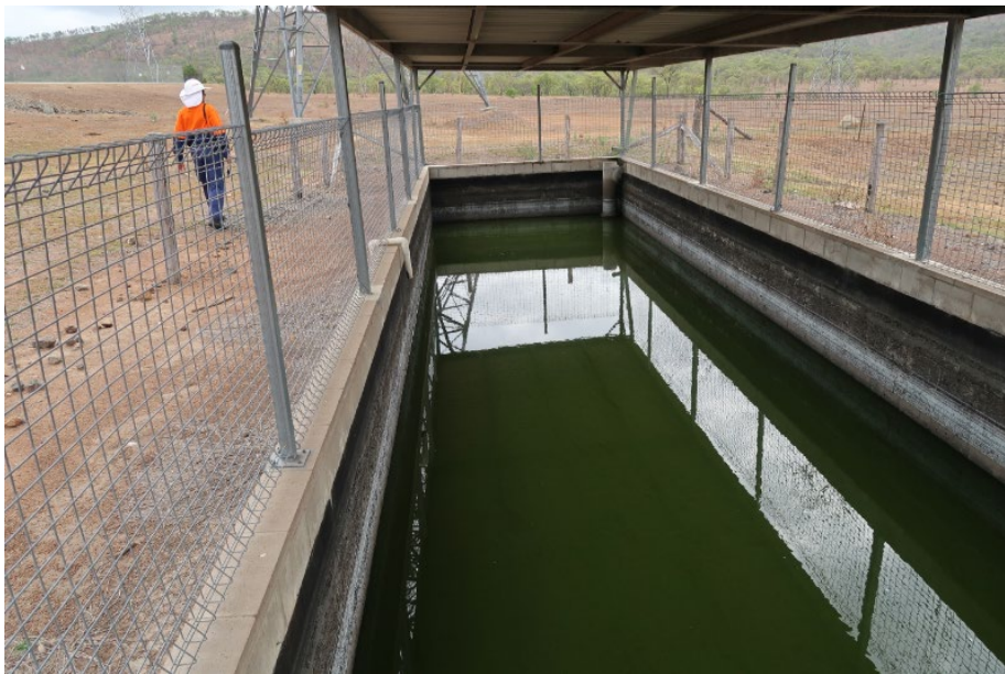
Figure 10: Oil Separation Tank
