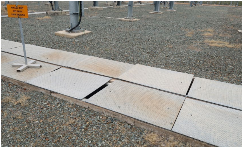
Figure 9 – Cable trenches
