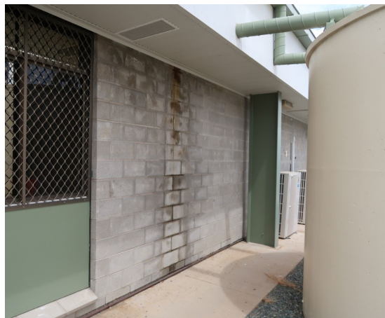
Figure 5: Building +1 Water Leak
