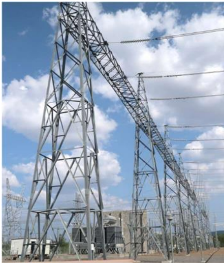
Figure 21: 275kV Strain Structure
