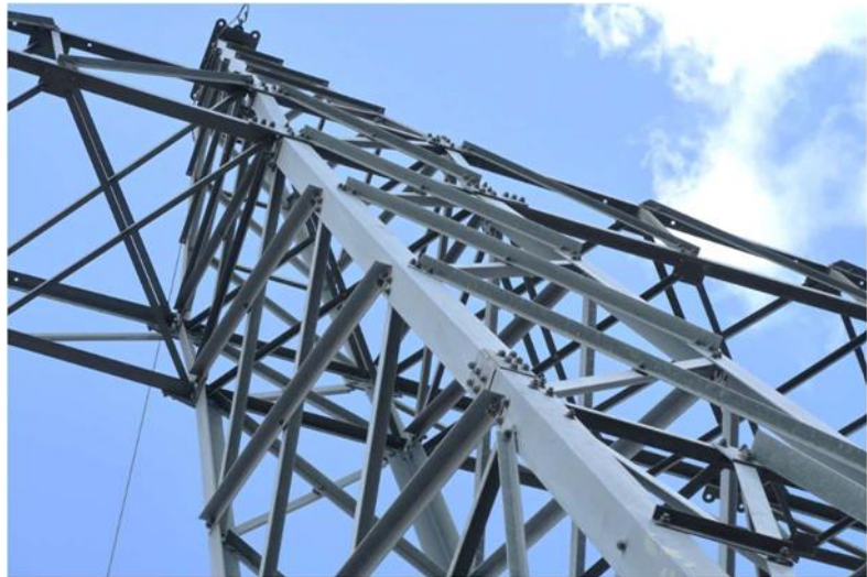
Figure 22: 275kV Structure Main Leg
