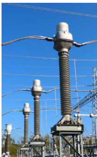
Figure 9 – Circuit Breaker
