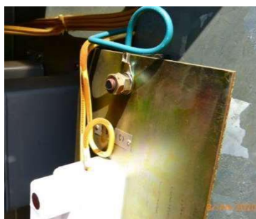
Figure 15 - Wiring UV damages
