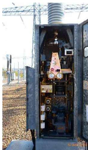
Figure 10 – Circuit breaker cubicle
