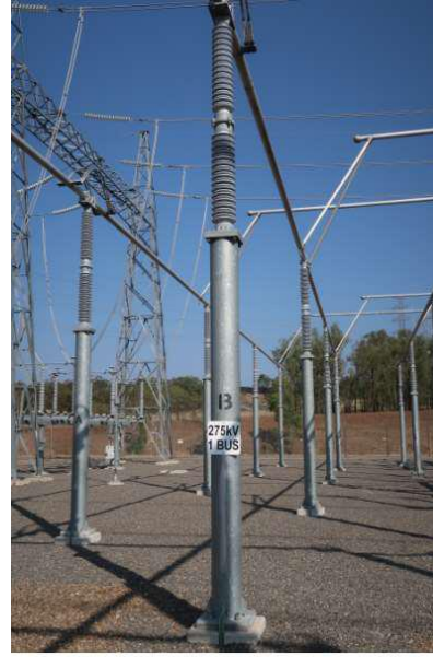
Figure 18: 275kV Tubular Bus Support Structure
