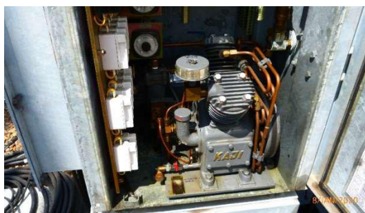
Figure 14 - CB Mech box oil leak
