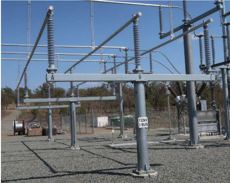
Figure 17: 132kV Bus Support Structure
