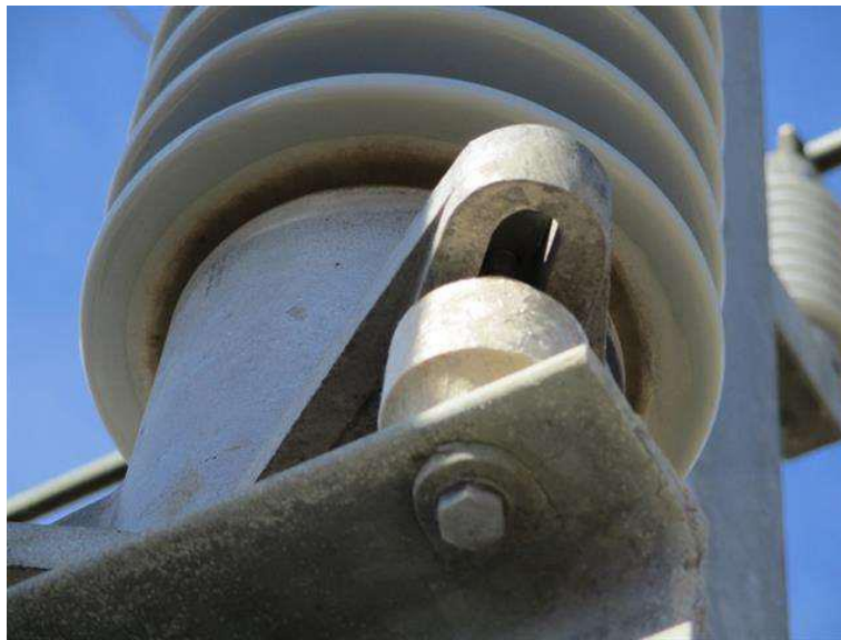
Figure 16 - Deteriorated coating on associated insulator
