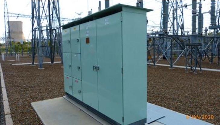
Figure 26: AC changeover board
