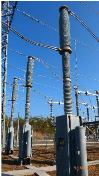
Figure 13 - Circuit Breaker
