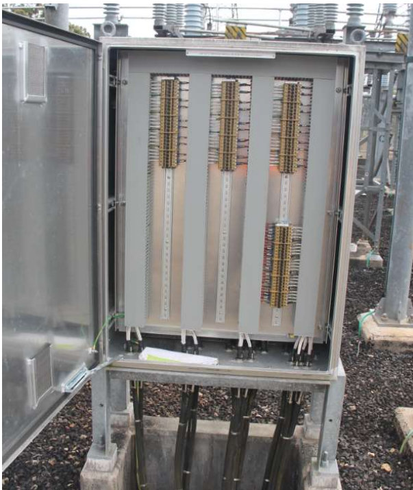
132kV Bay =D07 Feeder 7166 bay marshalling kiosk
