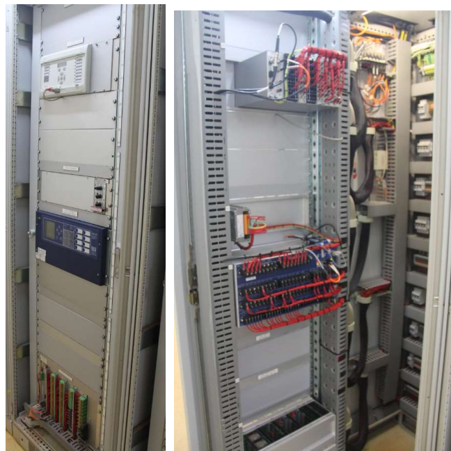
Feeder 858 protection and control panel
