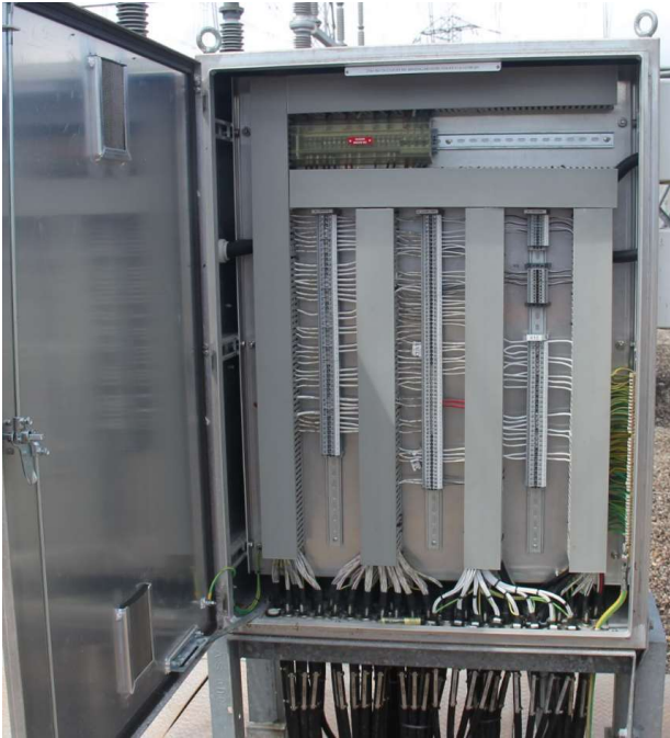
275kV Bay 4 coupler bay marshalling kiosk
