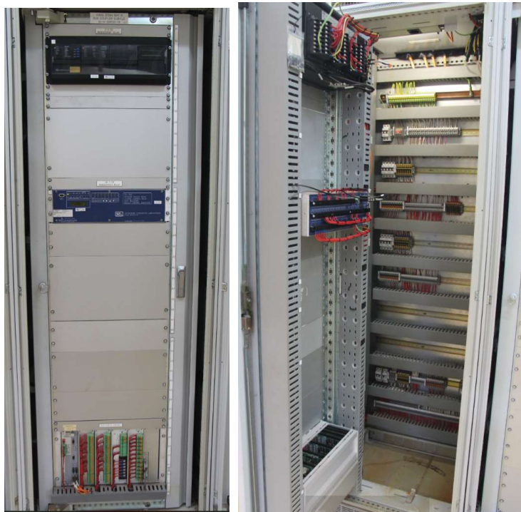
Coupler 506 protection/control panel
