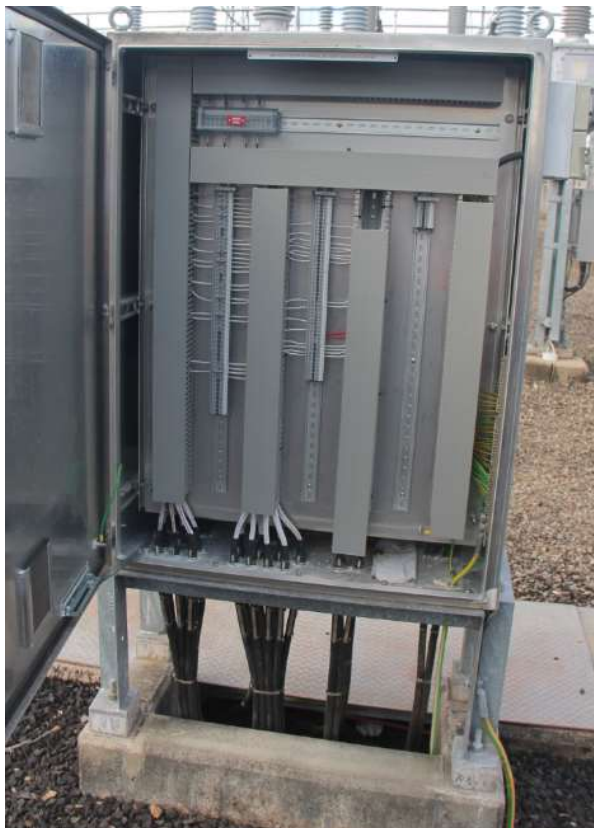
132kV Bay =D06 Feeder 7192 bay marshalling kiosk
