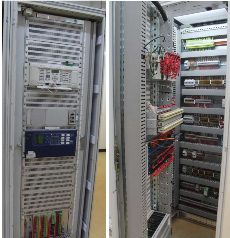
Feeder 876 bay protection/control panel
