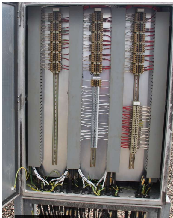
275kV Feeder 857 bay marshalling kiosk
