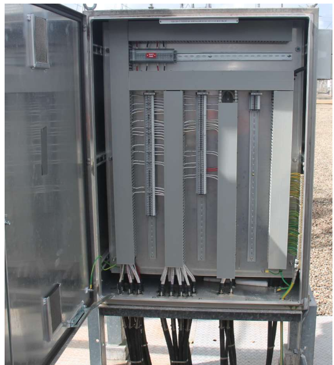
132kV Bay =D07 Feeder 7166 bay marshalling kiosk
