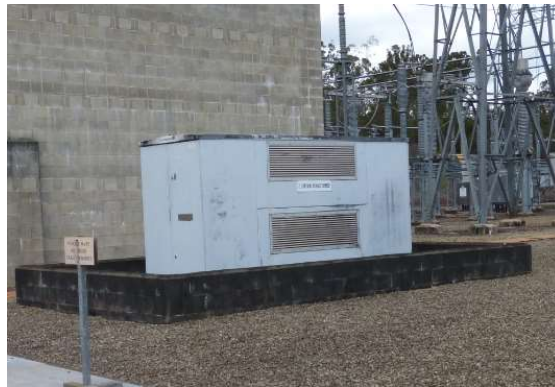
Figure 13 - 1 T station supply transformer
