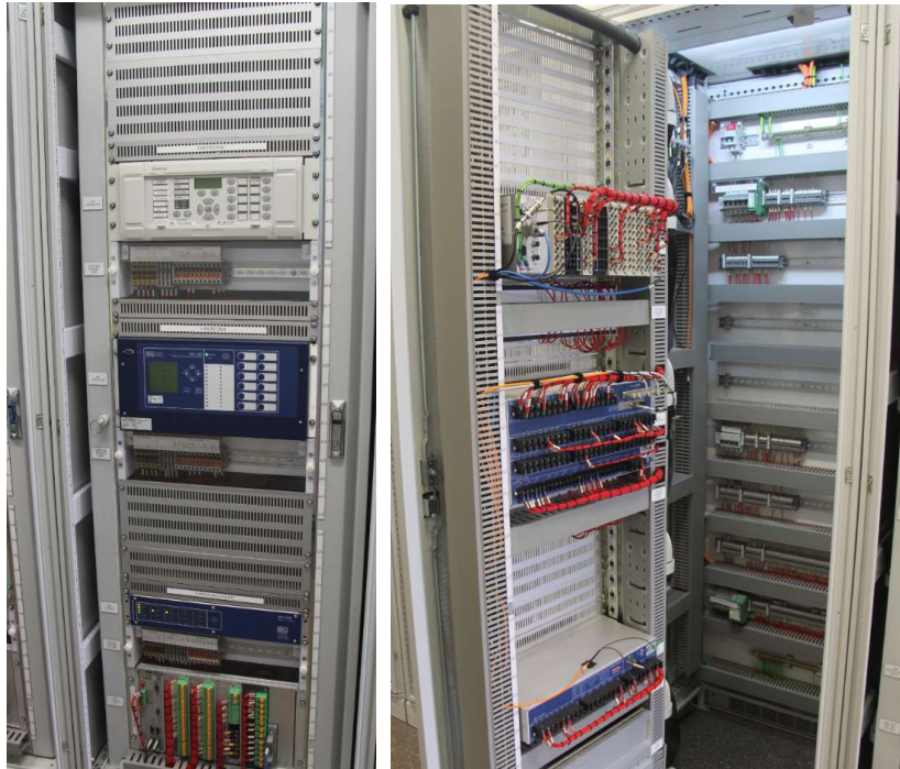
Feeder 7191 protection and control panel
