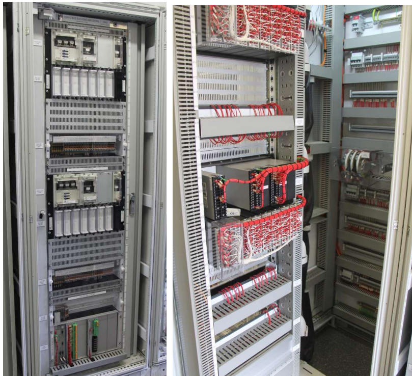
132kV 2 Bus zone protection and control panel
