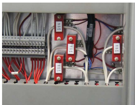
Hathaway travelling wave fault locator
