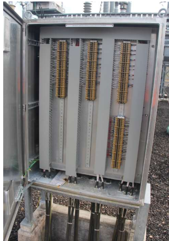
132kV Bay =D06 Feeder 7192 bay marshalling kiosk
