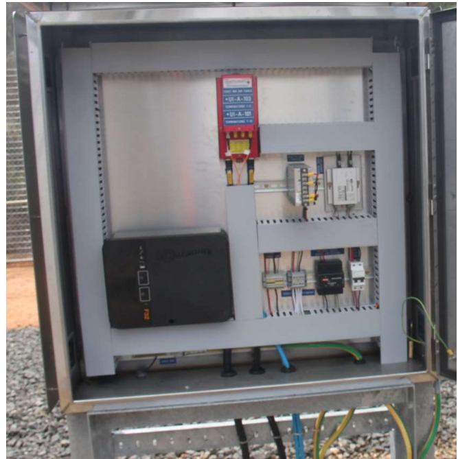
Electric fence and associated control cubicle
