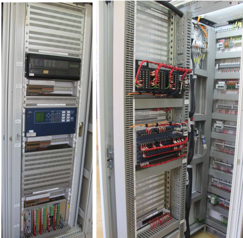
Coupler 504 protection/control panel
