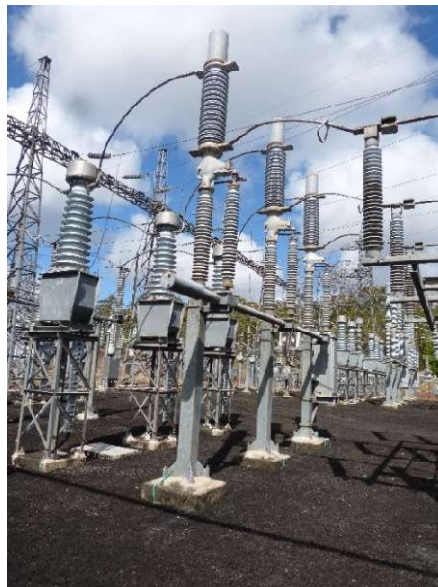
Figure 9 – HLR Circuit Breaker
