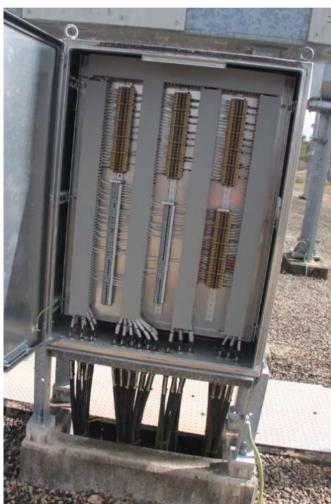
132kV Bay =D03 coupler 411 marshalling kiosk
