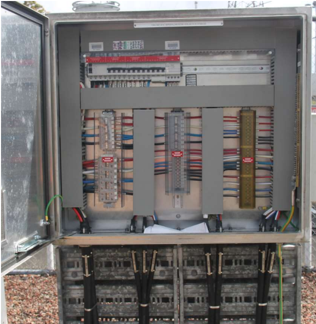
132kV Bay =D08 AC and DC marshalling kiosk
