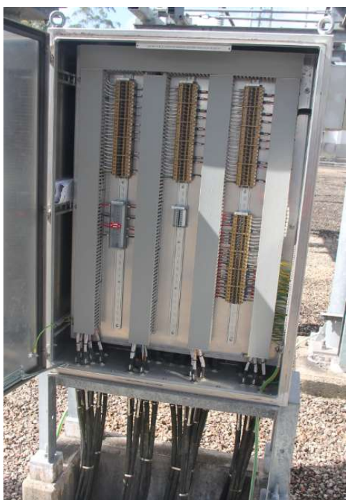
132kV Bay =D03 coupler 411 marshalling kiosk
