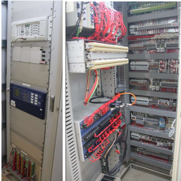
Feeder 877 bay protection/control panel
