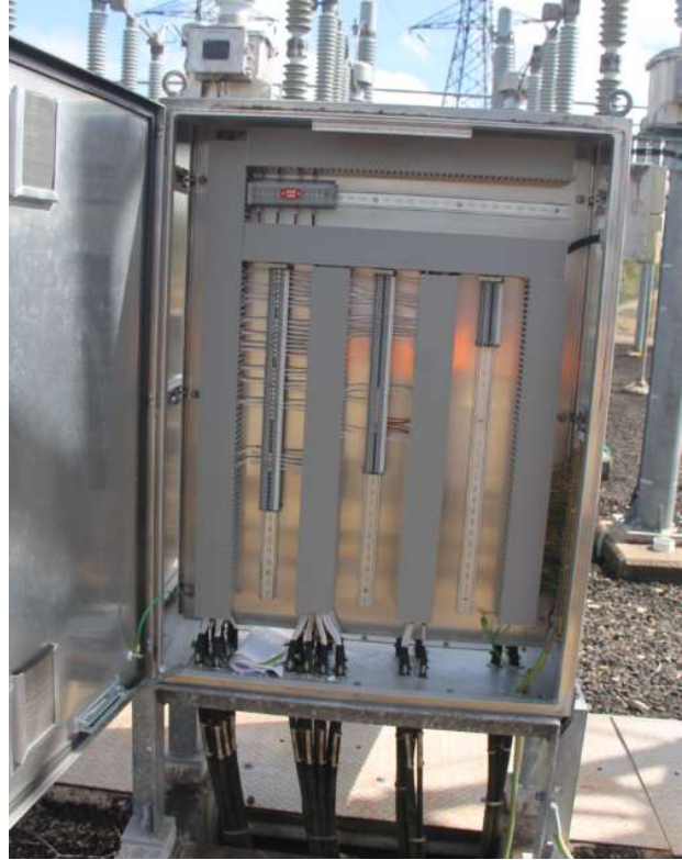
132kV Bay =D06 2 Transformer LV bay marshalling kiosk
