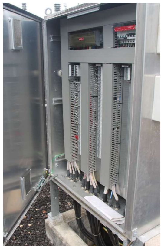
275kV Feeder 857 reactor marshalling kiosk
