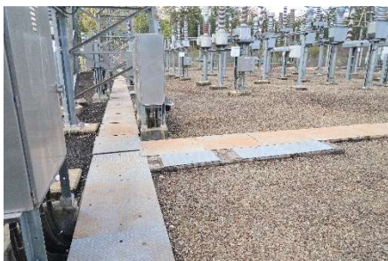
Figure 17 – Cable trenches
