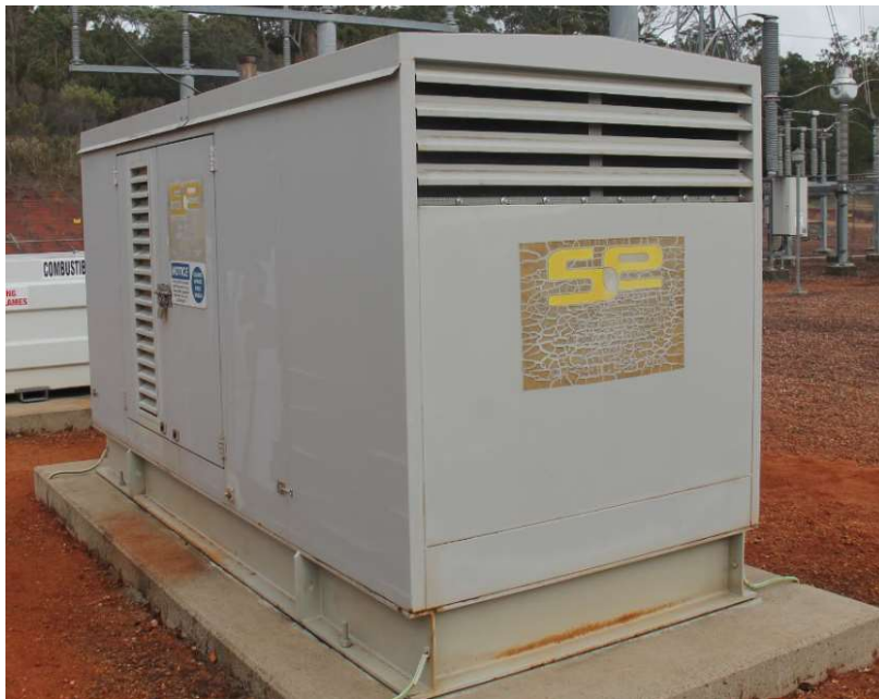
On site diesel generator
