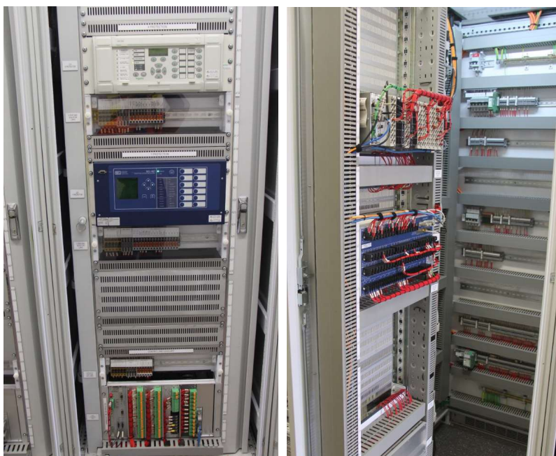
Feeder 7166 protection and control panel
