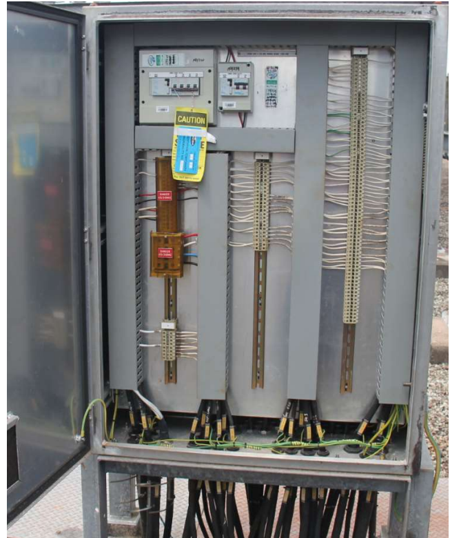
275kV Feeder 858 bay marshalling kiosk
