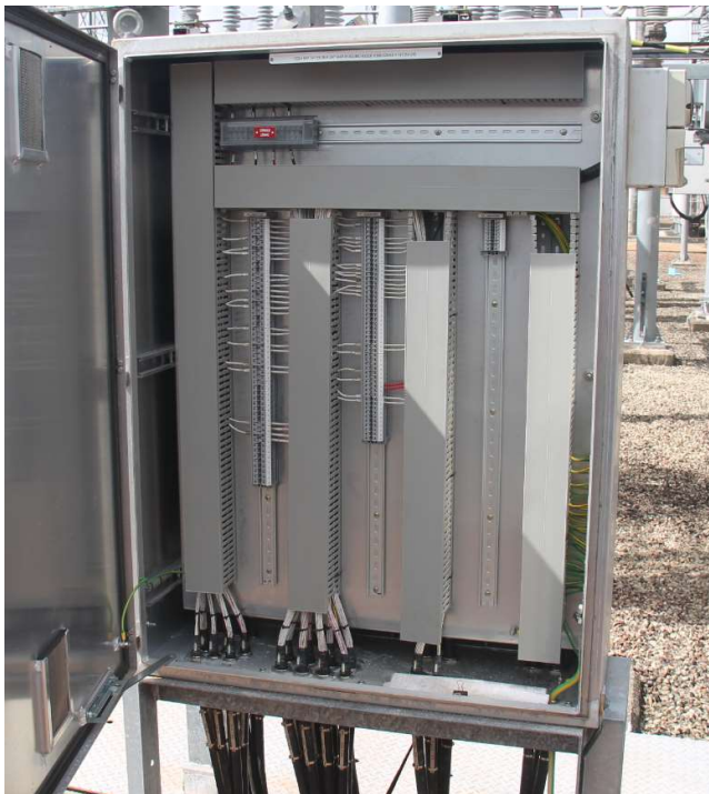
132kV Bay =D08 Feeder 7165 bay marshalling kiosk
