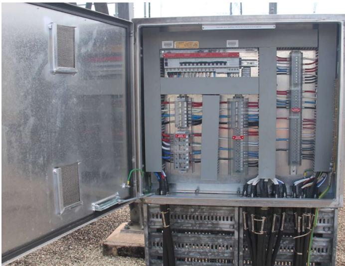
275kV =C04 AC and DC marshalling kiosk
