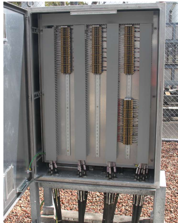
132kV Bay =D08 Feeder 7165 bay marshalling kiosk
