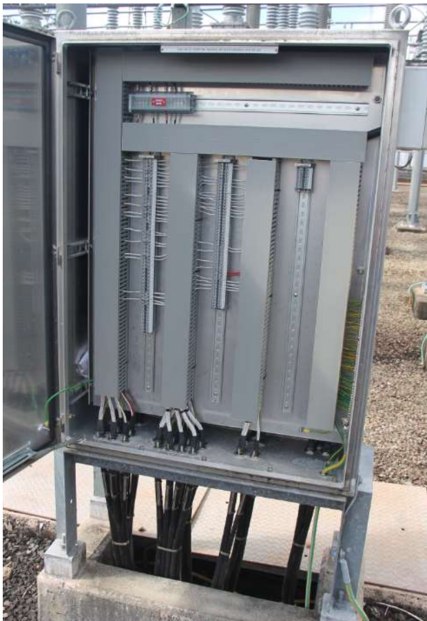
132kV Bay =D05 Feeder 7191 bay marshalling kiosk
