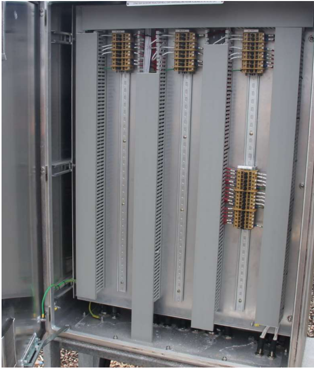
275kV Feeder 858 reactor marshalling kiosk
