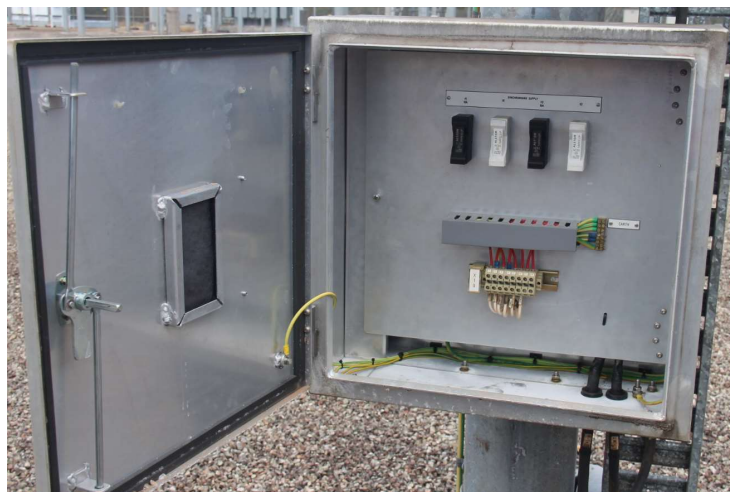
275kV Feeder 877 13 and 18 VT marshalling kiosk
