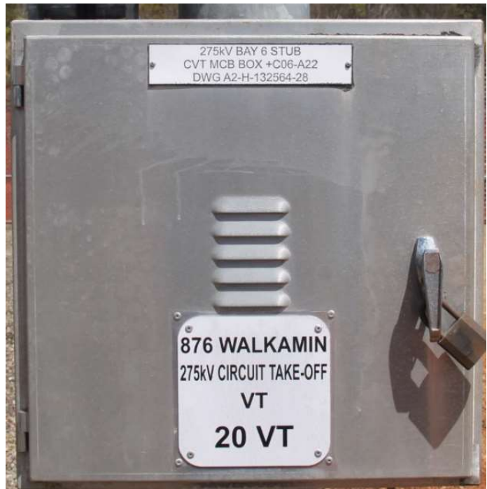
275kV feeder 876 19 and 20 VT marshalling kiosk
