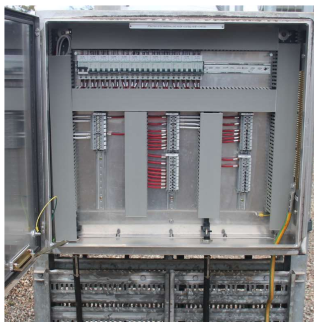
275kV =C05 AC and DC marshalling kiosk
