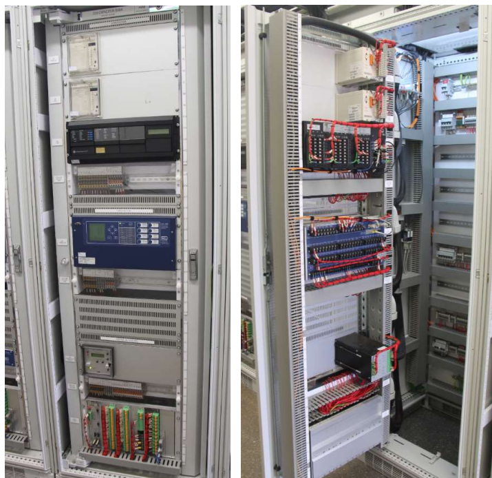
1 CAP protection and control panel
