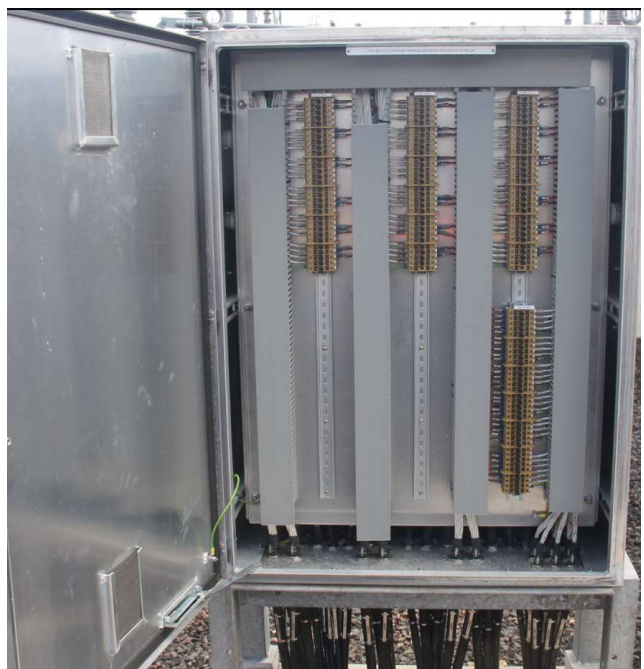
275kV Bay 3 coupler bay marshalling kiosk
