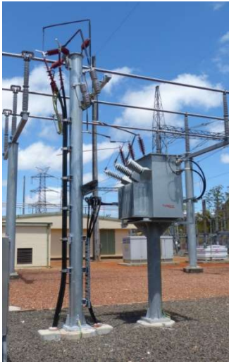
Figure 12 -2 T station supply transformer
