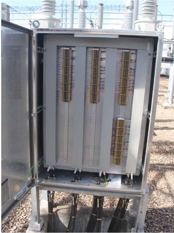
132kV Bay =D06 2 Transformer LV bay marshalling kiosk
