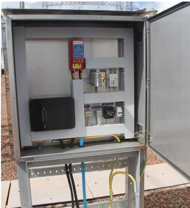
Electric fence and associated control cubicle
