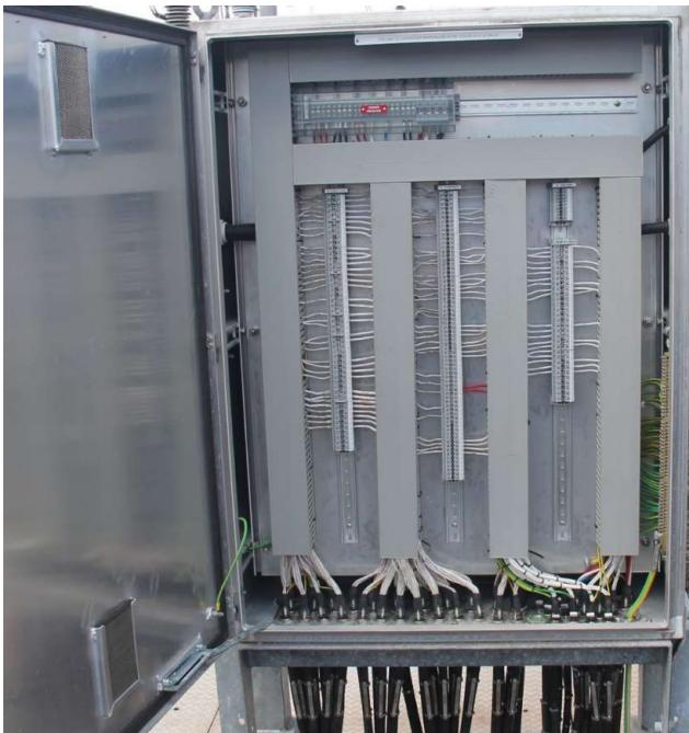
275kV Bay 3 coupler bay marshalling kiosk
