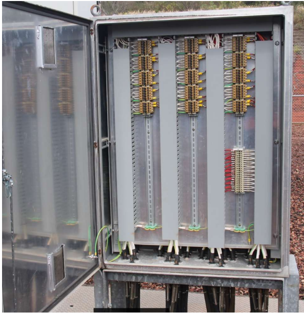
275kV Feeder 876 bay marshalling kiosk
