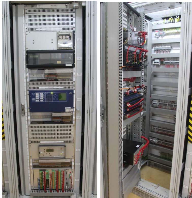
858 feeder reactor protection and control panel
