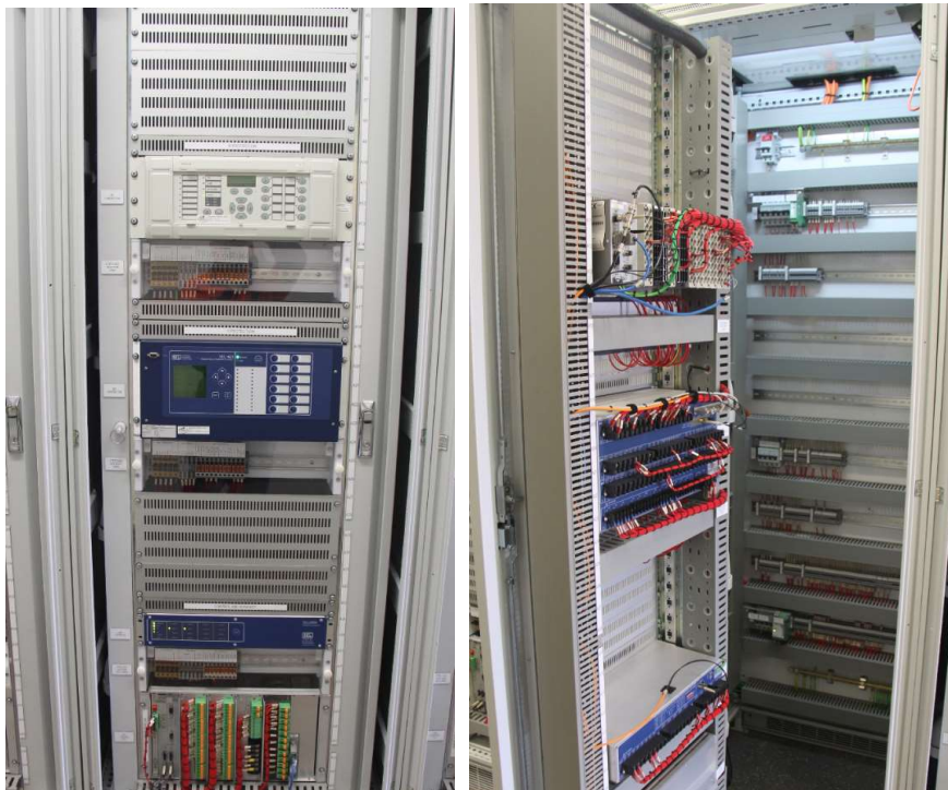
Feeder 7192 protection and control panel
