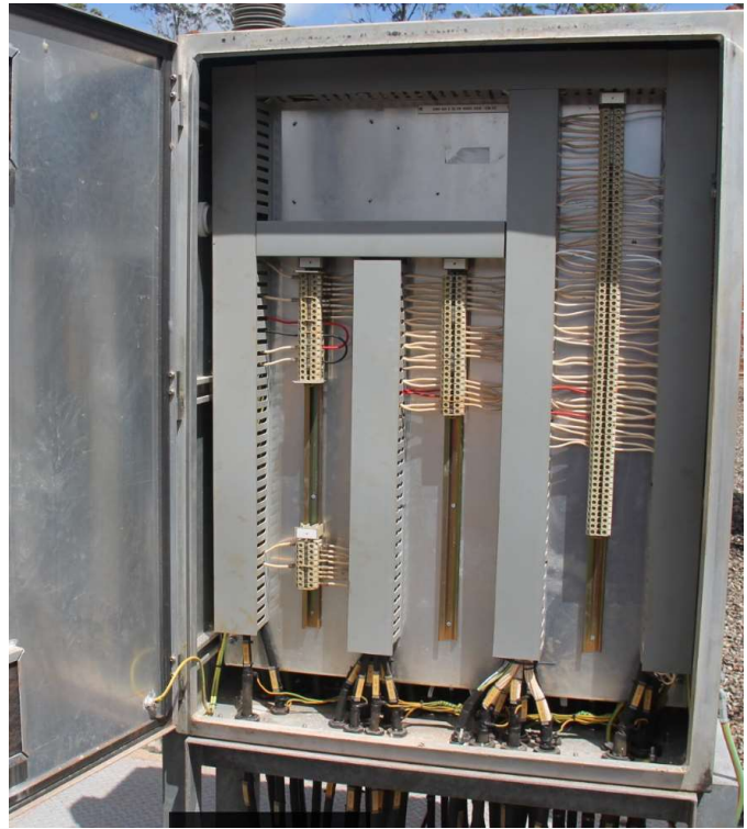
275kV Feeder 877 bay marshalling kiosk
