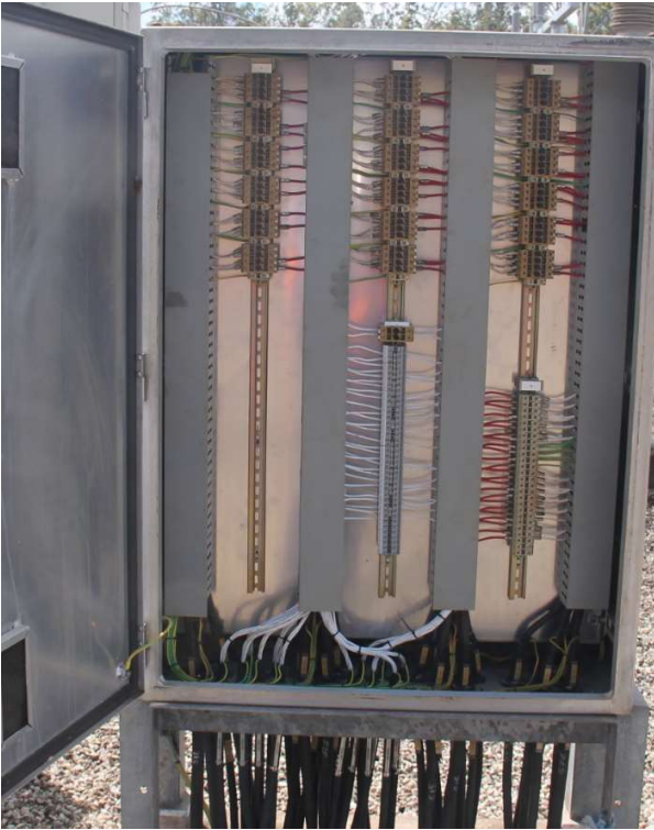
275kV Feeder 877 bay marshalling kiosk
