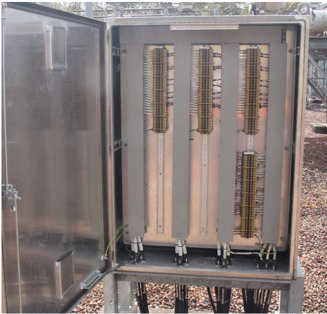
132kV =D09 1 CAP bay marshalling kiosk
