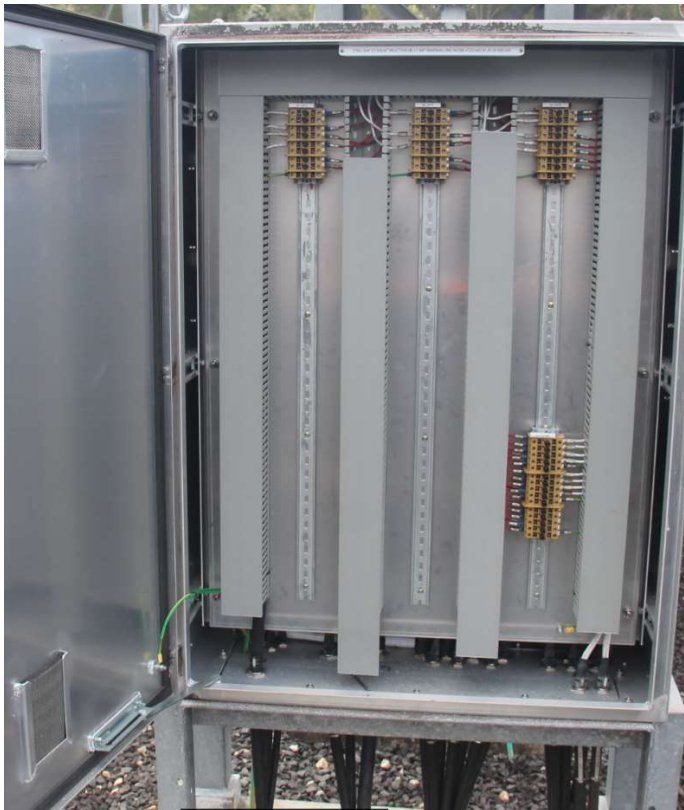
275kV Feeder 857 reactor marshalling kiosk
