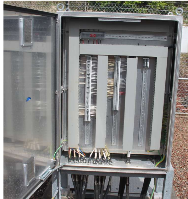
132kV =D09 1 CAP bay marshalling kiosk
