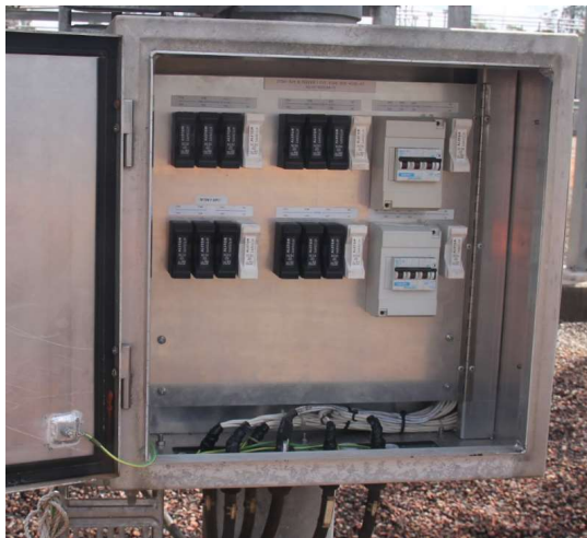
275kV Feeder 877 13 and 18 VT marshalling kiosk
