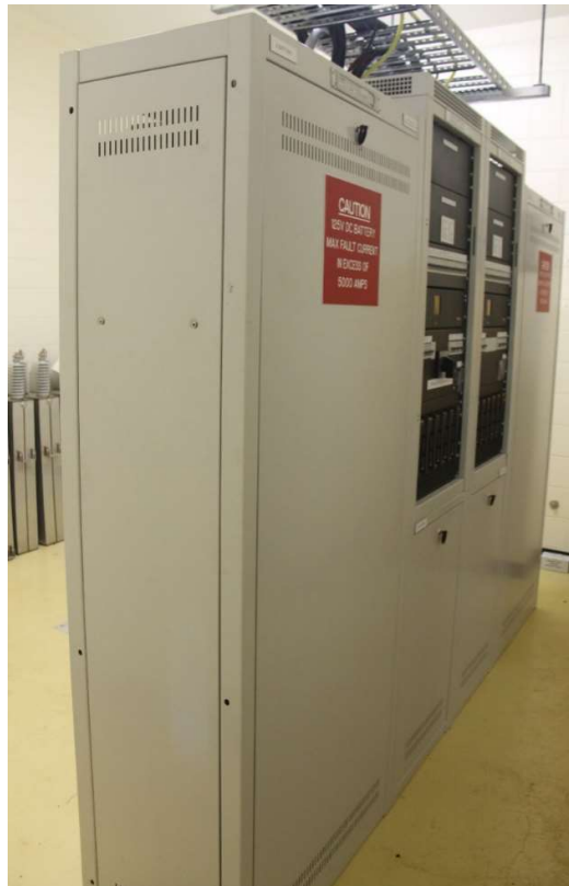
125VDC Batteries and charger
