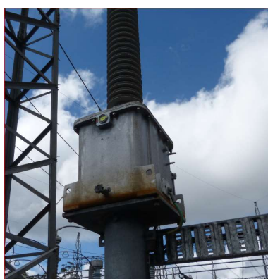
Figure 11 - CVT corrosion
