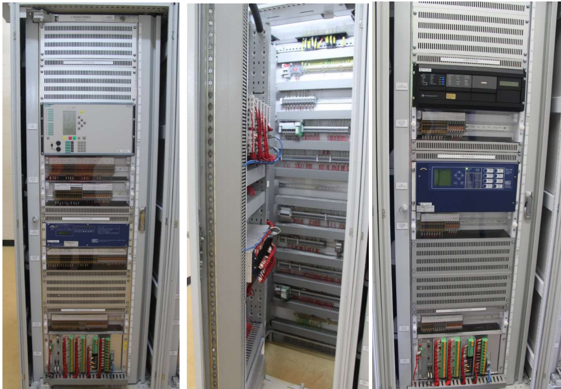
1 Transformer 275/132kV protection and control panel
