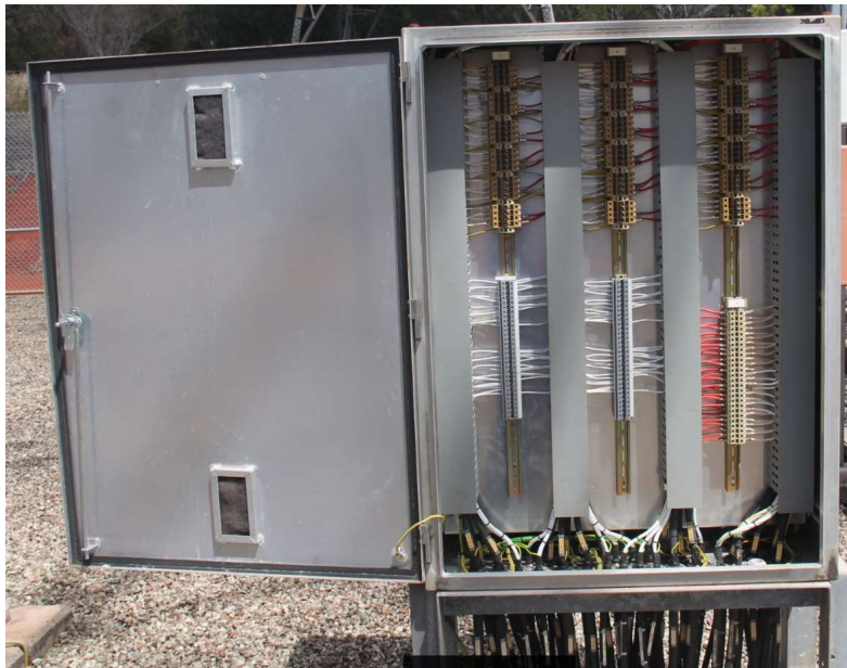
275kV Bay 6 coupler bay marshalling kiosk
