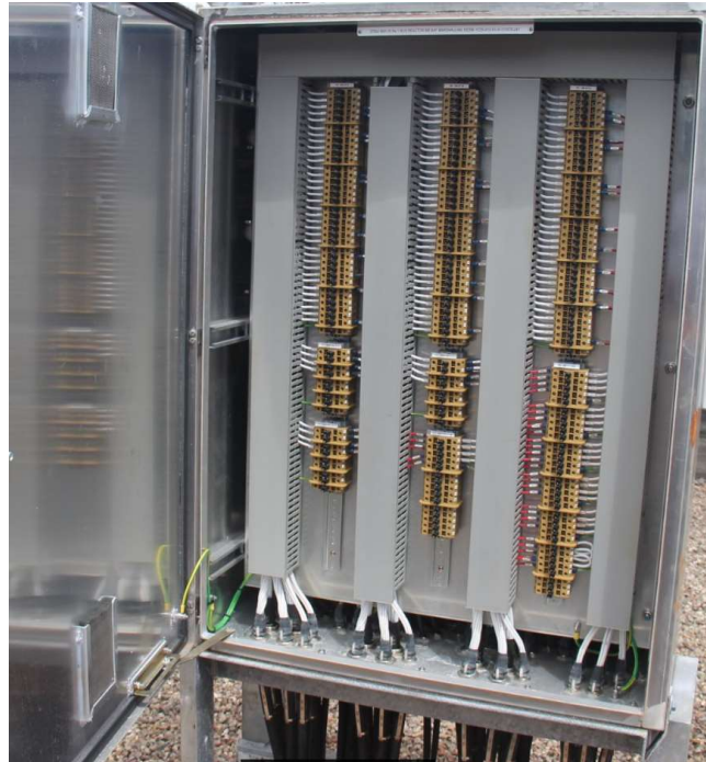
275kV bus reactor 5 bay marshalling kiosk
