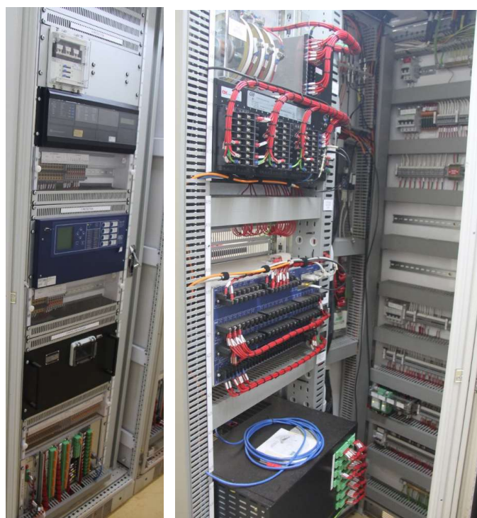
275kV Bus reactor protection and control panel
