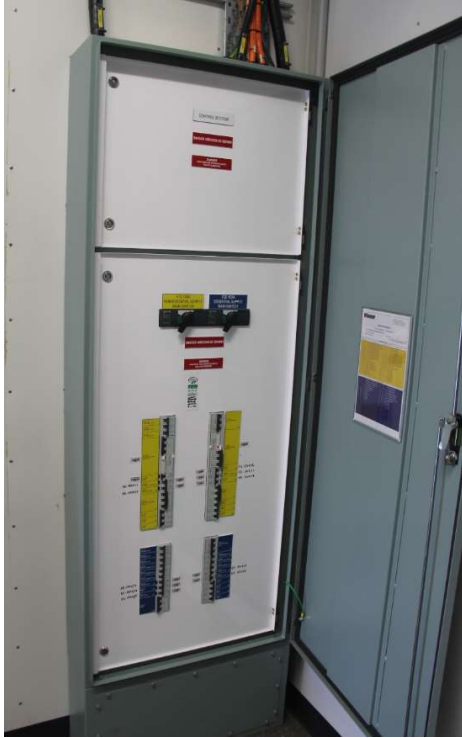
AC distribution boards in building +4
