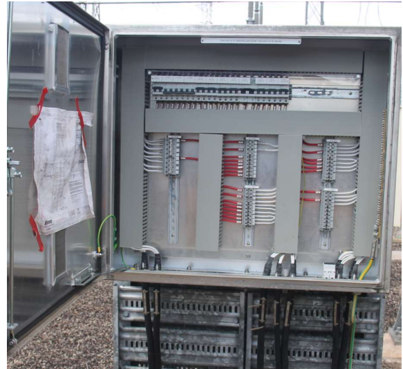
275kV =C04 AC and DC marshalling kiosk
