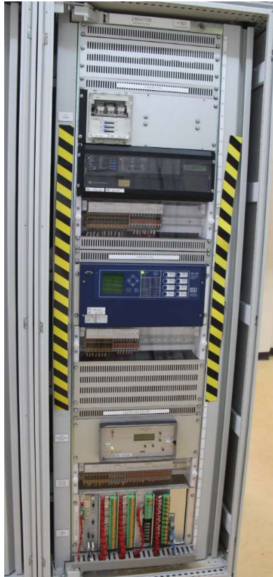
857 feeder reactor protection and control panel
