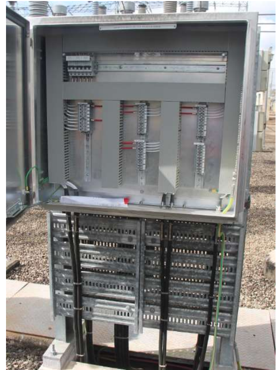
132kV Bay =D06 AC and DC marshalling kiosks
