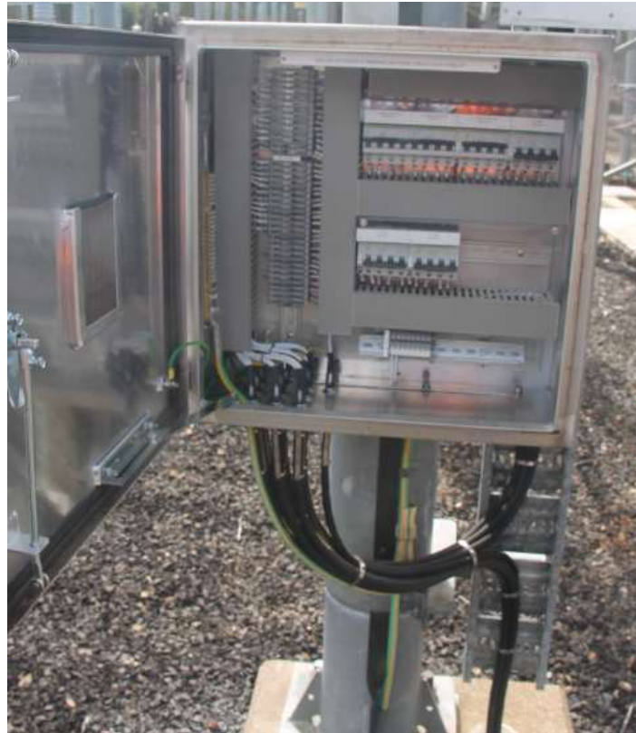
132kV Bay =D06 Feeder 7192 6VT box
