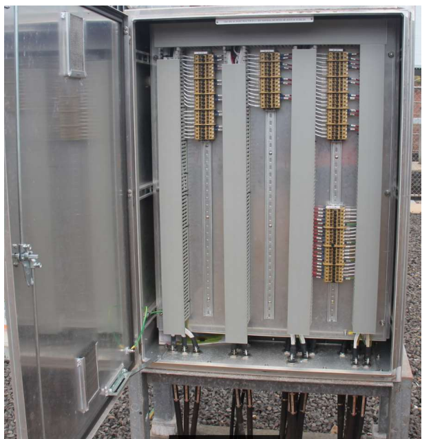
132kV 1T shunt reactor marshalling kiosk
