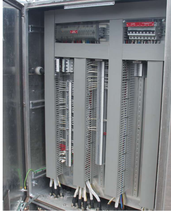
275kV Feeder 858 reactor marshalling kiosk
