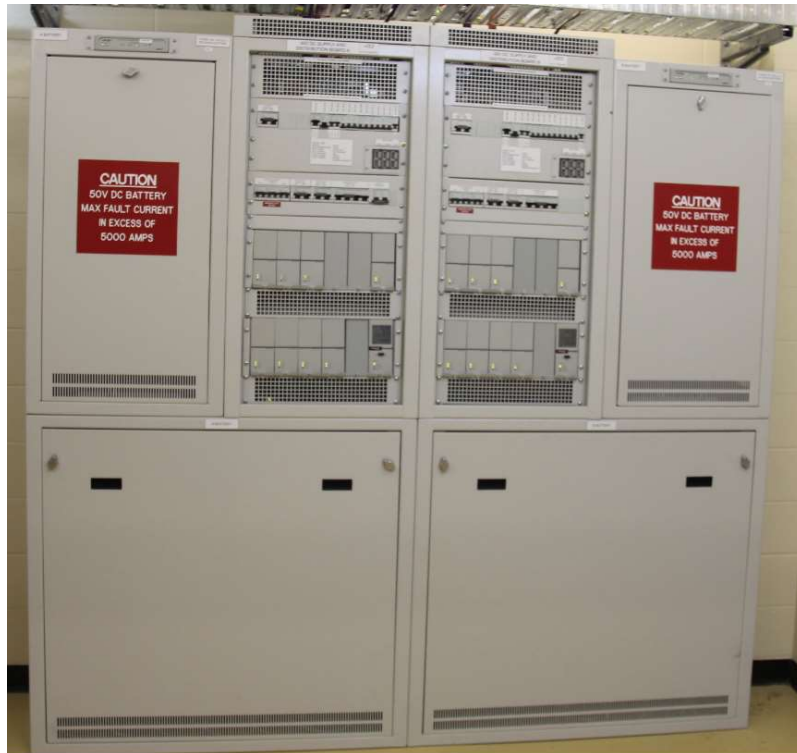
48VDC Batteries and charger in building +1
