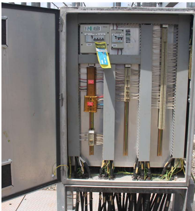
275kV Feeder 857 bay marshalling kiosk
