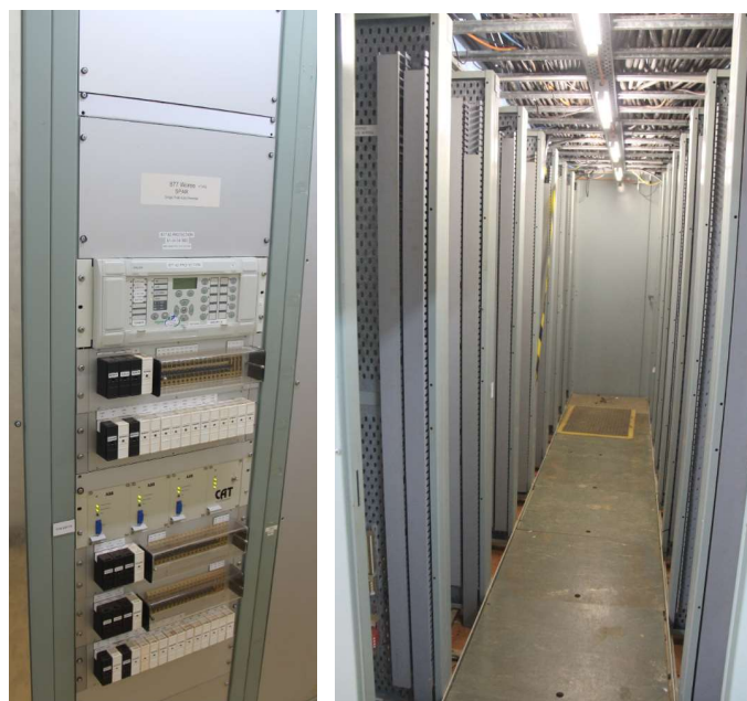
Feeder 877 SPAR scheme panel
