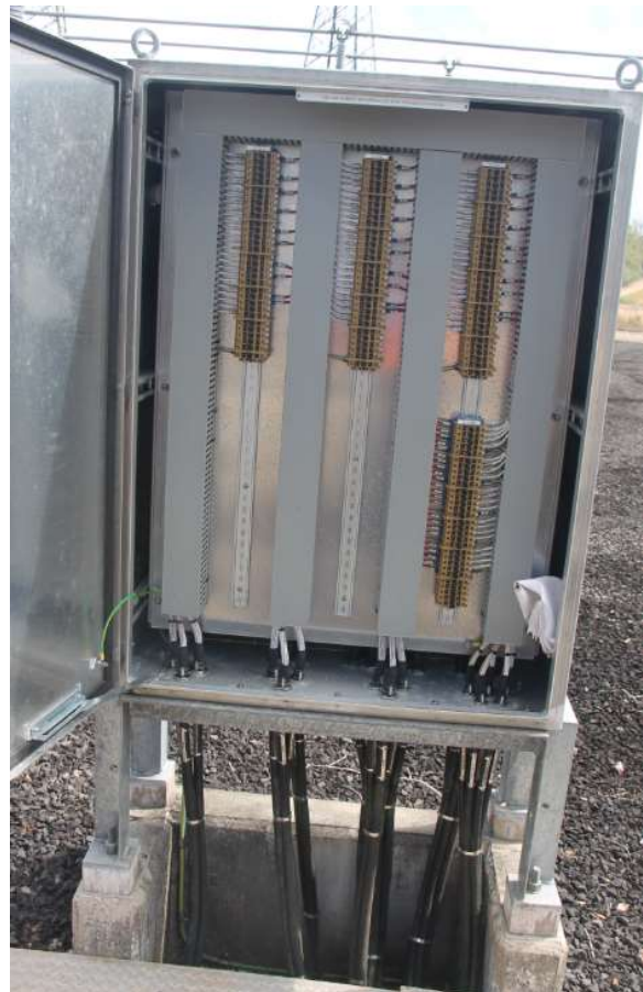
132kV Bay =D05 Feeder 7191 bay marshalling kiosk
