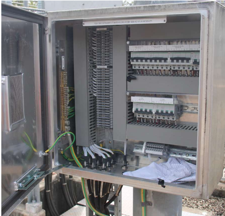
132kV Bay =D08 Feeder 7165 8VT box
