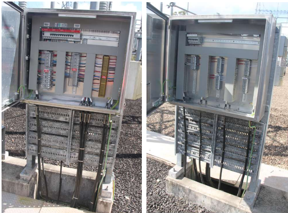
132kV Bay =D04 AC and DC marshalling kiosks
