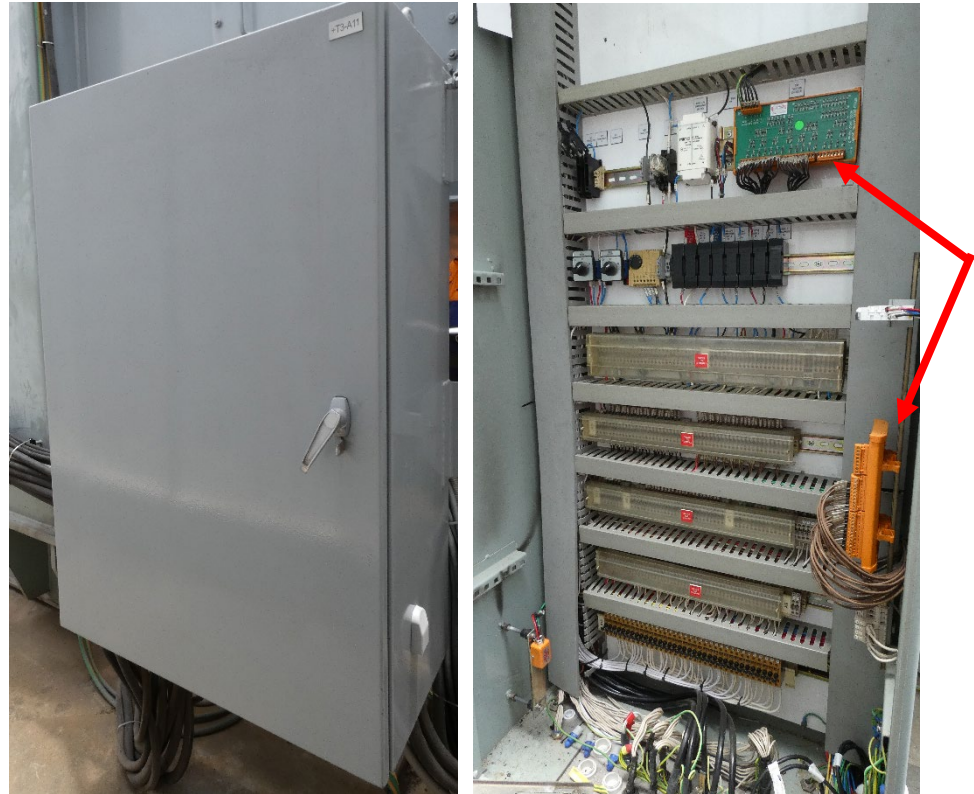
Figure 27: Main Control Cubicle view with the outer door open. Note dual OLTC TPI cards, one for PLQ and one for Energy Queensland.
