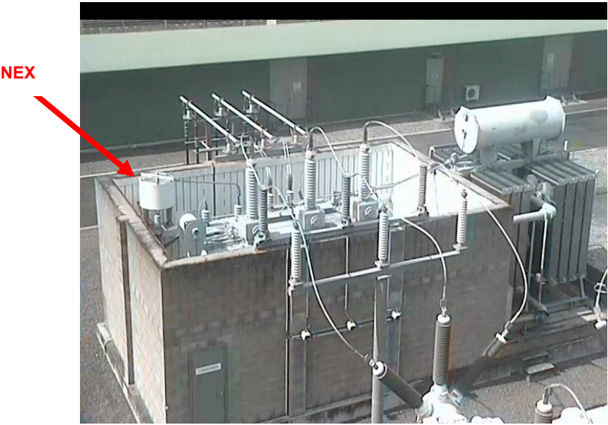
Figure 6: T142 Tennyson transformer T03 installed inside a sound wall enclosure. Note the NEX installed on a steel post near the OLTC oil conservator.
