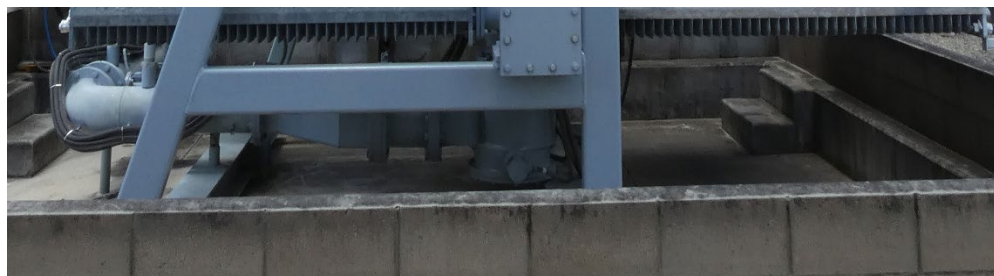
Figure 17: View under and around the Cooler Bank. No oil residue or pooling
