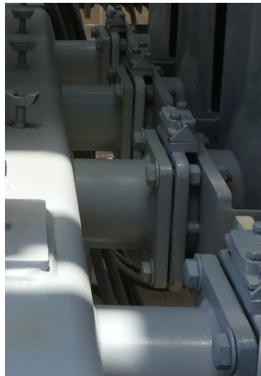
Figure 20: Butterfly valves are installed for isolating each of the radiator panels from the top and bottom main oil headers.
