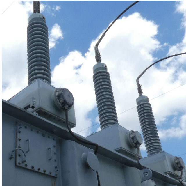
Figure 33: 110kV OIP HV bushings are shown.
