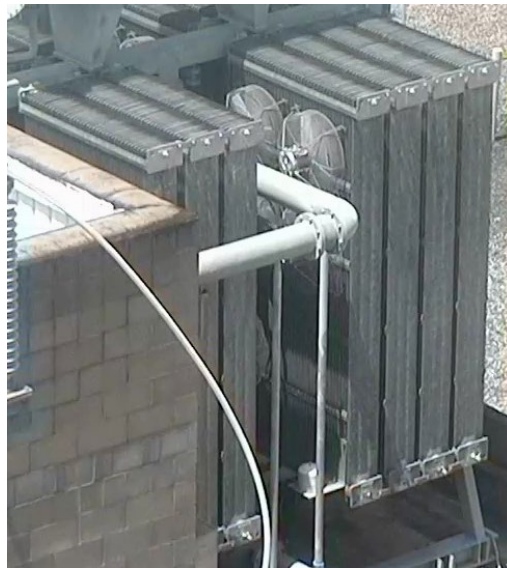
Figure 14: View of the Cooler Bank with galvanised radiator panels and painted support structures.
