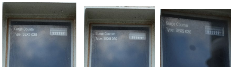
Figure 53: Readings on the lightning surge counters installed on the 110kV bushings from left to right are 26, 07 and 07.
