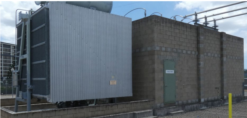
Figure 6: T142 Tennyson transformer T03 installed inside a sound wall enclosure. Note the NEX installed on a steel post near the OLTC oil conservator.
