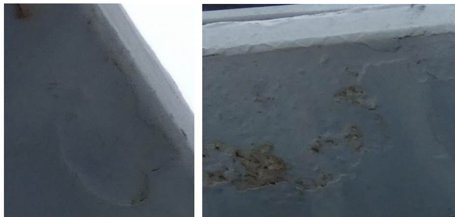
Figure 13: A close-up of the paint damage under the main tank flange is visible. Damaged area has just a colour coating applied over it.
