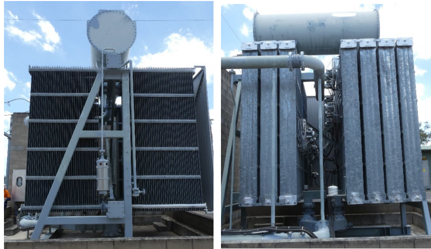
Figure 15: (LHS) View of the outer Cooler Bank 'A'-frame support structure.
