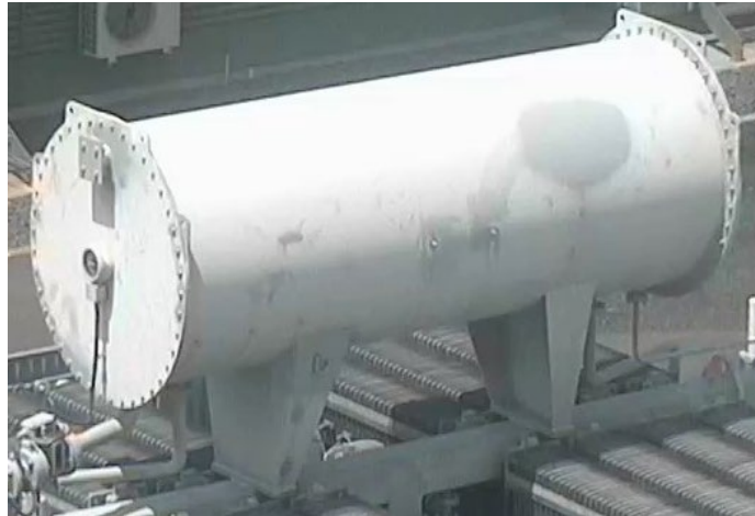
Figure 21: The main oil conservator showing oxidised paint and some local paint touch-ups.
