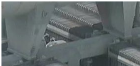
Figure 22: There is no sign of corrosion where the main oil conservator support structure is welded to the top main oil header.
