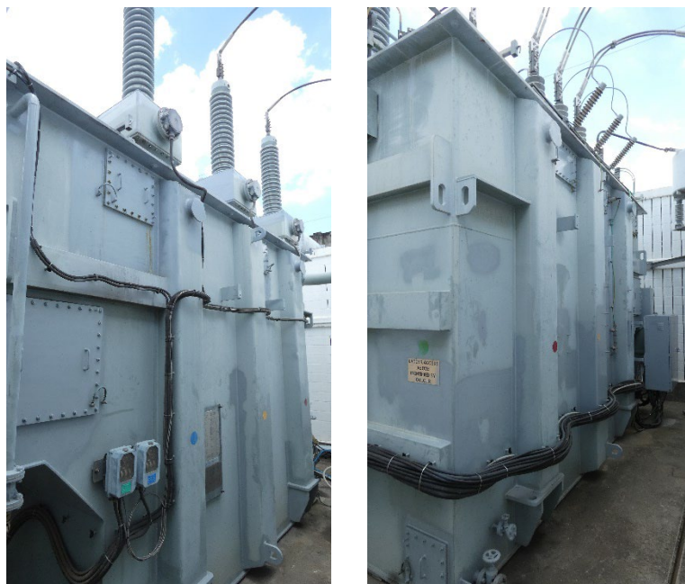
Figure 8: (LHS) Tennyson T03 HV side. (RHS) A view of the LV side. Note the paint touch-ups.
