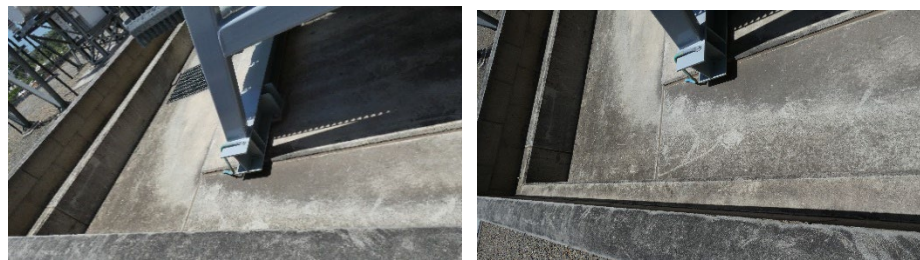
Figure 16: View under and around the Cooler Bank. No oil residue or pooling.
