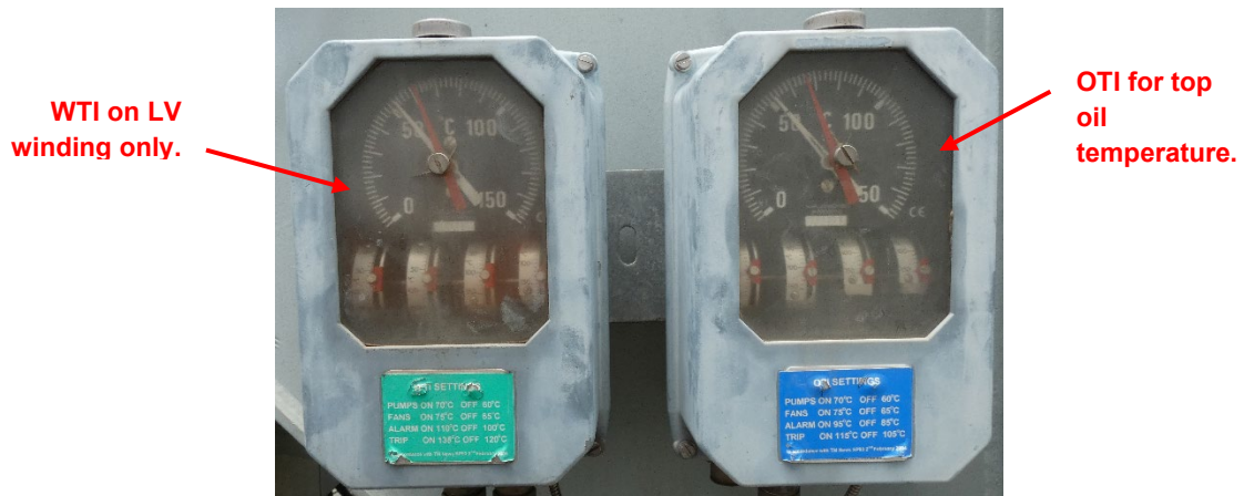
Figure 26: One WTI and one OTI are installed.
