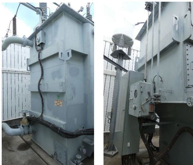
Figure 8: (LHS) Tennyson T03 HV side. (RHS) A view of the LV side. Note the paint touch-ups.
