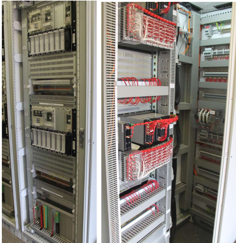
132kV 1 Bus zone protection and control panel
