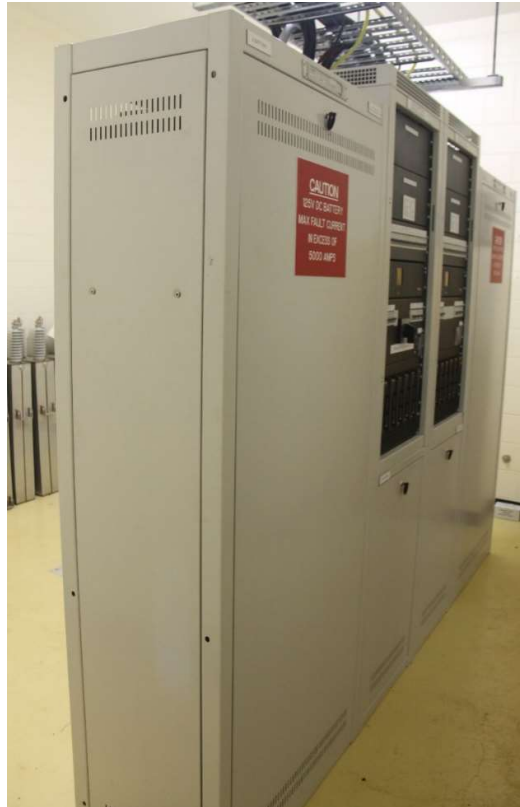
125VDC Batteries and charger
