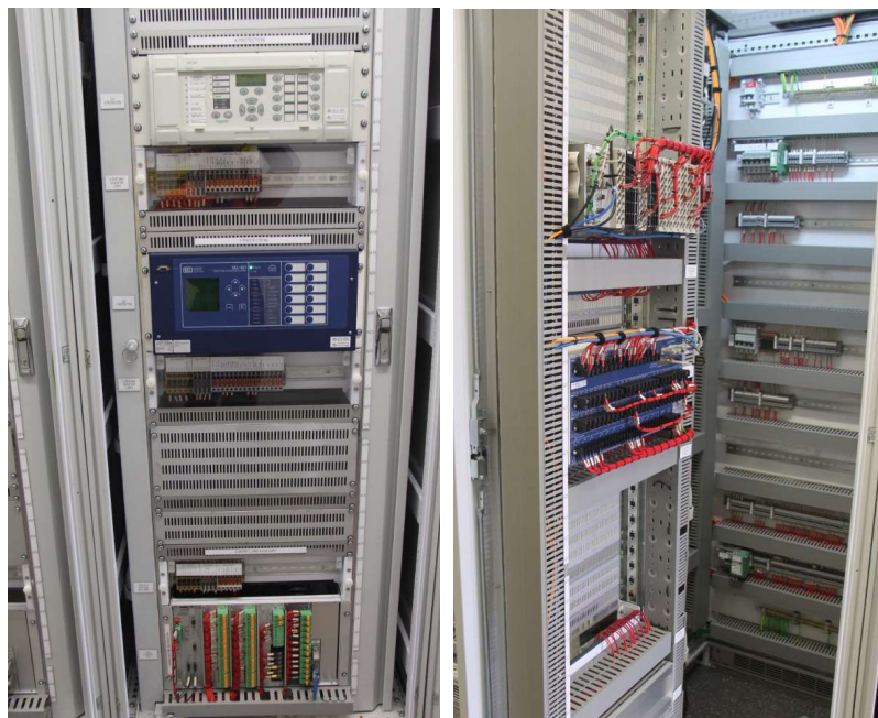
Feeder 7166 protection and control panel
