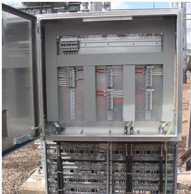
132kV Bay =D08 AC and DC marshalling kiosk
