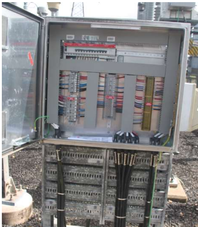
132kV Bay =D06 AC and DC marshalling kiosks
