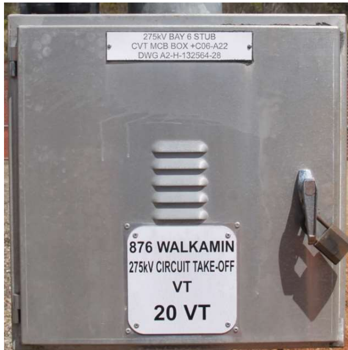
275kV feeder 876 19 and 20 VT marshalling kiosk
