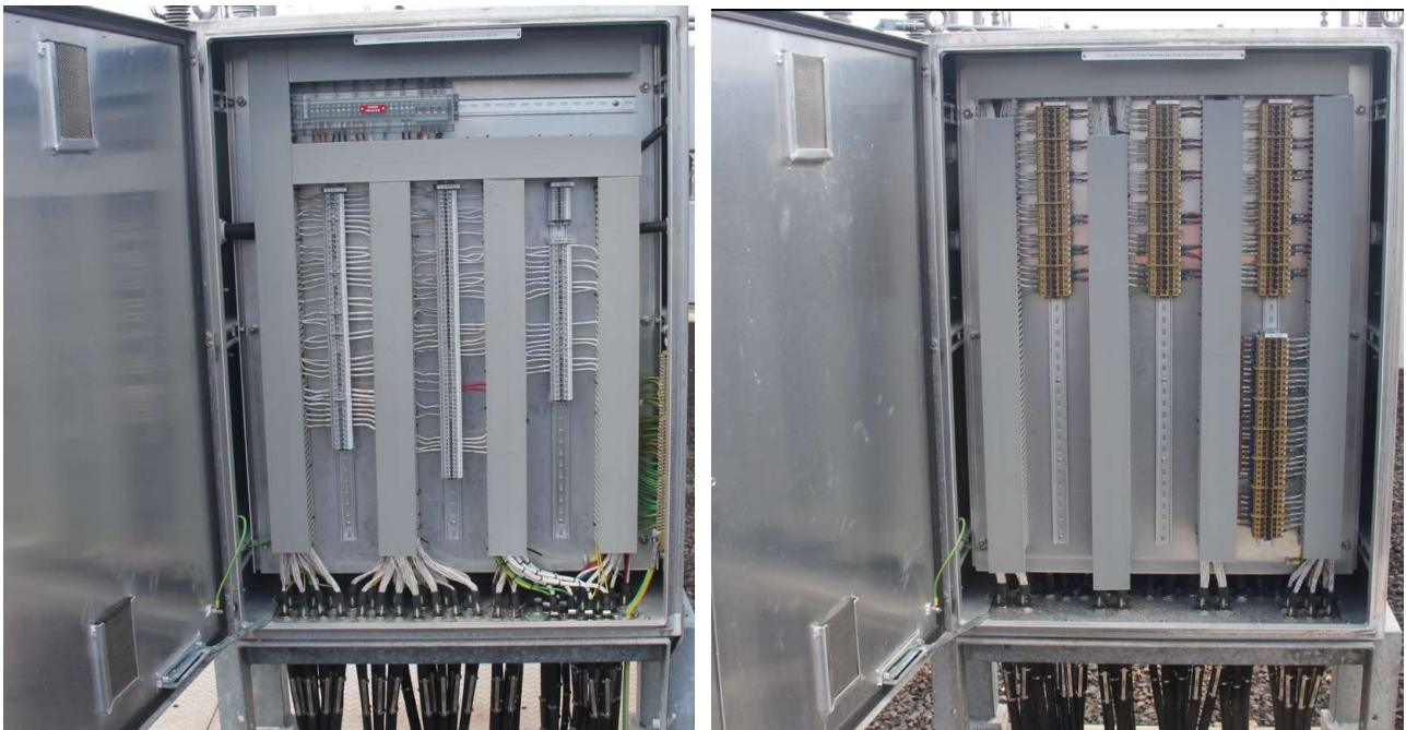
275kV Bay 3 coupler bay marshalling kiosk
