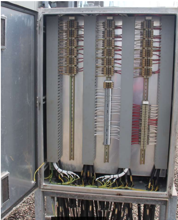
275kV Feeder 858 bay marshalling kiosk
