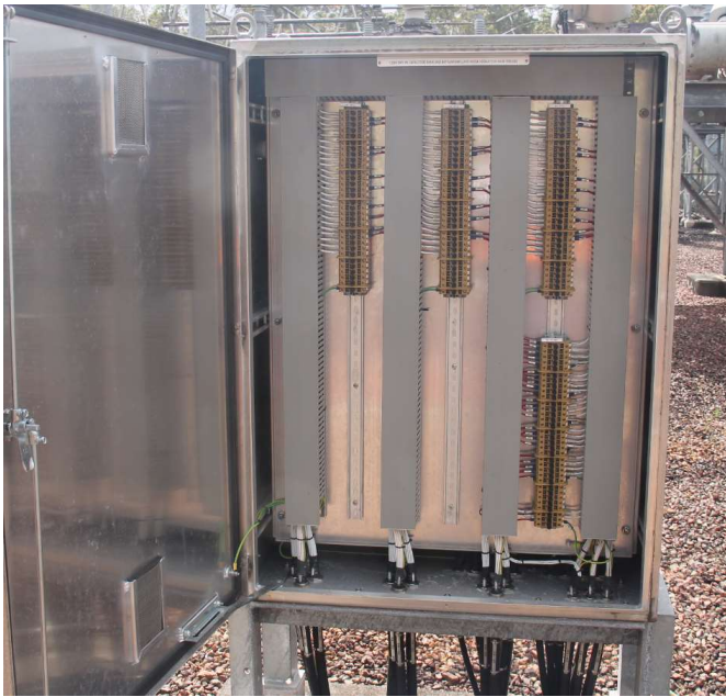
132kV =D09 1 CAP bay marshalling kiosk
