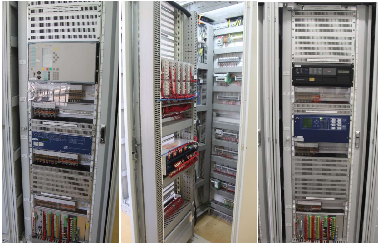
2 Transformer 275/132kV protection and control panel
