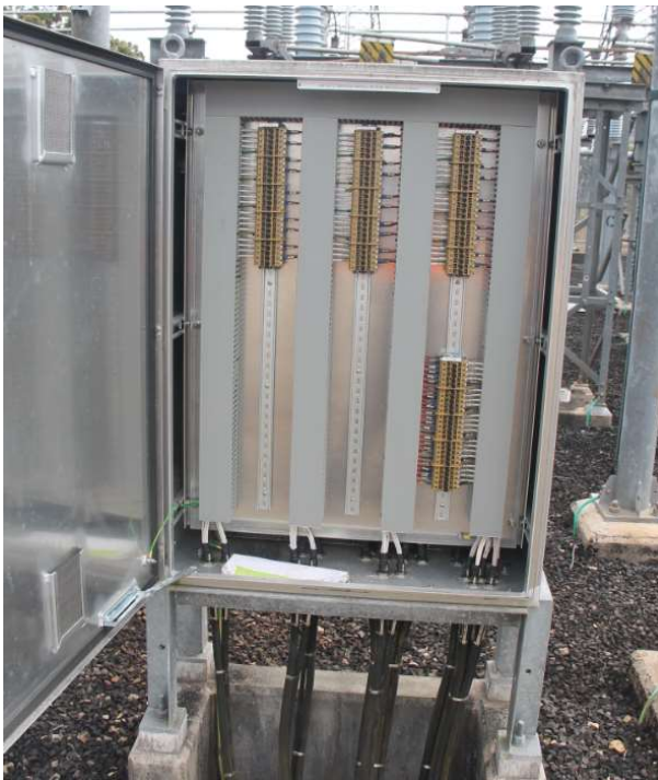
132kV Bay =D07 Feeder 7166 bay marshalling kiosk
