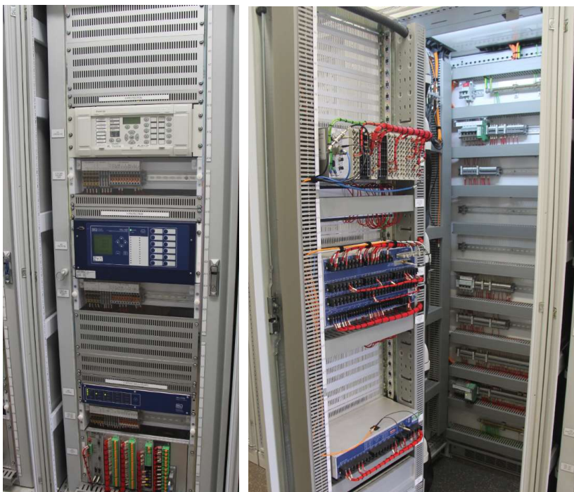
Feeder 7191 protection and control panel
