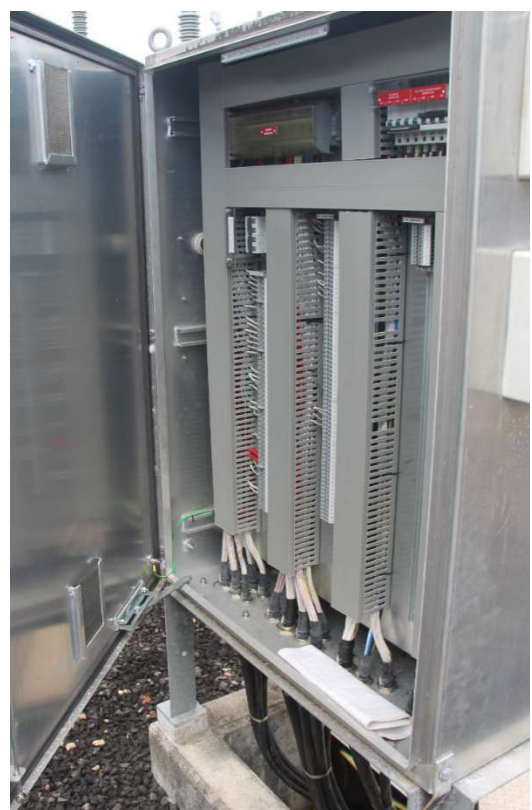
275kV Feeder 857 reactor marshalling kiosk
