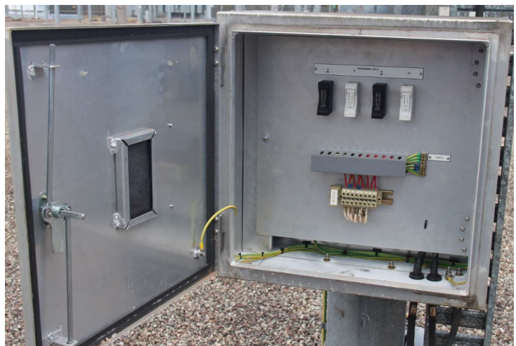
275kV Feeder 877 13 and 18 VT marshalling kiosk
