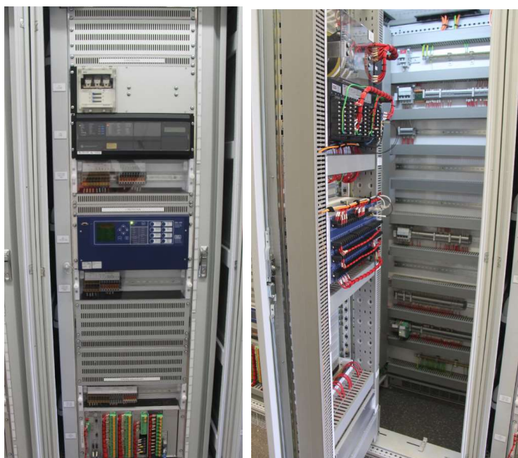
19kV Reactor protection and control panel
