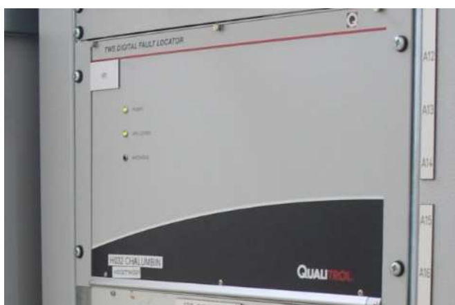
Hathaway travelling wave fault locator
