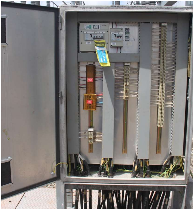
275kV Feeder 857 bay marshalling kiosk
