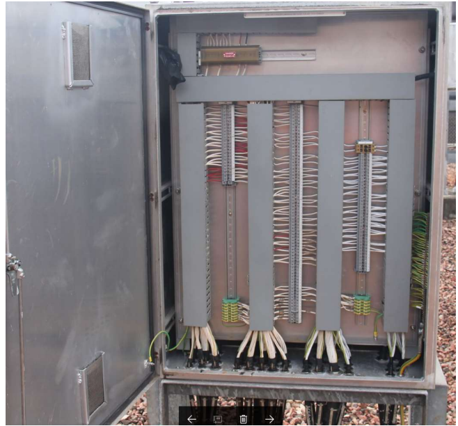
275kV Feeder 876 bay marshalling kiosk
