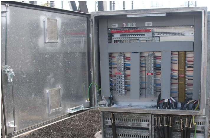
275kV =C03 AC and DC marshalling kiosk
