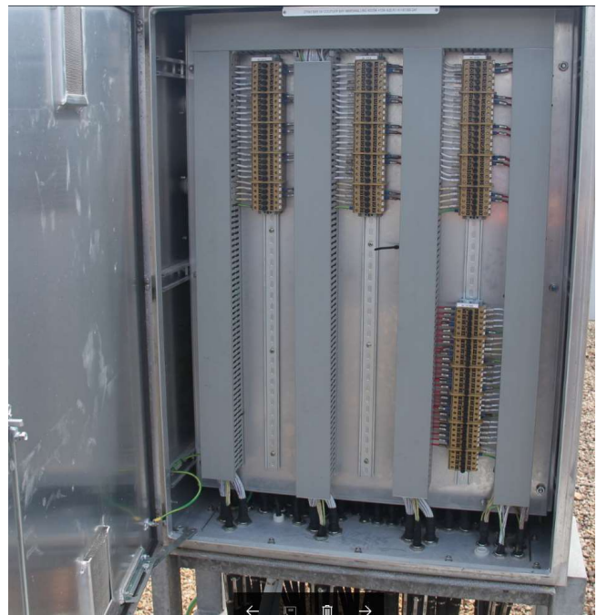
275kV Bay 4 coupler bay marshalling kiosk
