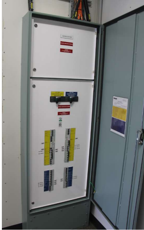
AC distribution boards in building +4
