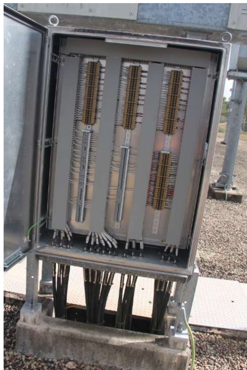
132kV Bay =D03 coupler 411 marshalling kiosk
