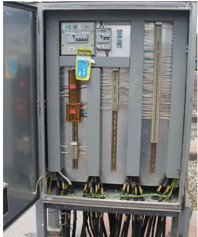
275kV Feeder 858 bay marshalling kiosk
