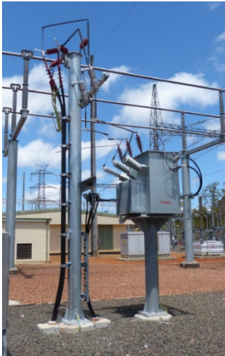
Figure 12 - 2 T station supply transformer
