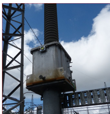
Figure 11 - CVT corrosion
