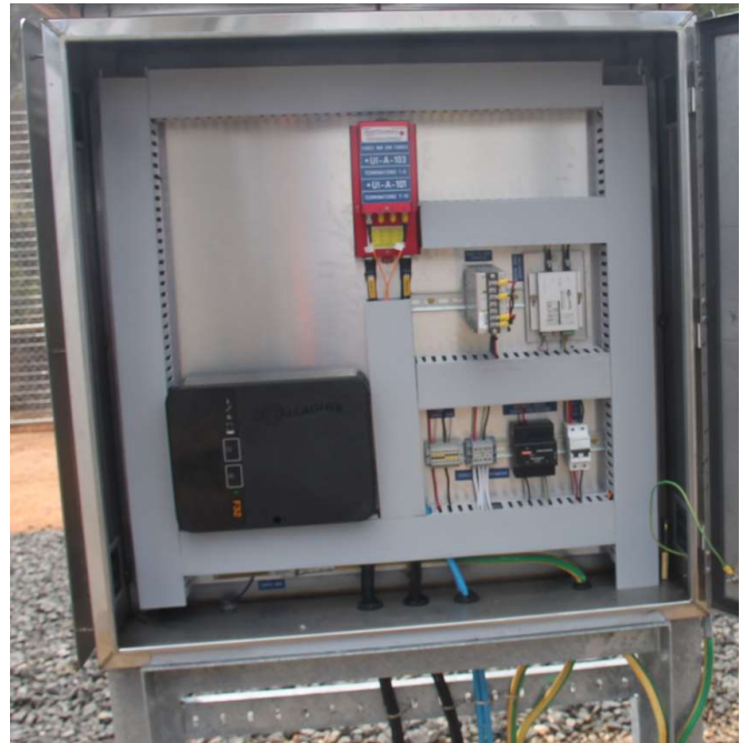
Electric fence and associated control cubicle
