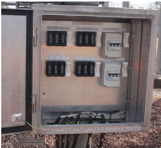
275kV Feeder 877 13 and 18 VT marshalling kiosk
