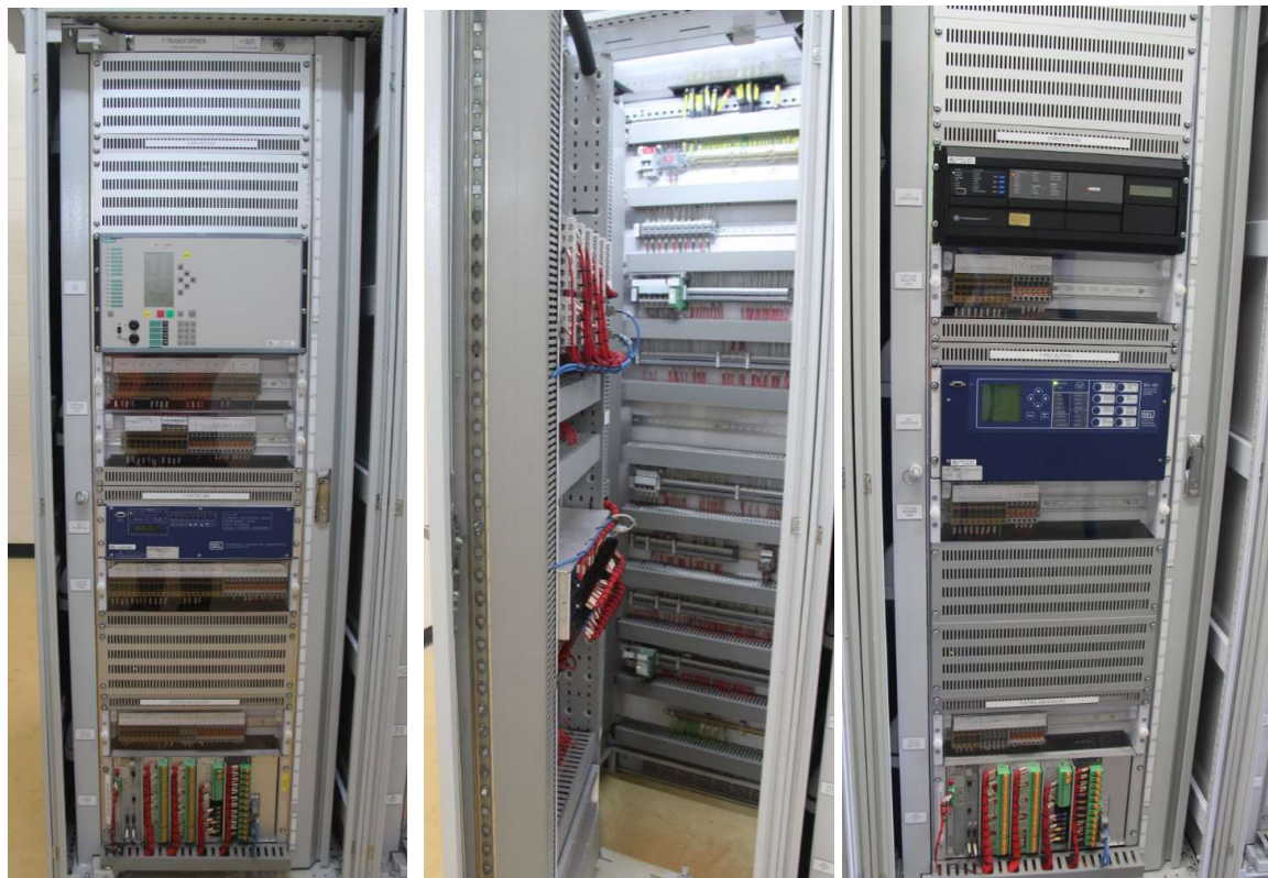
1 Transformer 275/132kV protection and control panel
