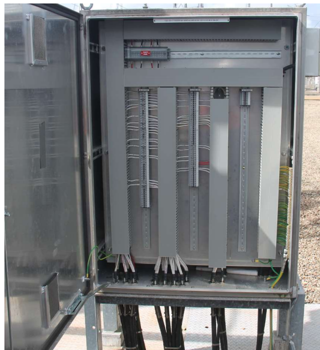
132kV Bay =D07 Feeder 7166 bay marshalling kiosk
