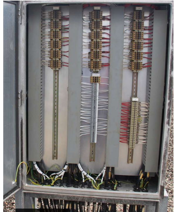
275kV Feeder 857 bay marshalling kiosk
