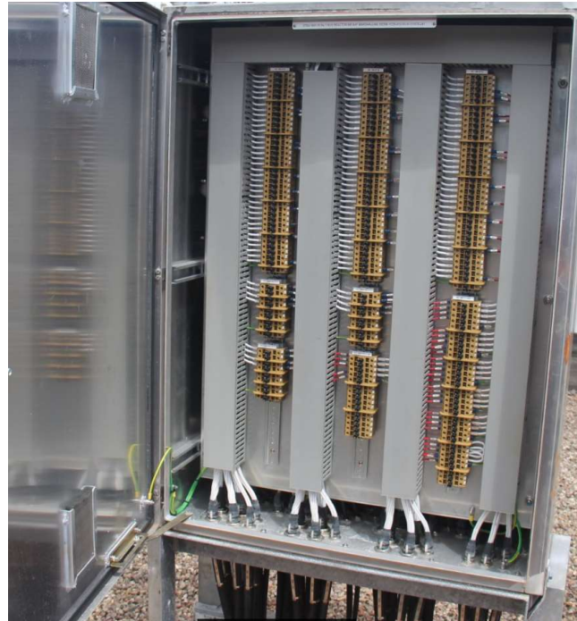
275kV bus reactor 5 bay marshalling kiosk
