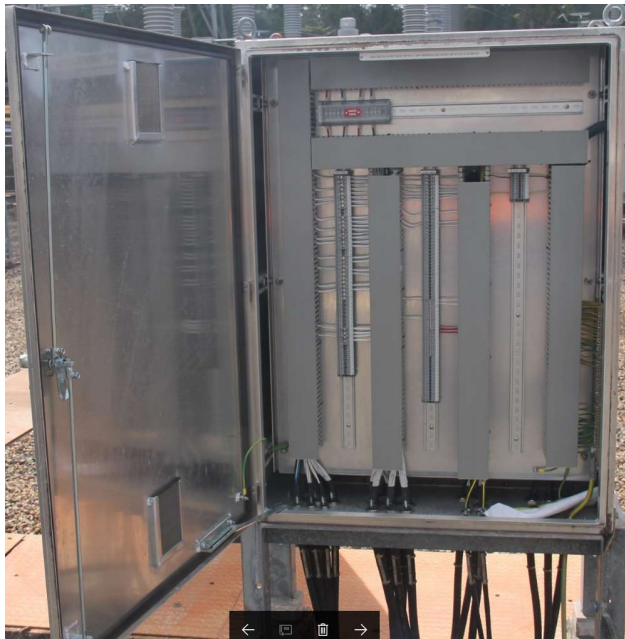
132kV 1T shunt reactor marshalling kiosk
