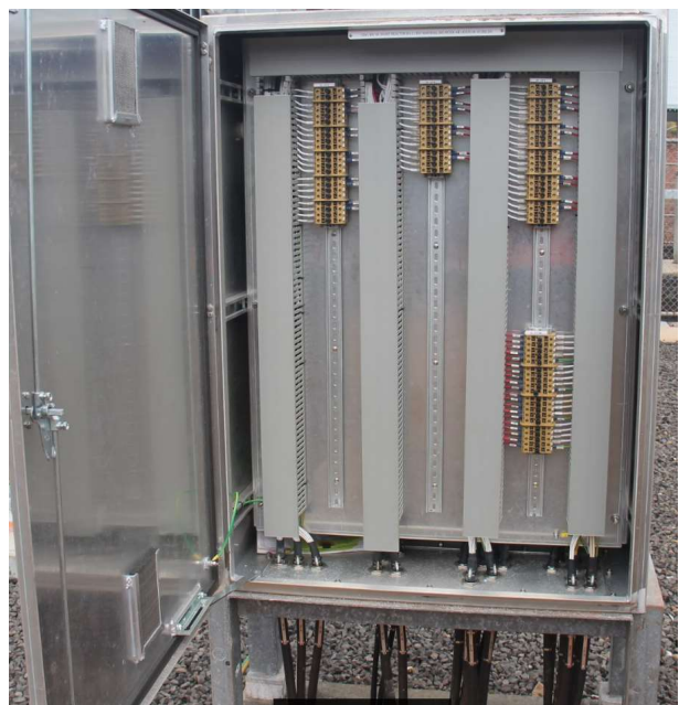
132kV 1T shunt reactor marshalling kiosk
