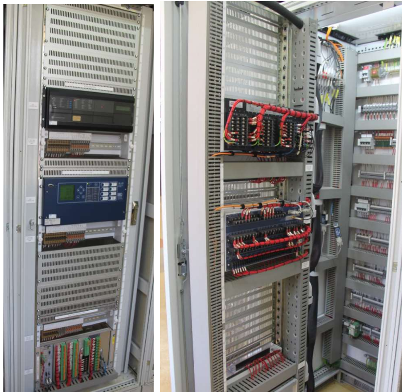
Coupler 504 protection/control panel
