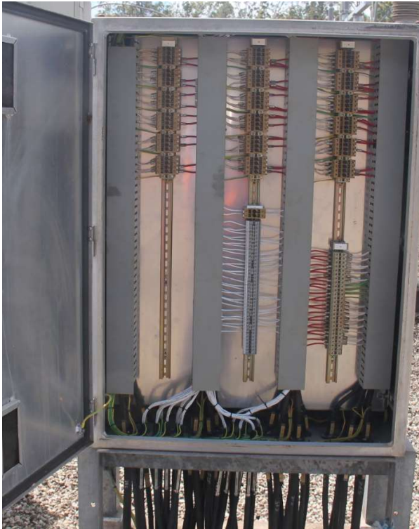
275kV Feeder 877 bay marshalling kiosk
