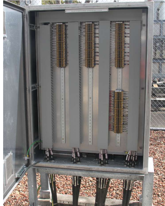
132kV Bay =D08 Feeder 7165 bay marshalling kiosk
