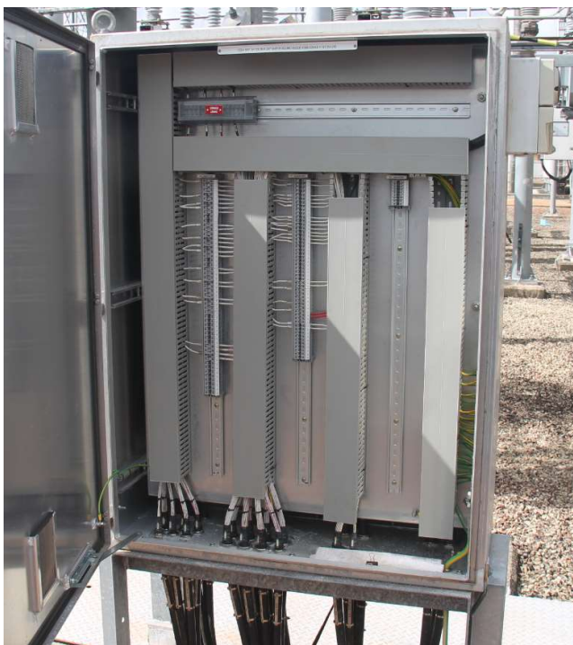
132kV Bay =D08 Feeder 7165 bay marshalling kiosk
