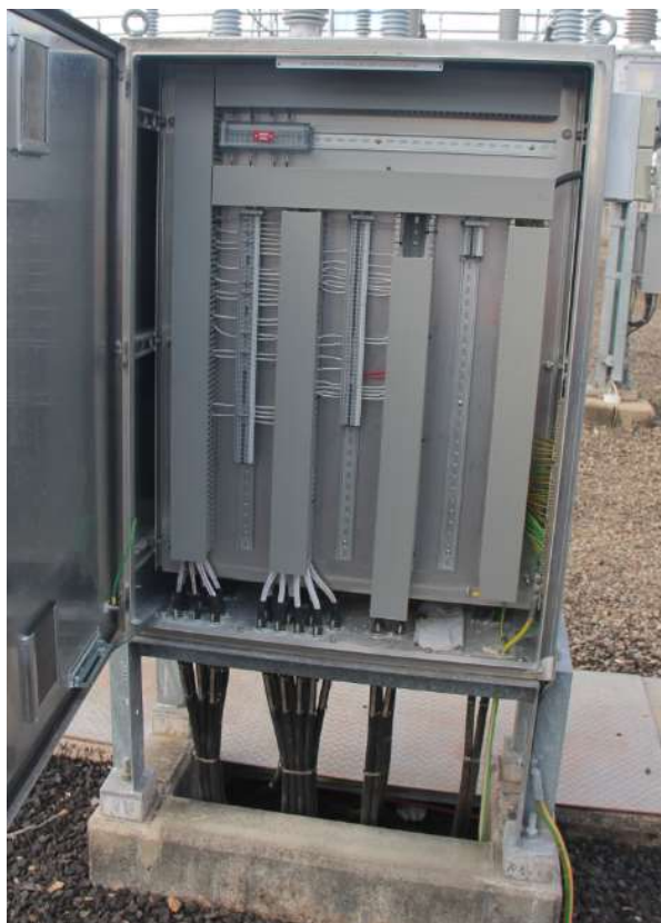
132kV Bay =D06 Feeder 7192 bay marshalling kiosk
