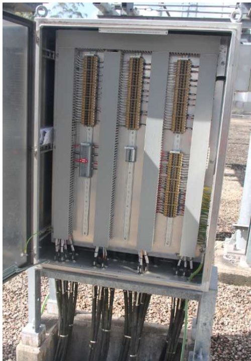
132kV Bay =D03 coupler 411 marshalling kiosk
