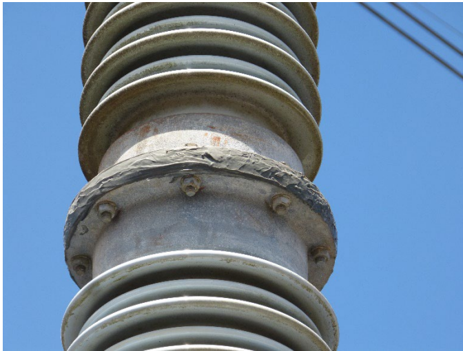
Figure 6 – 5032- Repair (Belzona) applied
