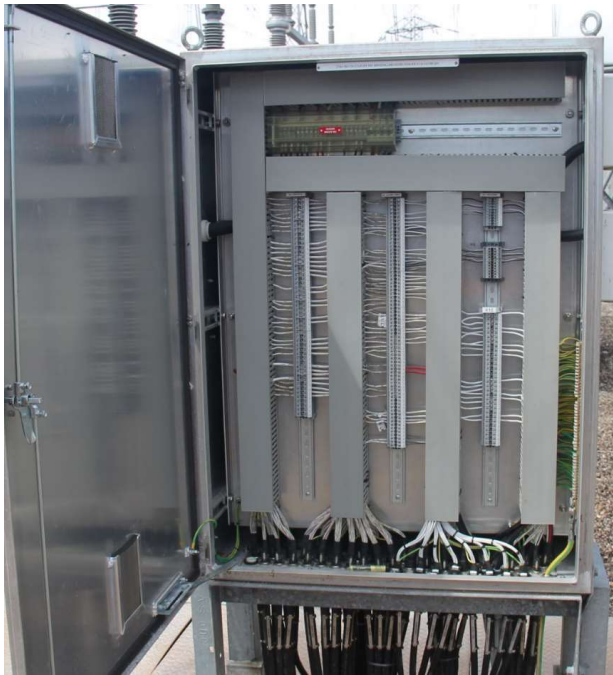
275kV Bay 4 coupler bay marshalling kiosk
