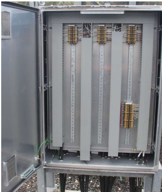
275kV Feeder 857 reactor marshalling kiosk
