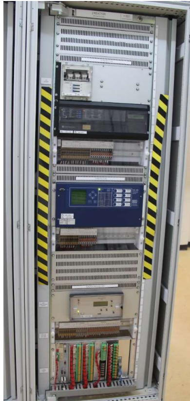
857 feeder reactor protection and control panel
