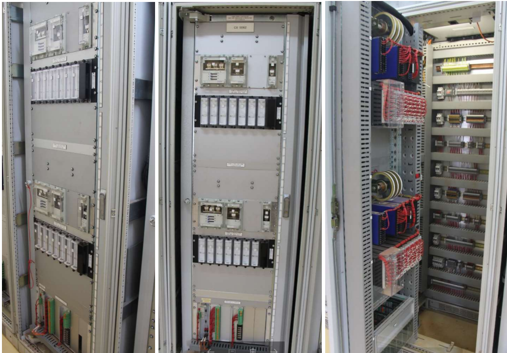
275kV 1 & 2 Bus protection and CB fail bus trip panel
