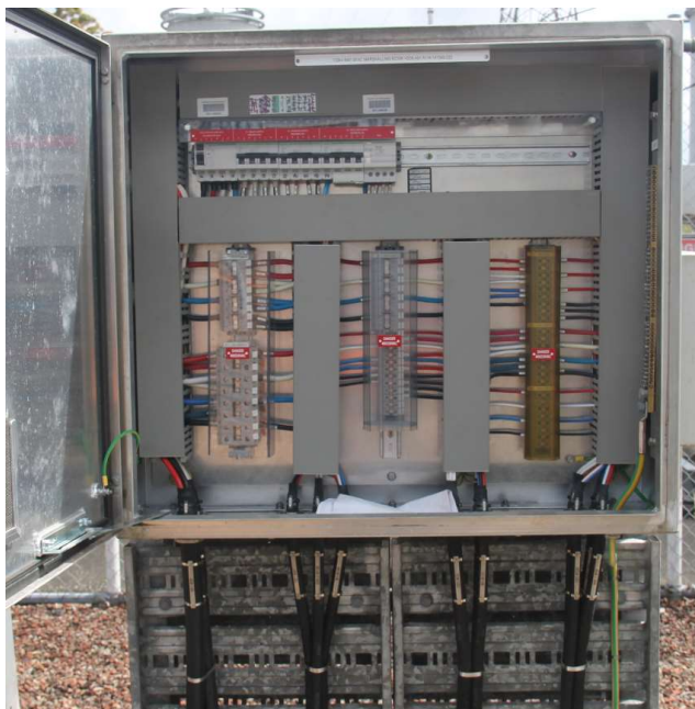
132kV Bay =D08 AC and DC marshalling kiosk
