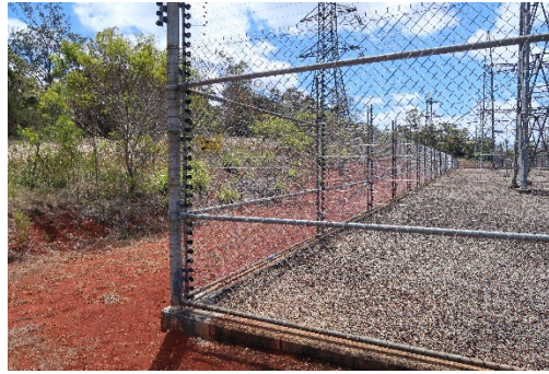
Figure 15 –Substation security fence
