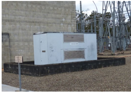
Figure 13 - 1 T station supply transformer
