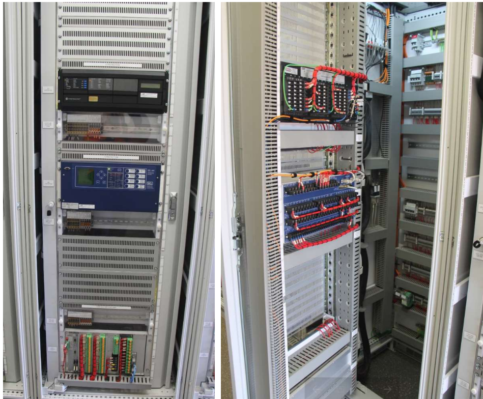
132kV Bus coupler protection and control panel
