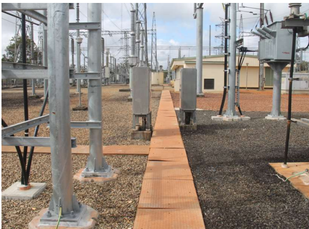
Substation trenches
