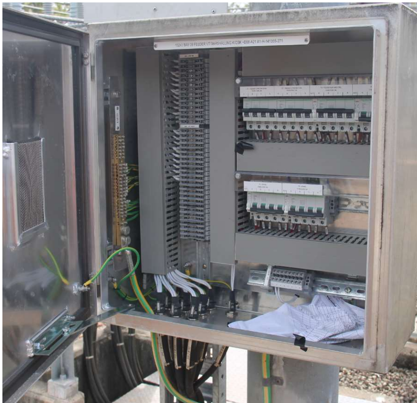
132kV Bay =D08 Feeder 7165 8VT box
