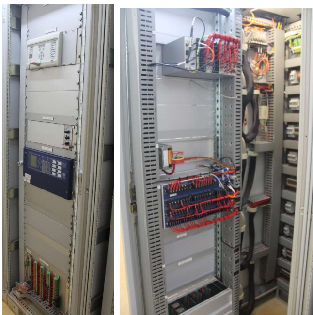
Feeder 858 protection and control panel
