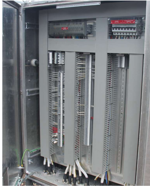
275kV Feeder 858 reactor marshalling kiosk
