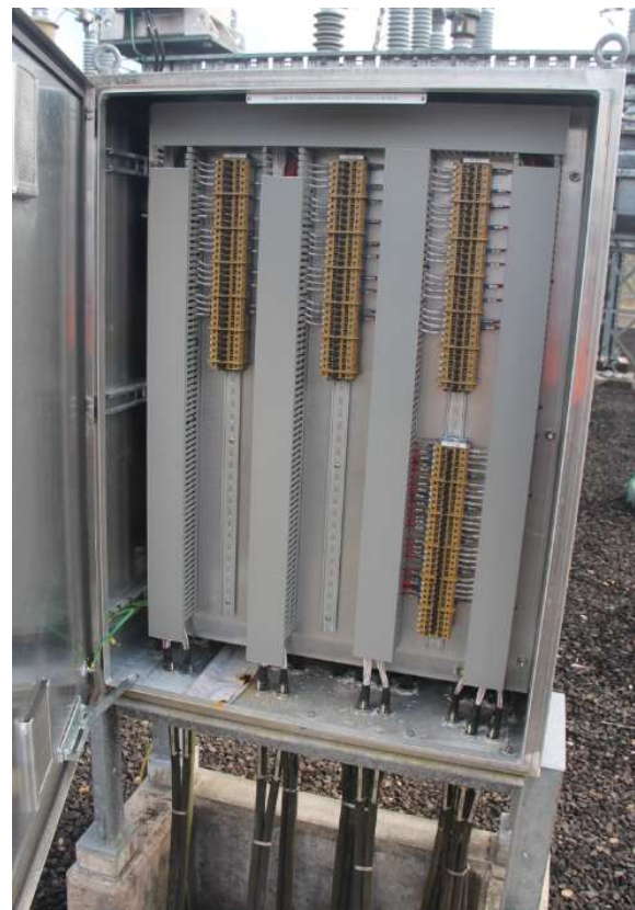
132kV Bay =D06 Feeder 7192 bay marshalling kiosk
