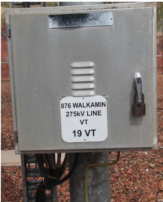
275kV feeder 876 19 and 20 VT marshalling kiosk
