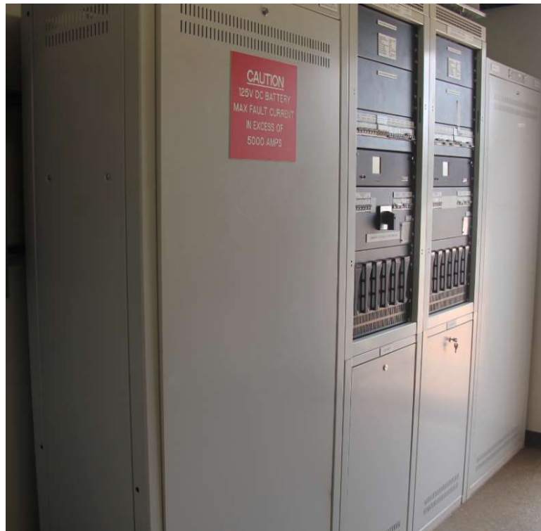
125VDC Batteries and charger in building +4
