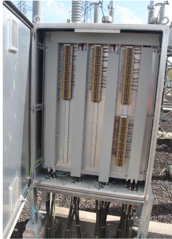
132kV Bay =D04 1 Transformer LV bay marshalling kiosk
