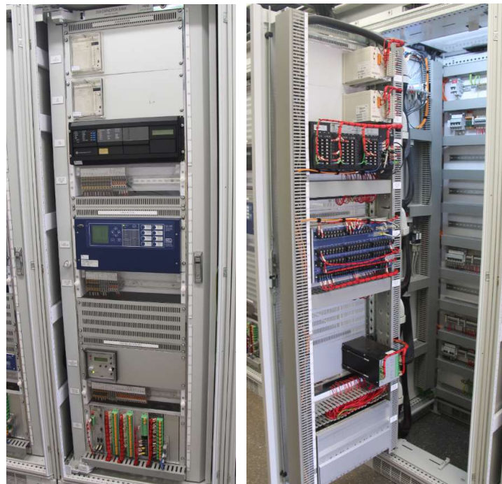
1 CAP protection and control panel
