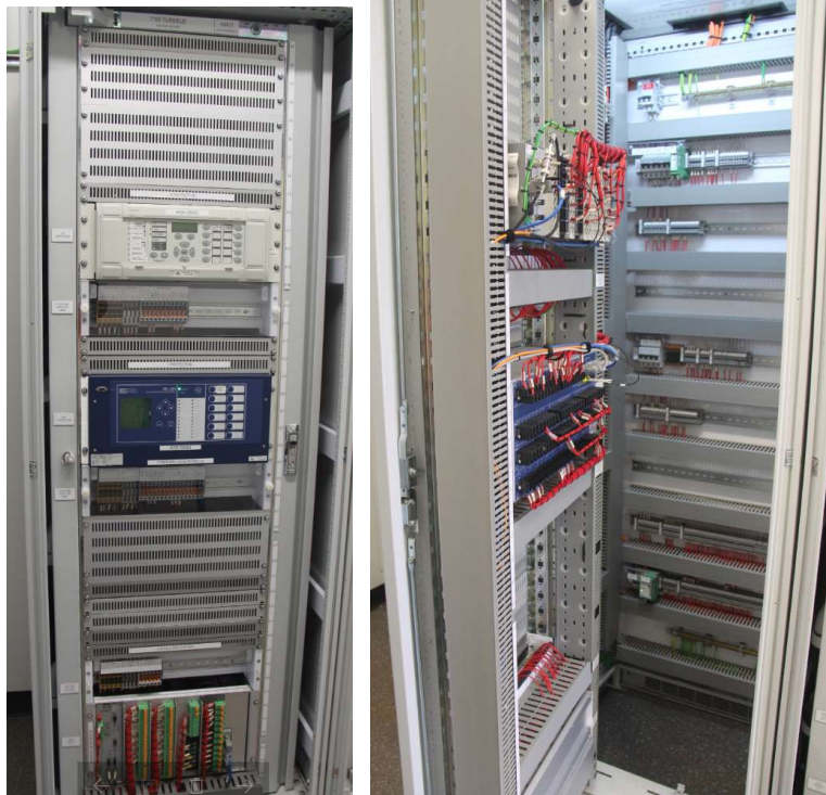
Feeder 7165 protection and control panel
