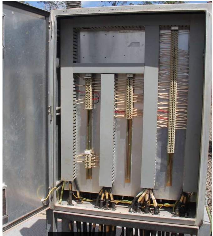
275kV Feeder 877 bay marshalling kiosk
