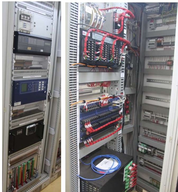
275kV Bus reactor protection and control panel
