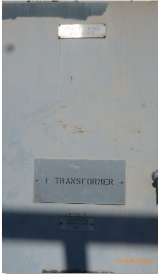
Figure 26- Minor Corrosion on Control Cubicle Door
