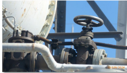
Figure 15- Oil Leak from Oil Isolation Valve
