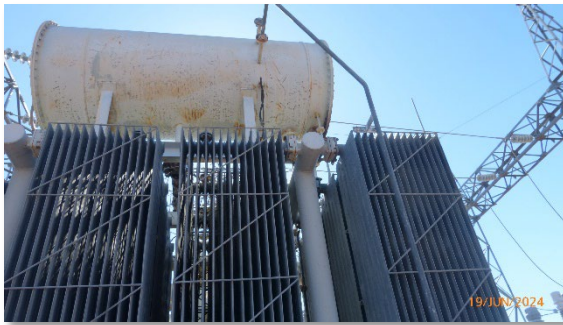
Figure 2- Conservator Tank with Visible Corrosion (June 2024)
