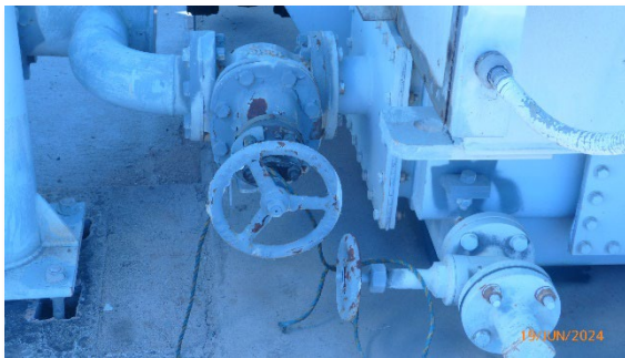
Figure 6- Grade 2 Corrosion and paint flake on Oil Valves
