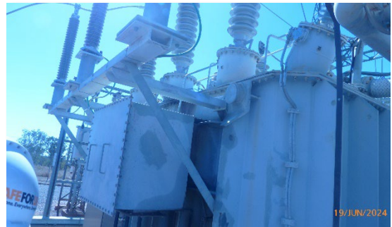
Figure 5- Touch-Up Paint Marks on Transformer
