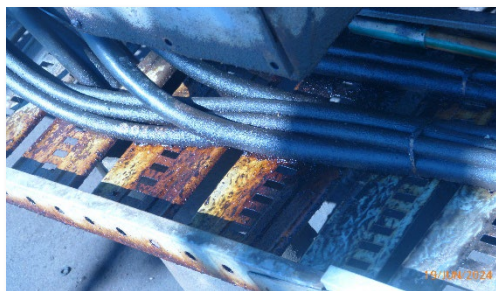
Figure 19- Oil Leak on Cable Tray Showing Corrosion
