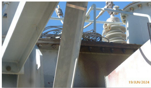
Figure 15- Oil Leak from Oil Isolation Valve
