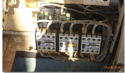
Figure 27- Oil-Contaminated Control Components
