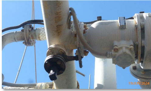
Figure 13- Oil Leak from Drain/Fill Flange
