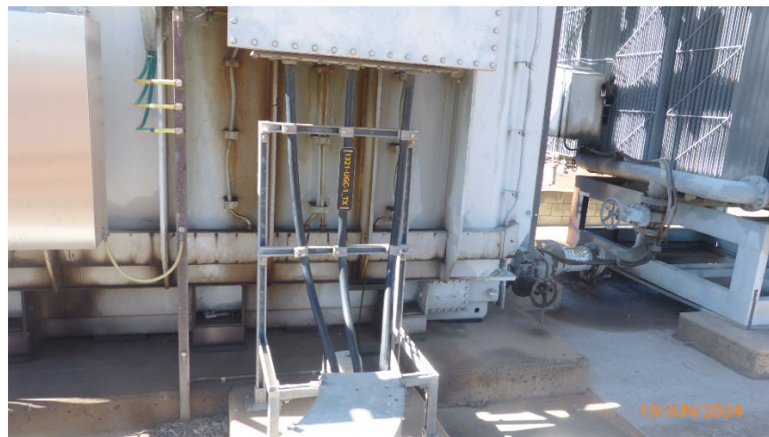
Figure 12- Oil on Transformer Surface from Active Leaks
