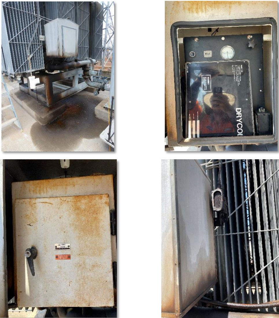
Figure 24- Drycol Breather Control Box
