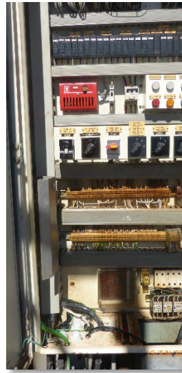
Figure 27- Oil-Contaminated Control Components
