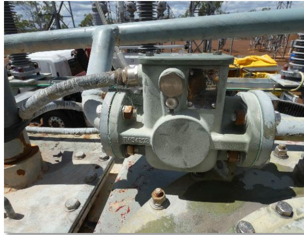
Figure 31- Corrosion on Fasteners for Oil Surge Relays and Diverter Lids
