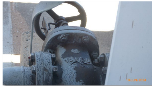
Figure 9- Corrosion and paint flake
