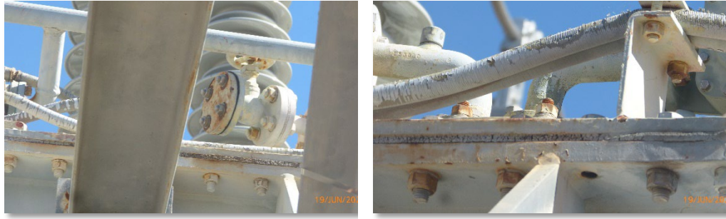
Figure 20- Flange with Significant Gasket Deformation
