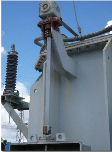
Figure 32- OLTC Drive Linkage with Minor Corrosion
