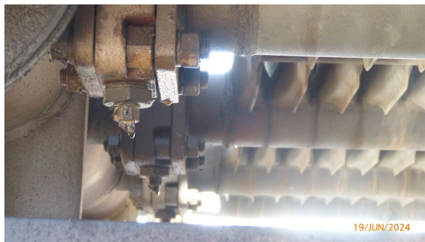
Figure 11- Oil Leak from Transformer Cooler Flanges
