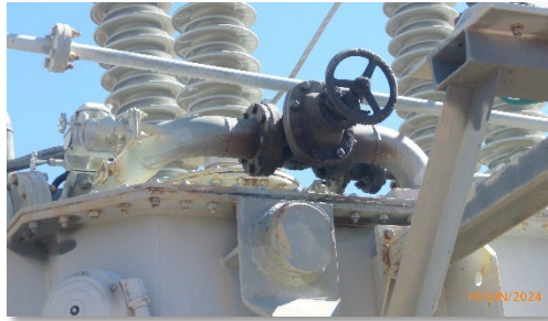
Figure 15- Oil Leak from Oil Isolation Valve
