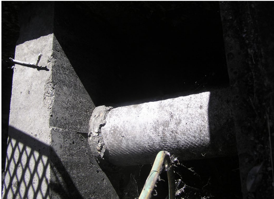
Figure 35- Flame Trap
