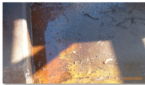
Figure 18- Oil on Transformer Bund Floor
