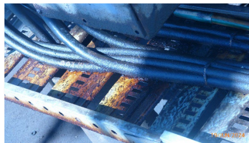
Figure 19- Oil Leak on Cable Tray Showing Corrosion
