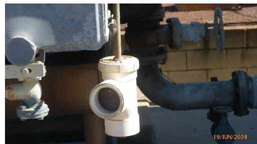
Figure 22- OLTC Breather with Ergon Retrofit PVC Solution
