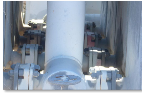
Figure 14- Oil Leak from Oil Cooler Bank Receiver Flanges
