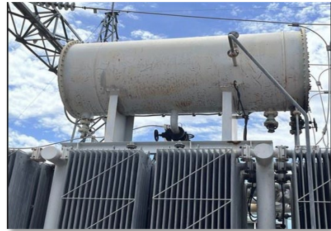
Figure 3- Conservator Tank Prior to Painting (2023)
