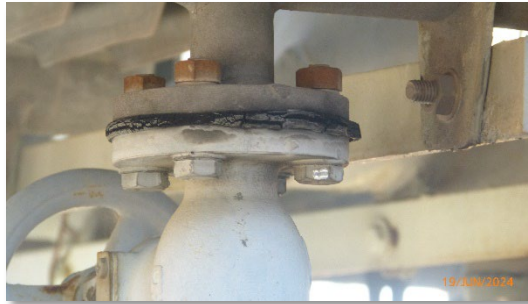
Figure 21- Flange Gasket Deformed and Deteriorated
