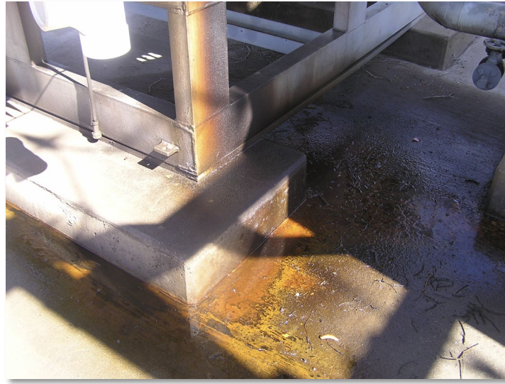
Figure 34- Apron Crack
