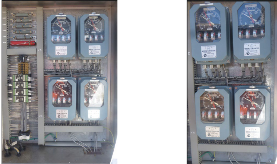
Figure 25- WTI and OTI (Installed in Shared Control Cubicle)
