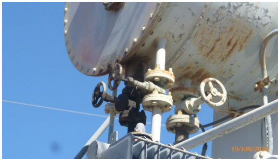
Figure 4- Close-up of Conservator Tank Corrosion
