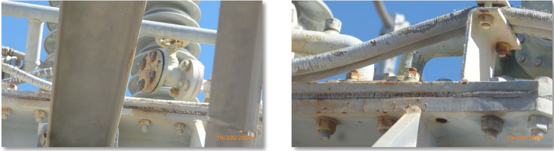
Figure 10- Corrosion on Transformer Components (Grades 1 to 3)
