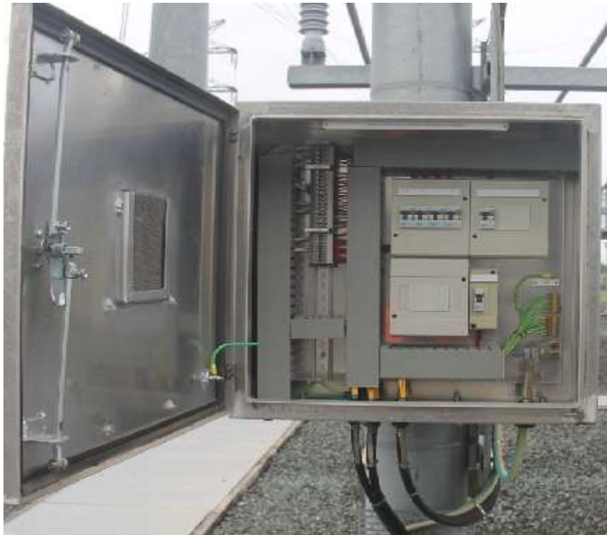
7 Transformer 110kV LV VT box, +D60-A14
