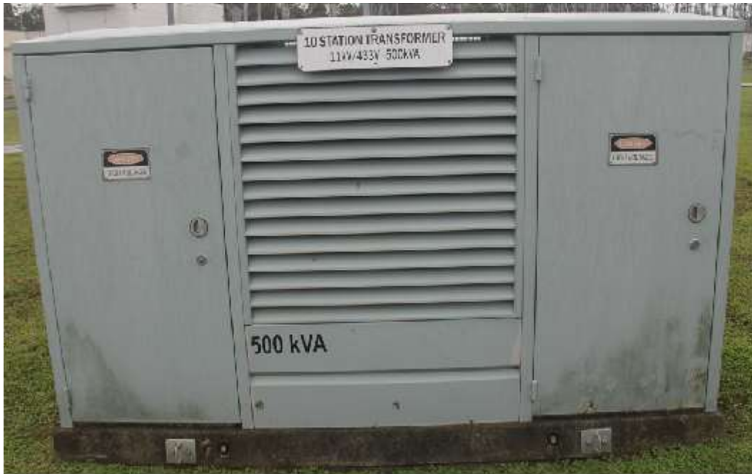
Pad-mount Station Services transformer
