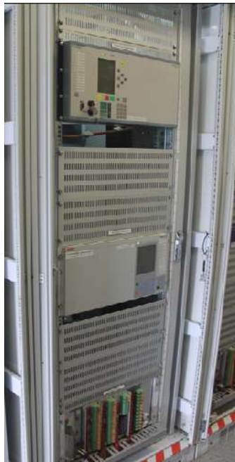
Typical Protection/control panel in Building +4 (Bay 55 Fdr panel)
