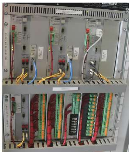
NSC Link and Common RTUs in Buildings +2, +4 and +7 respectively
