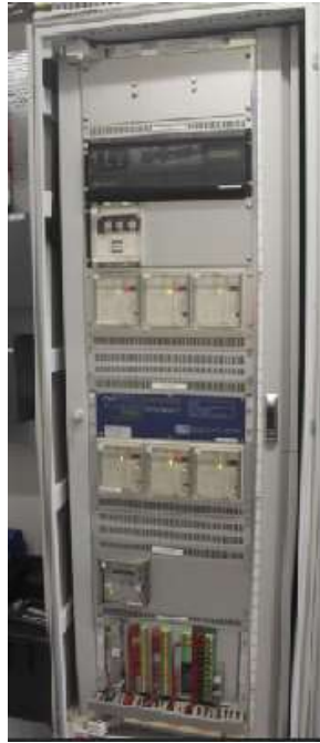
Typical Protection/control panel in Building +6 (9 Cap)
