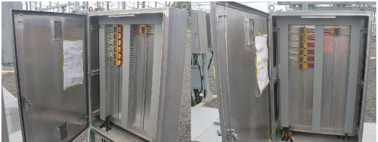
110kV 4 Bus CT marshalling kiosk, +KD4-A1
