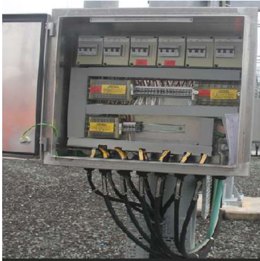
110kV Feeder 746 VT box
