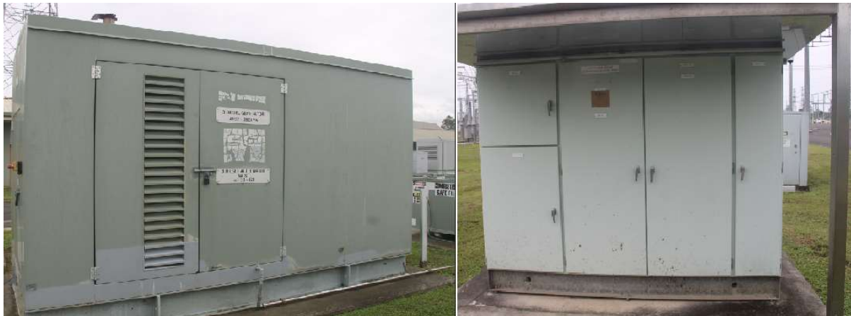
Diesel Generator and AC change-over board with a weather cover
