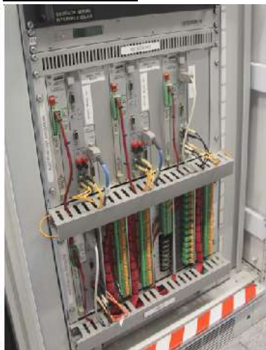
NSC Link and Common RTUs in Buildings +2, +4 and +7 respectively
