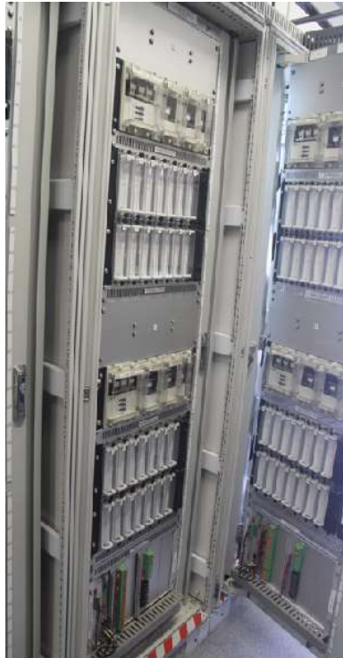
Typical Protection/control panel in Building +5 (adjacent Bus Zone panels)
