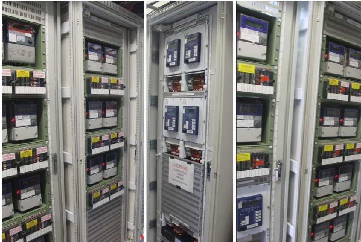
Revenue metering panel in Buildings +4, +6 and +7
