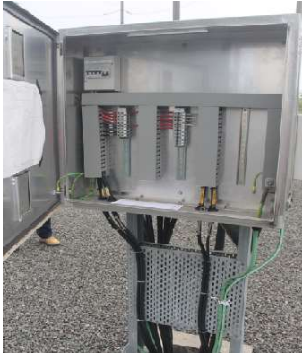
110kV bay =D73 DC marshalling kiosk, +D73 -A92
