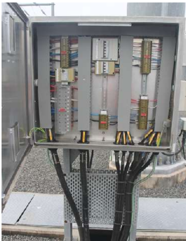
110kV bay =D73 AC marshalling kiosk, +D73-A91
