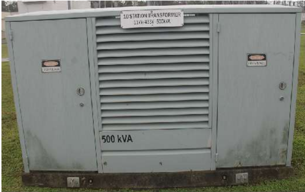
Pad-mount Station Services transformer
