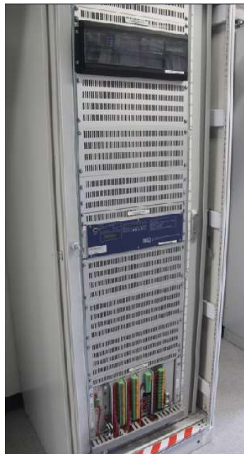
Typical Protection/control panel in Building +7 (Bay 33 4T LV panel)
