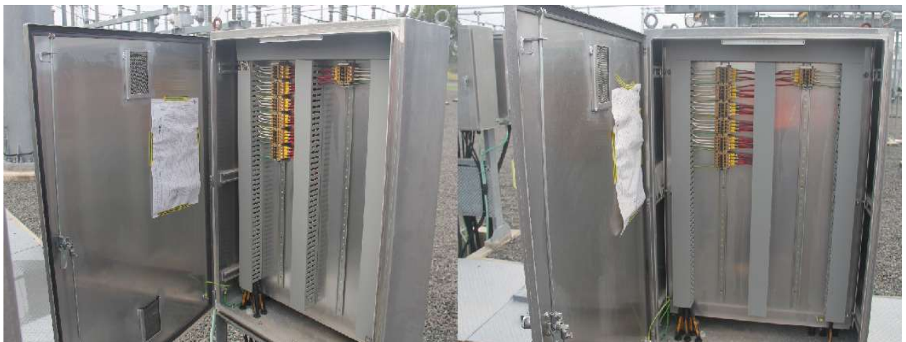
110kV 4 Bus CT marshalling kiosk, +KD4-A1
