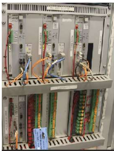
NSC Link and Common RTUs in Buildings +2, +4 and +7 respectively
