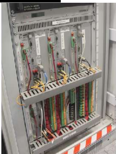
NSC Link and Common RTUs in Buildings +2, +4 and +7 respectively
