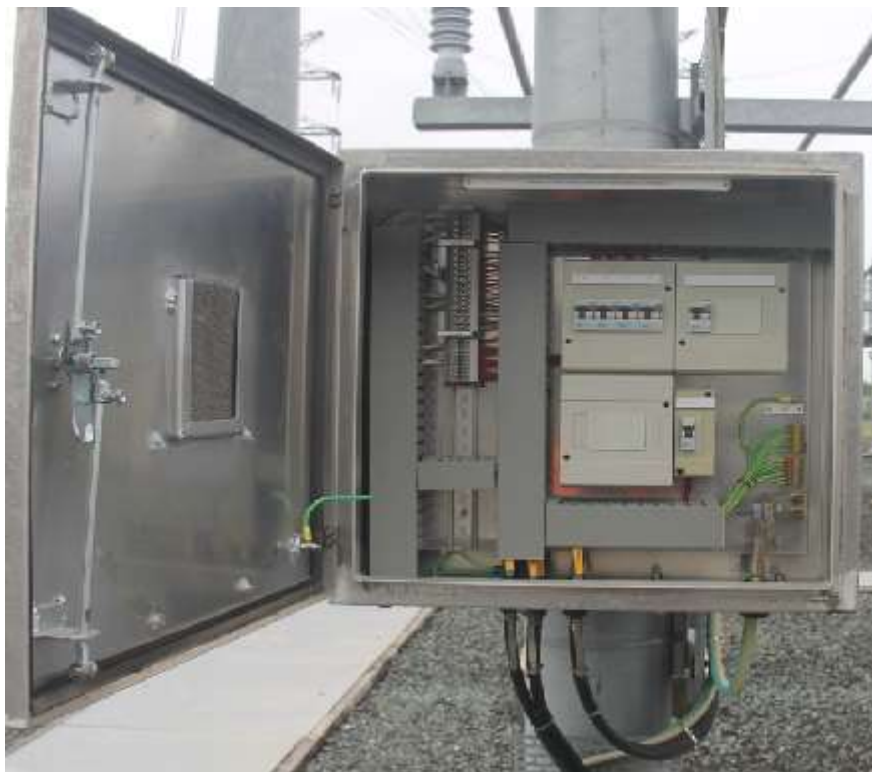
7 Transformer 110kV LV VT box, +D60-A14
