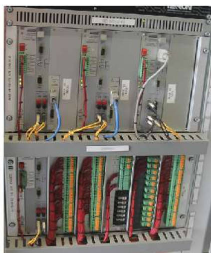
NSC Link and Common RTUs in Buildings +2, +4 and +7 respectively
