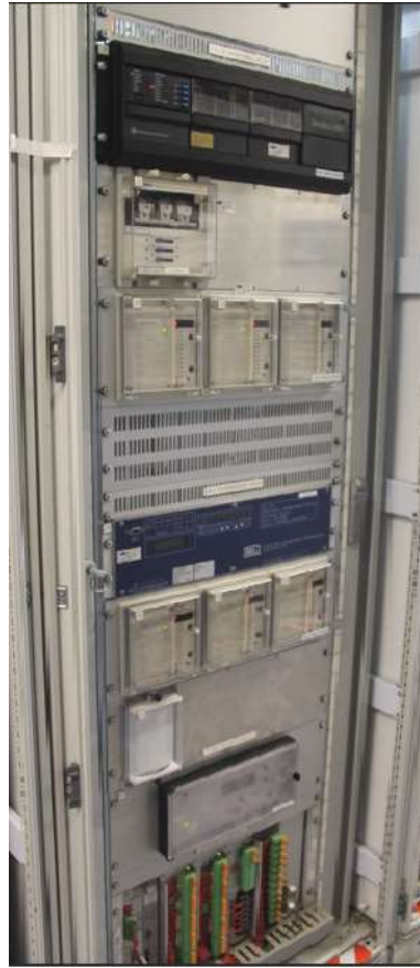
Typical Protection/control panel in Building +2 (3 Cap)
