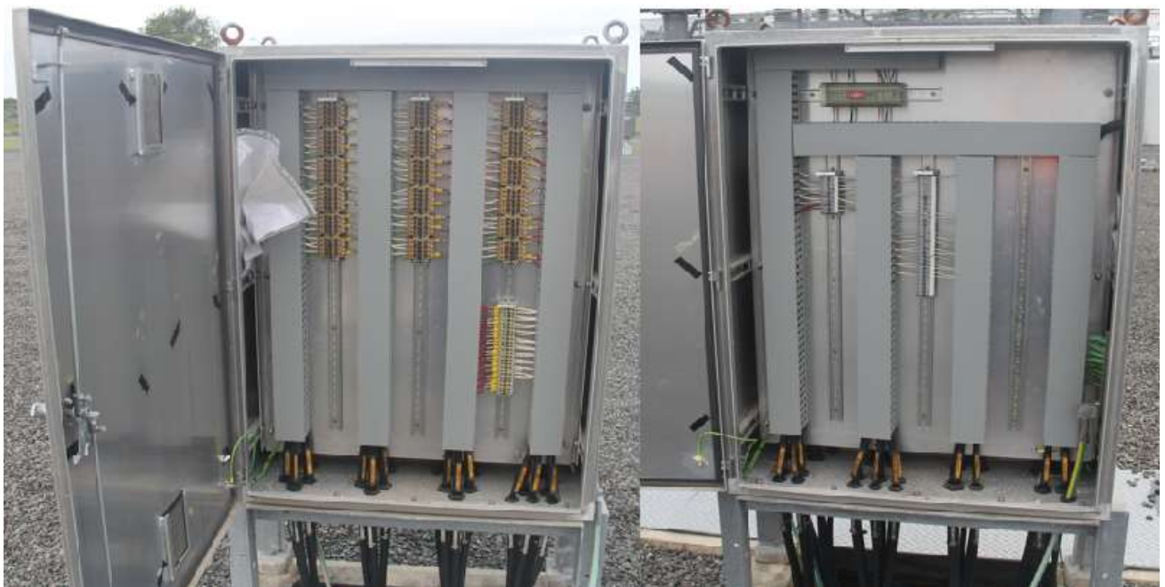
110kV T4 LV bay marshalling kiosk, +D33-A10
