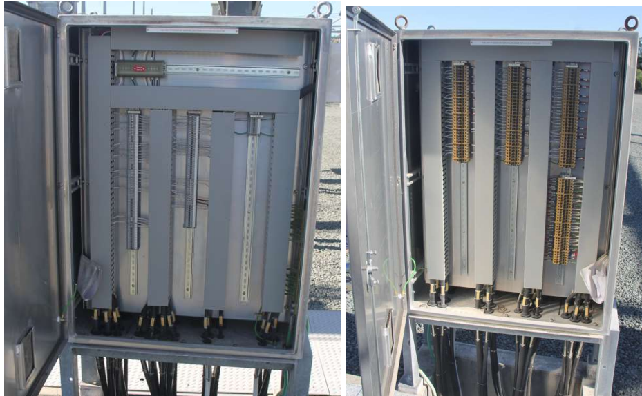
110kV Bay 82 Feeder 7345 Bay marshalling kiosk +D82-A10
