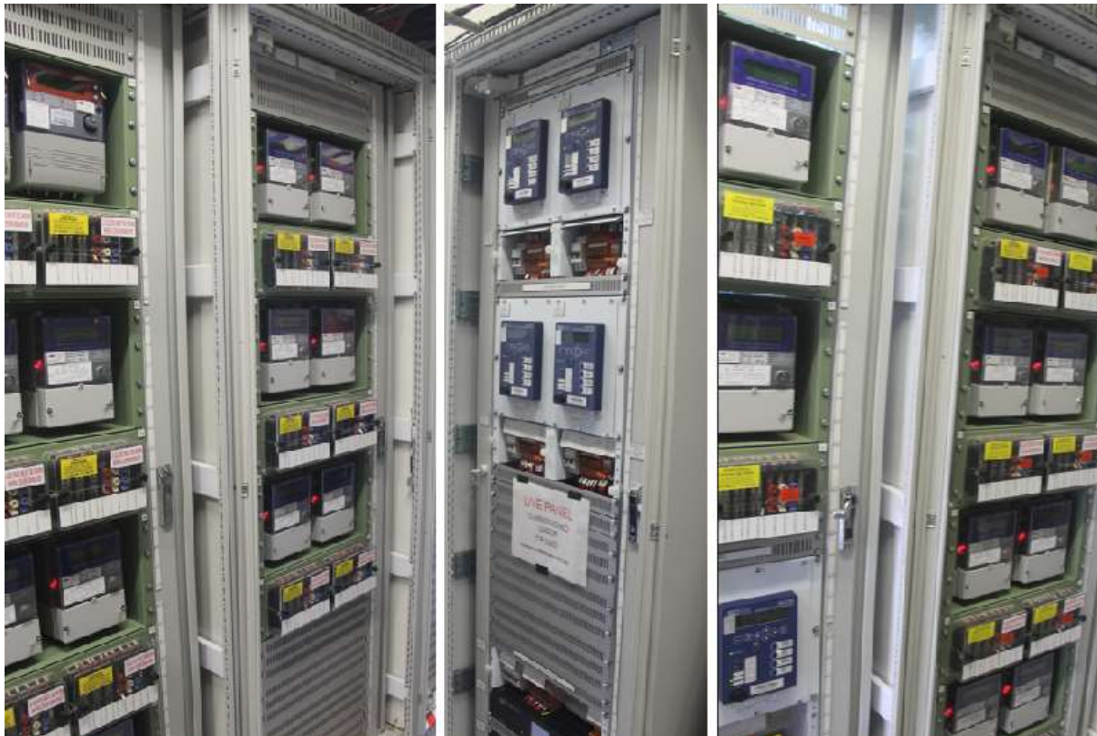
Revenue metering panel in Buildings +4, +6 and +7
