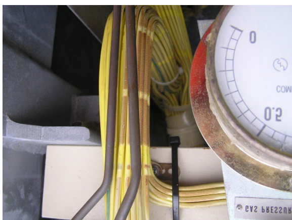
Figure 8- UV damage to internal wiring and the operation counter
