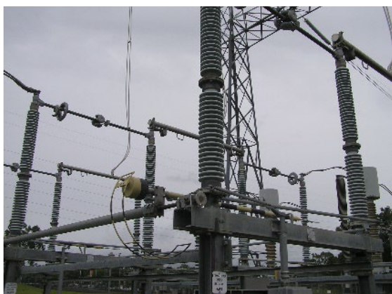
Figure 9- Visible corrosion on disconnector
