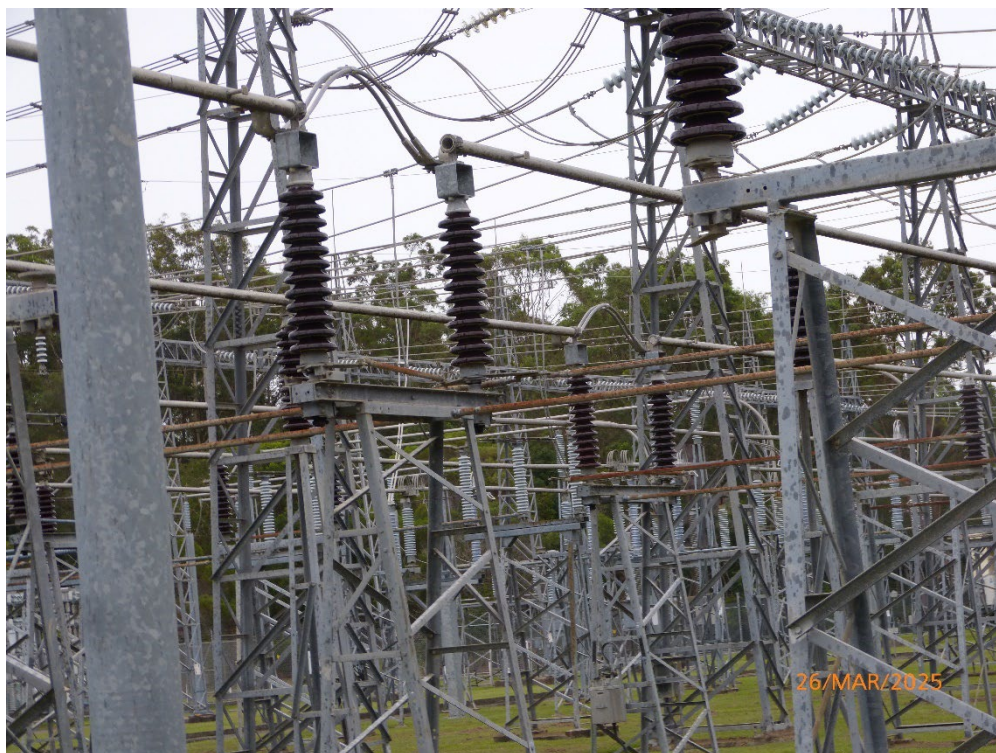
Figure 21-Bridged Disconnectors
