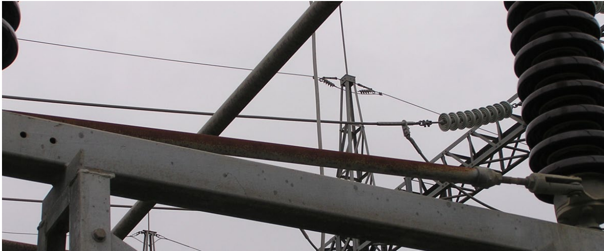
Figure 20- Corrosion on disconnector
