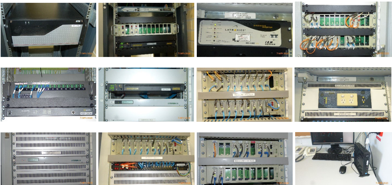
Figure 12 – Molendinar Substation Typical OpsWAN Equipment
