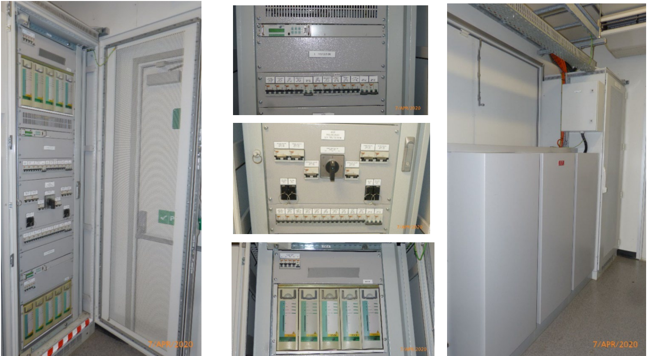
(Buildings +7 – Chargers, Monitors, DC Distribution 2006, Batteries 2006)
