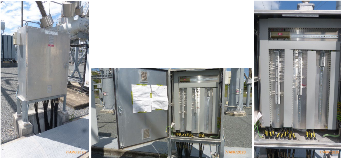
(a) 12 TFMR Deadtank CB Marshalling Kiosk (+D26-A10)
