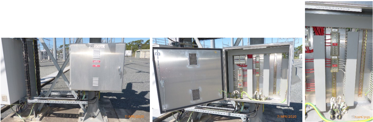
(e) CB79172 (F917 Southport) AC (+D13 A91) and DC (+D13 A92) Marshalling Kiosks
