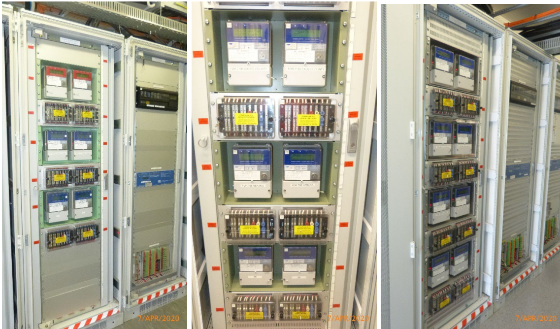
Figure 9 – Molendinar substation typical revenue metering panels
