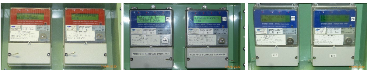
Figure 10 – Molendinar substation typical revenue meters
