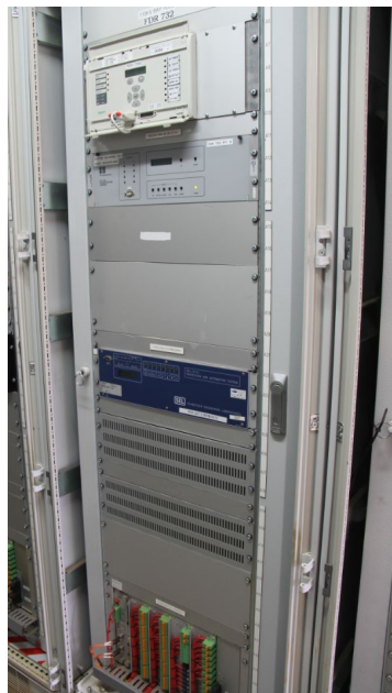
=D5.2 Feeder 732 protection and control panel
