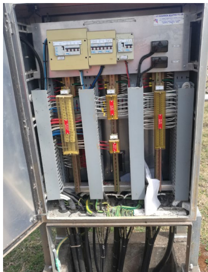
=D12.1 Feeder 736 marshalling kiosk
