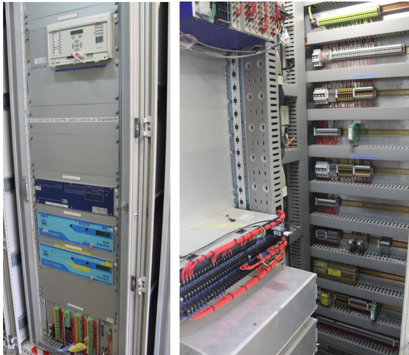
=D14.3 Feeder 735 protection and control panel
