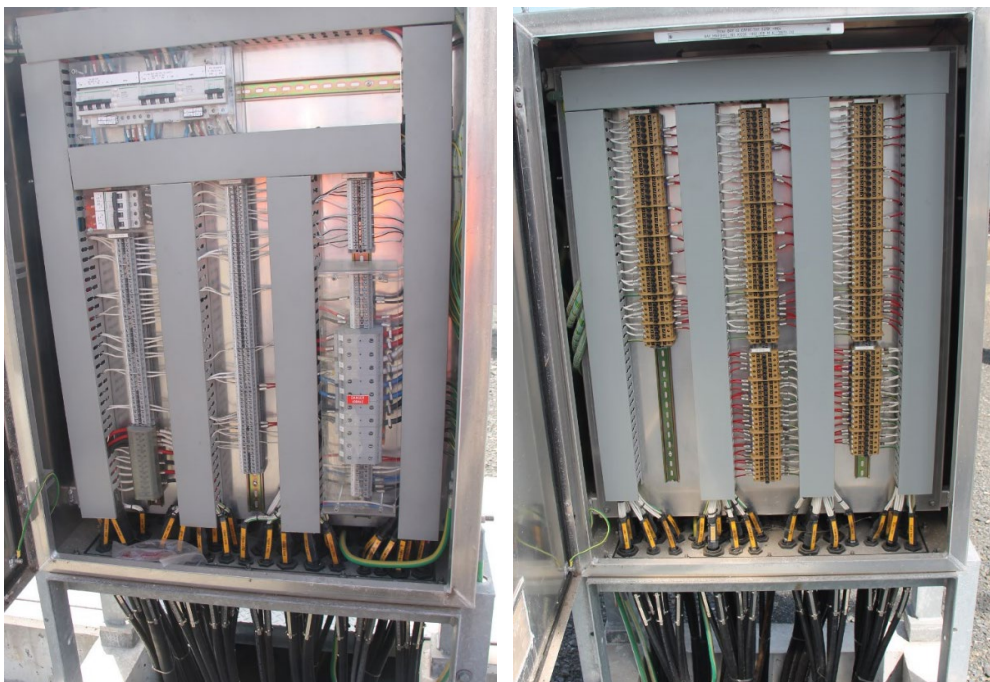
=B02 330kV Capacitor 4 bay marshalling kiosk
