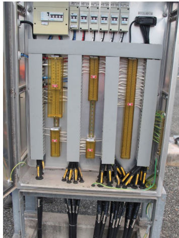
=C2 275kV Coupler 502 marshalling kiosk
