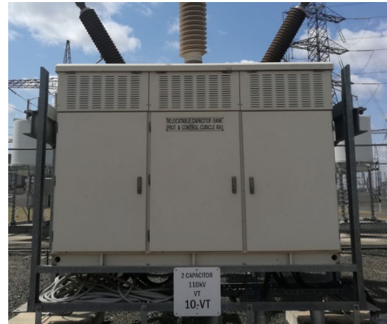
1 and 2 CAP protection and control panel
