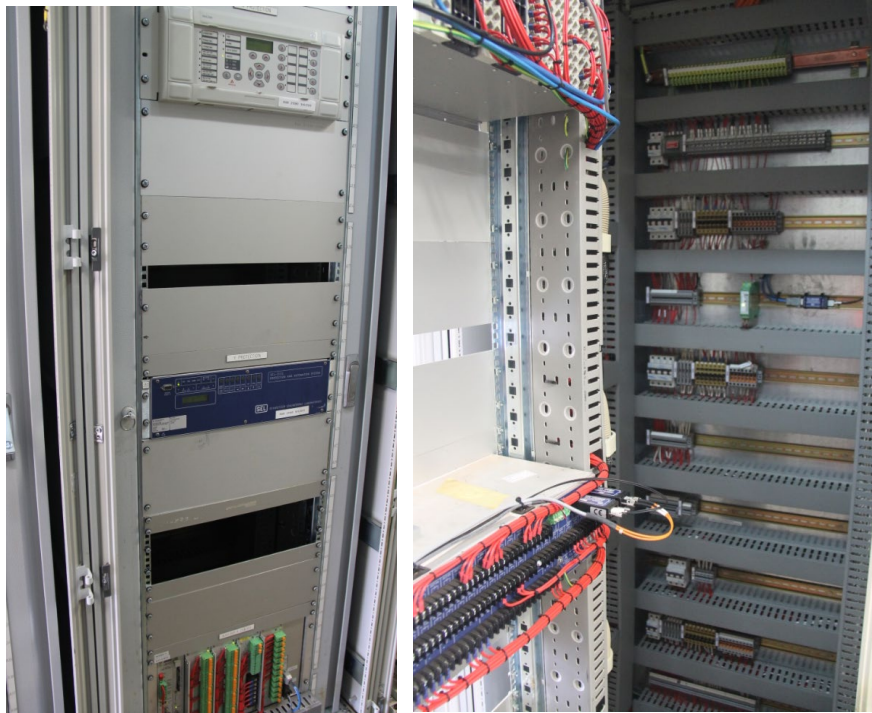
=D12.3 Feeder 7348 protection and control panel
