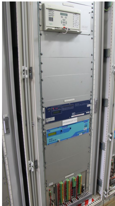
=D12.1 Feeder 736 protection and control panel
