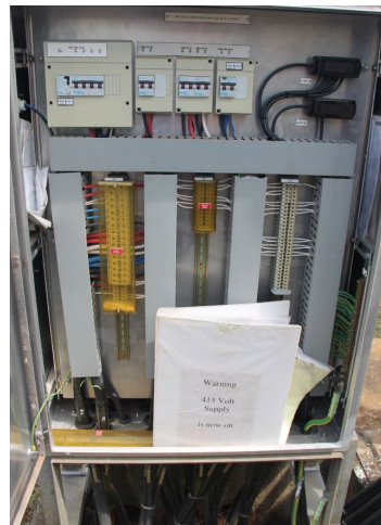
=D0.0 Bus 2-3 coupler marshalling kiosk
