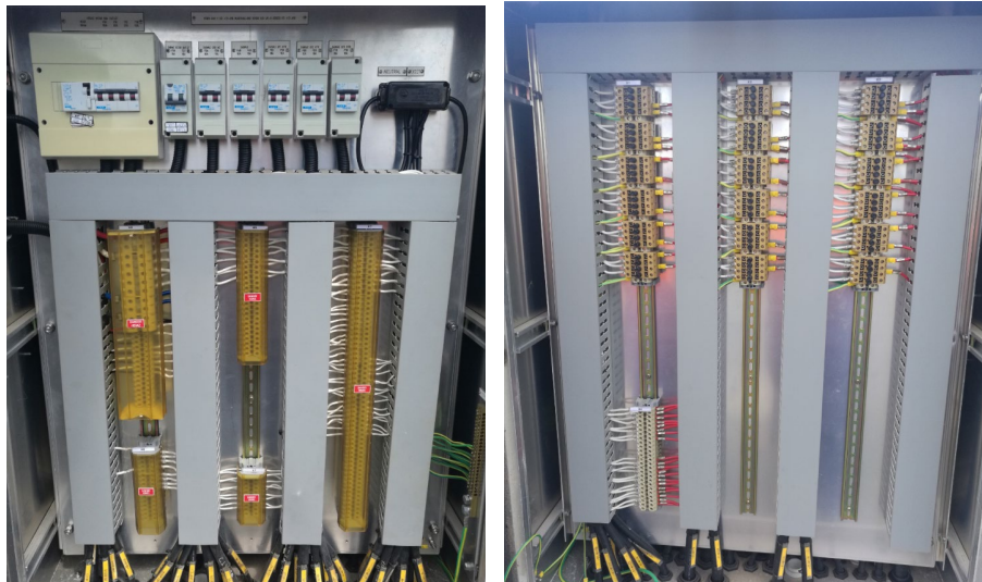
=C1.1 275kV Transformer 3 CB marshalling kiosk
