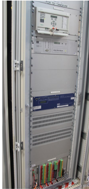
=D6.3 Feeder 731 protection and control panel
