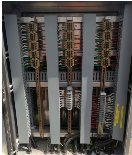
=D11.3 Transformer 1 marshalling kiosk
