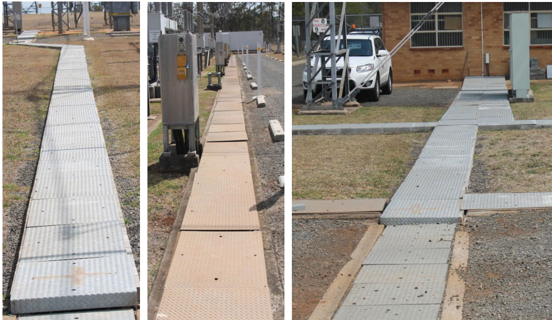
Substation trenches
