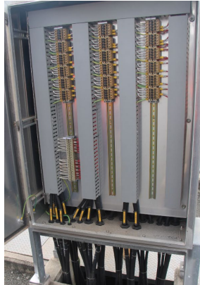
=C2 275kV Transformer 1 CB marshalling kiosk (+C2-A20)
