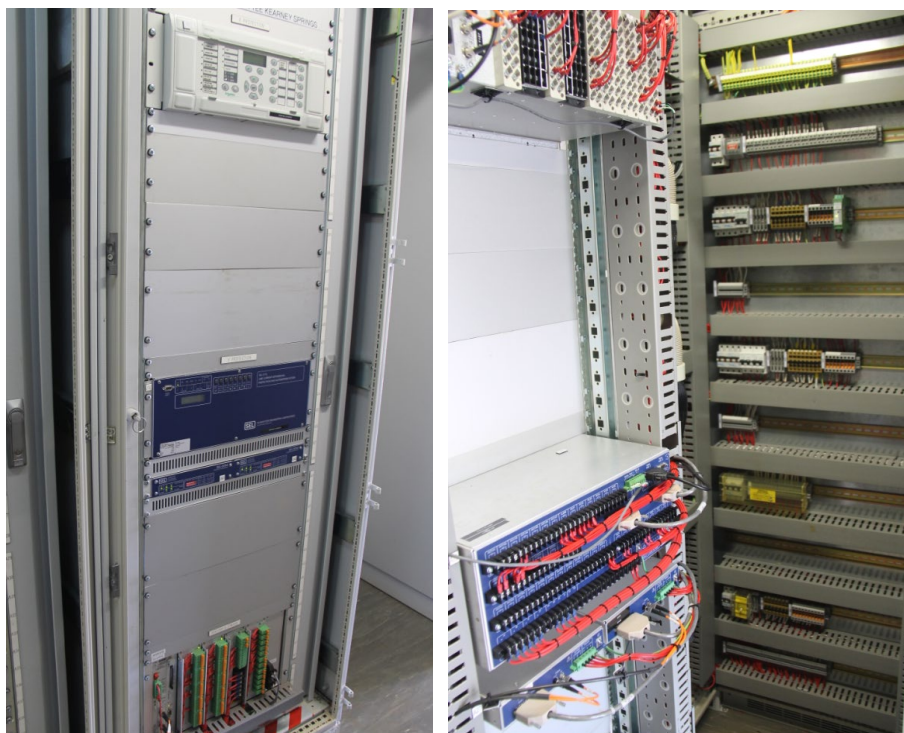
=D1.3 Feeder 730 protection and control panel
