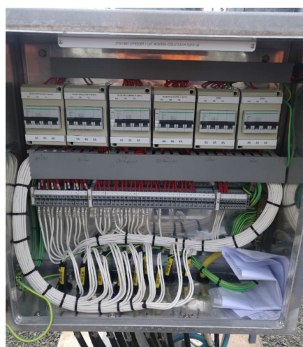
=C3.1 Feeder 8848 CVT box (=C03-A13)
