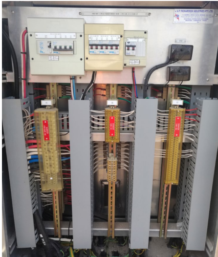
=D11.3 Transformer 1 marshalling kiosk
