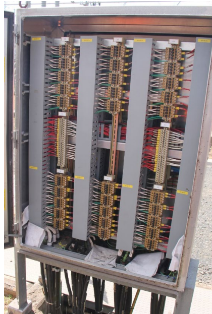
=D9 110kV 1-2 Bus coupler marshalling kiosk
