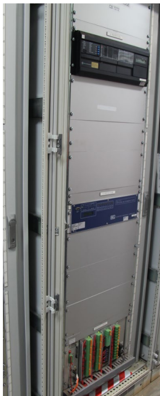
=D3.2 Feeder 727 protection and control panel
