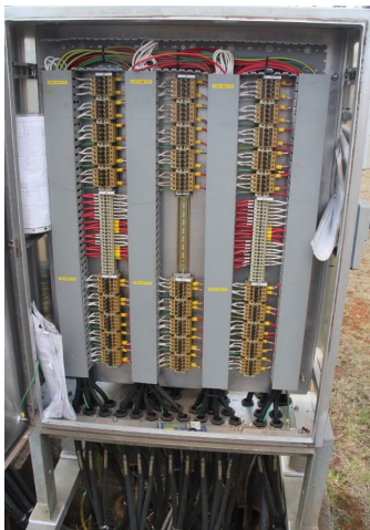
=D0.0 Bus 2-3 coupler marshalling kiosk
