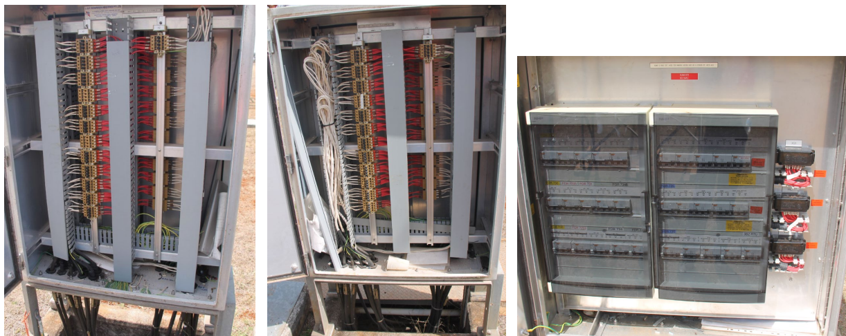
110kV 3 Bus zone marshalling kiosk and VT box
