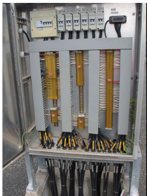
=C2 275kV Transformer 1 CB marshalling kiosk (+C2-A20)
