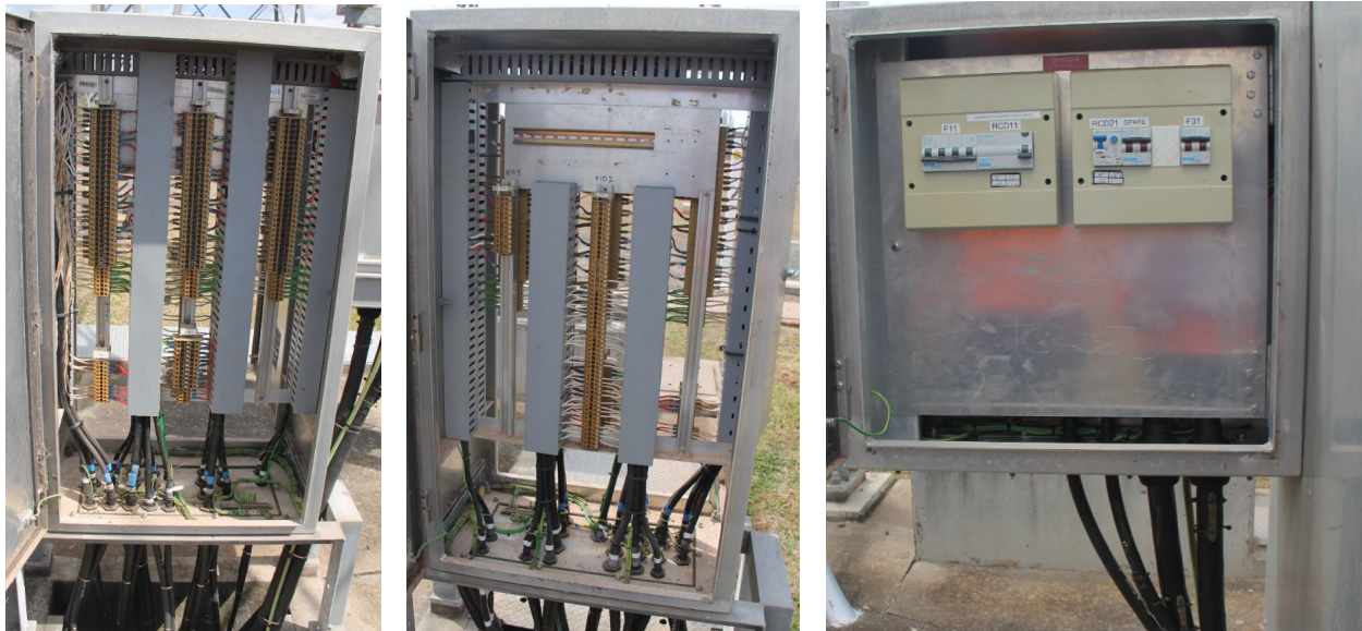
=D6 Feeder 731 marshalling kiosk
