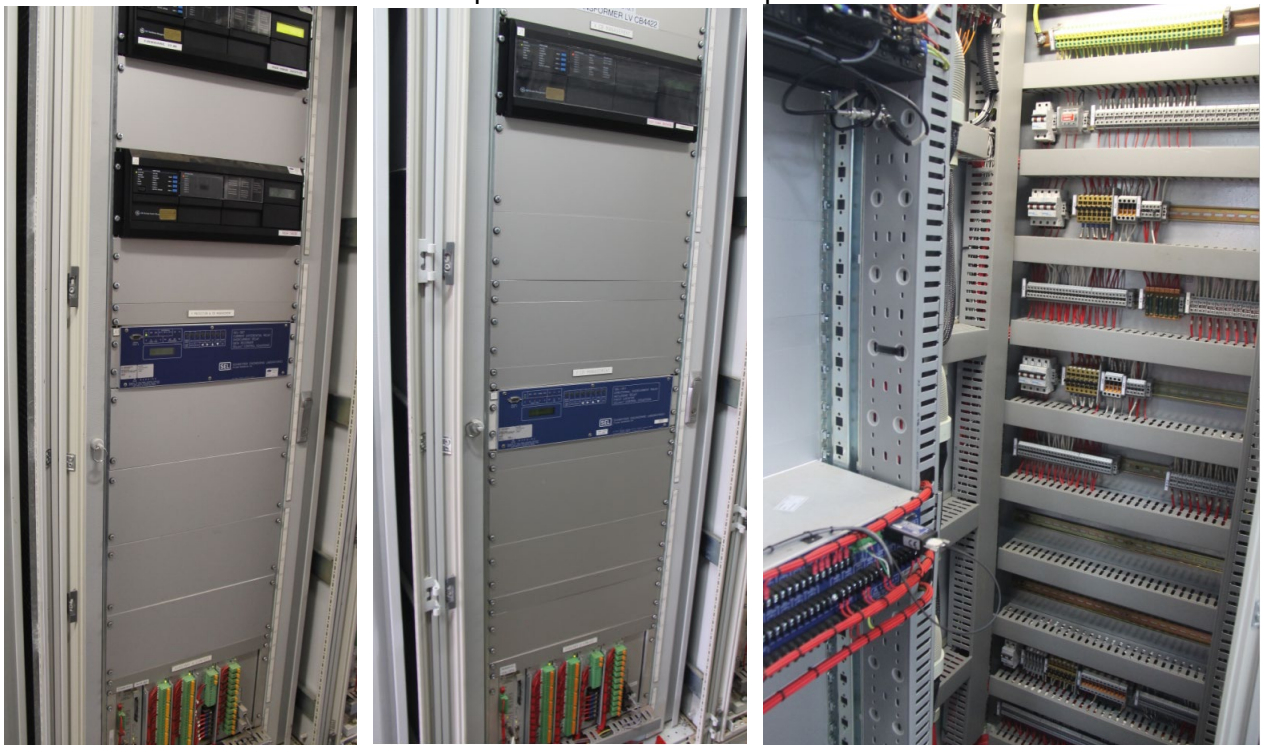
2T protection and control panel
