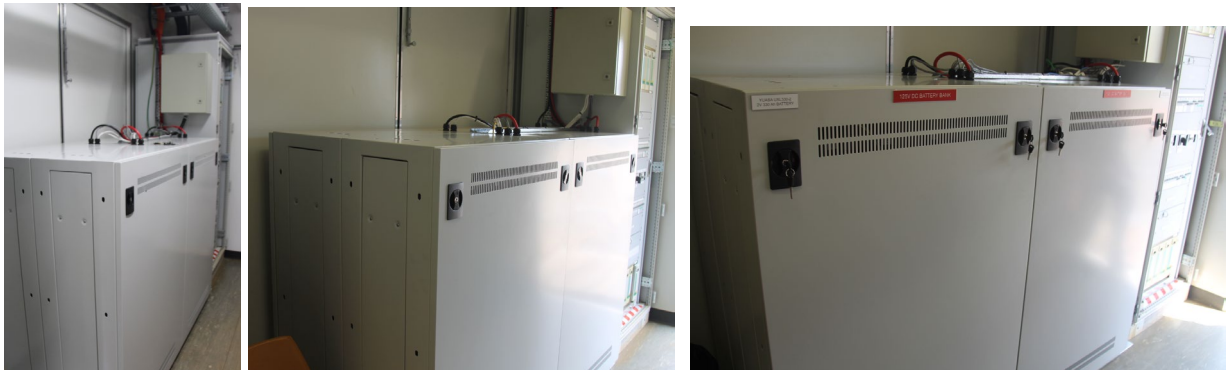
125VDC Batteries and charger in Building +6, +7 and +8
