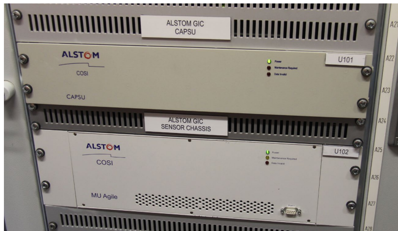
Transformer HV GIC monitoring system
