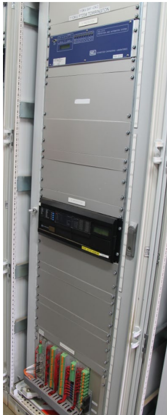
=D4.2 Feeder 7234 protection and control panel
