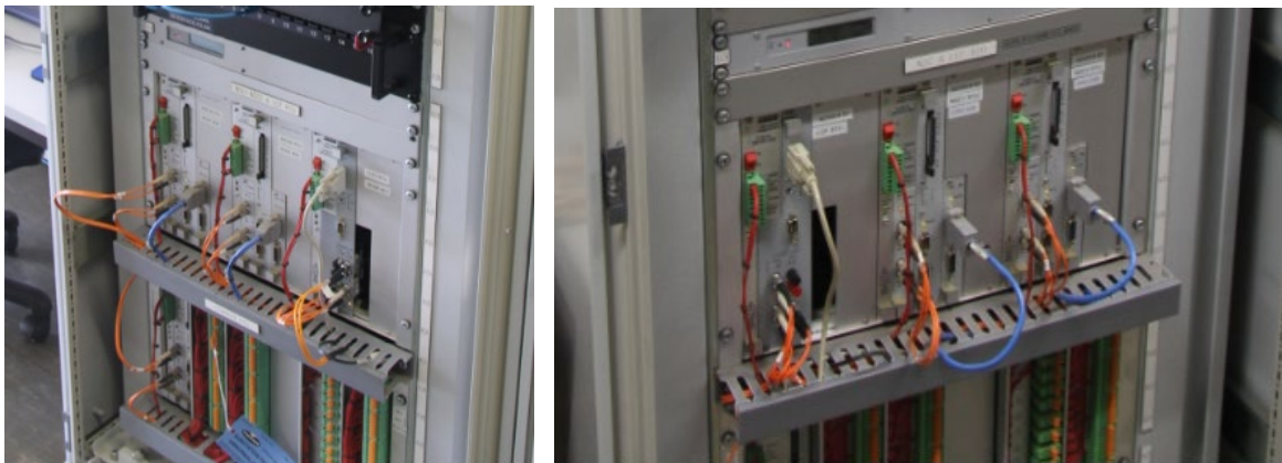
LCF and SCADA RTUs (330/275kV and 110kV)
