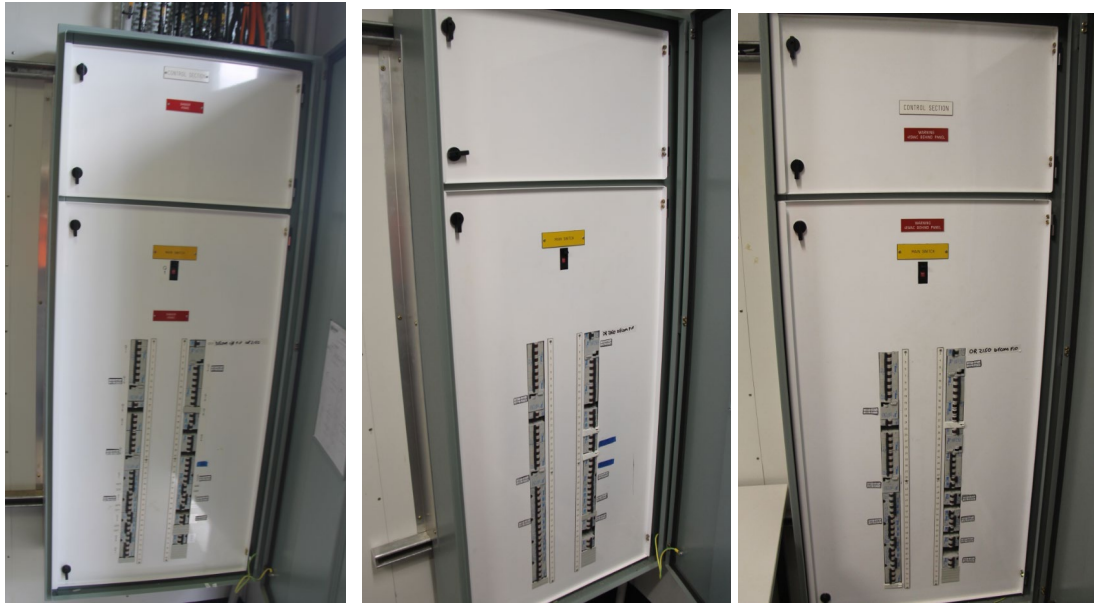
AC distribution board within building +6, +7 and +8
