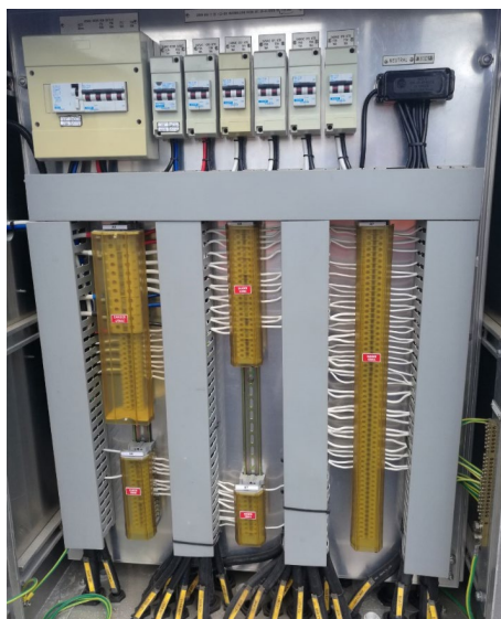
=C2.1 275kV Feeder 831 CB marshalling kiosk
