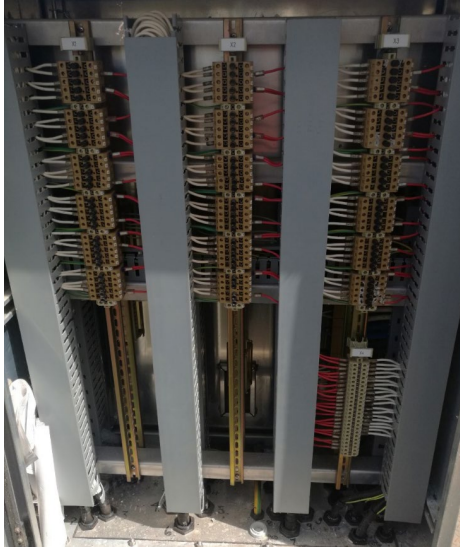
=D13.1 Spare 5 bay marshalling kiosk
