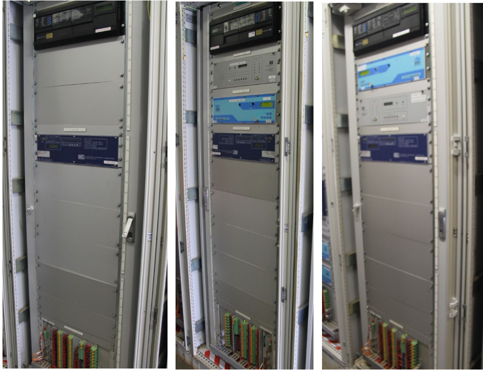
275kV bus coupler 501, 502 and 503 protection and control panel
