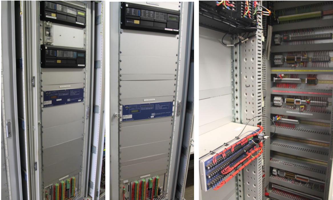
1T protection and control panel
