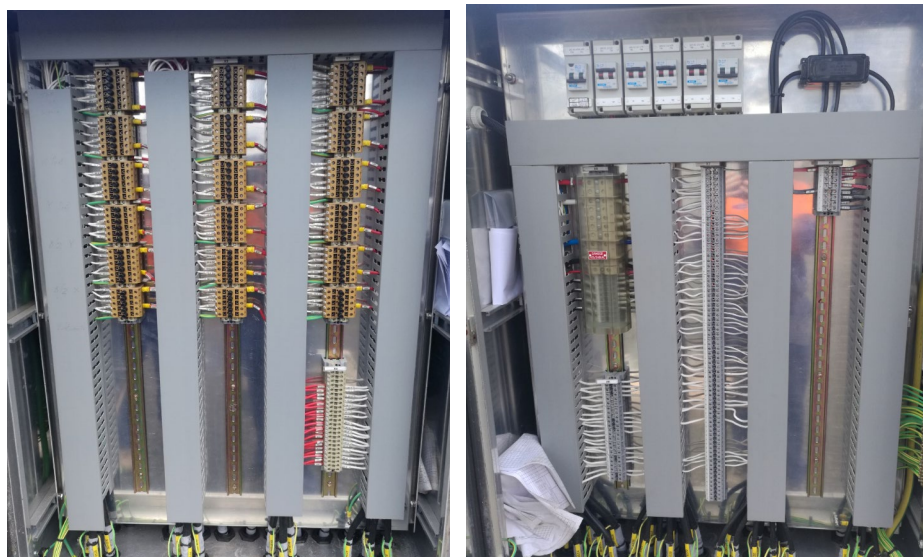
=C3.1 Feeder 8848 CB marshalling kiosk
