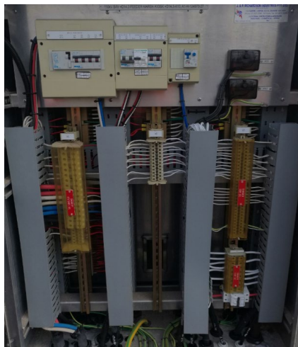
=D14.3 Feeder 735 marshalling kiosk
