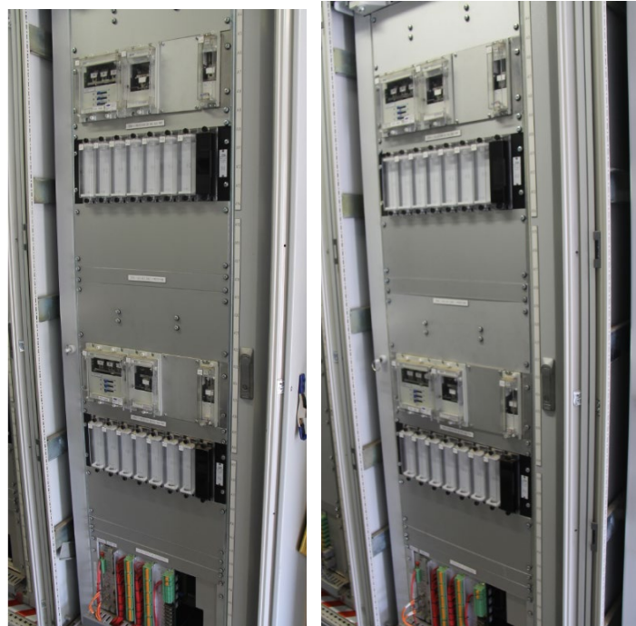
275kV 1 & 2 Bus zone and CB fail panels
