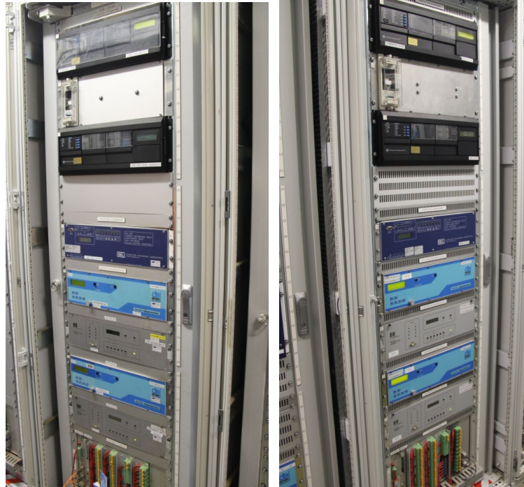
4 and 5 Transformer 275kV protection and control panel
