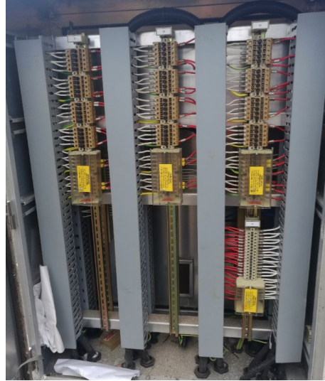
=D11.1 Feeder 733 marshalling kiosk
