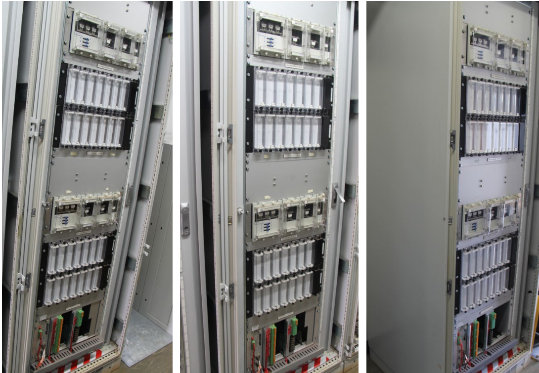
110kV Bus zone protection and control panels
