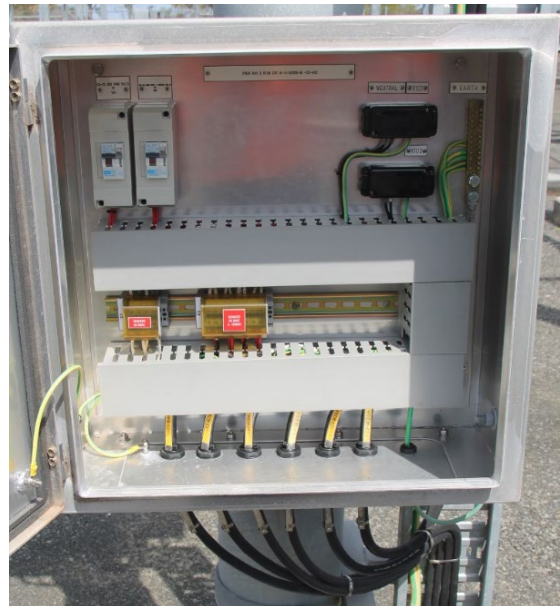
=C3 4 Transformer 275kV VT box
