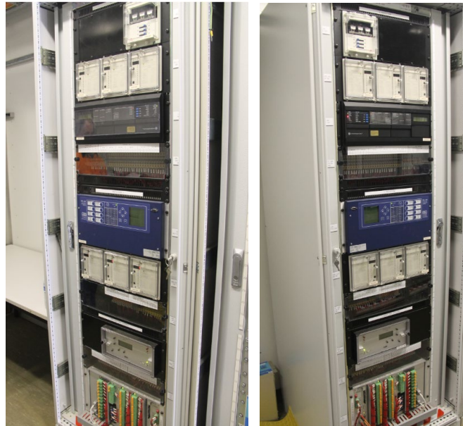
330kV 3 & 4 CAP protection and control panel
