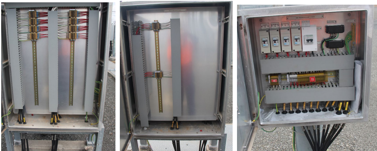
275kV 2 Bus marshalling kiosk and VT box
