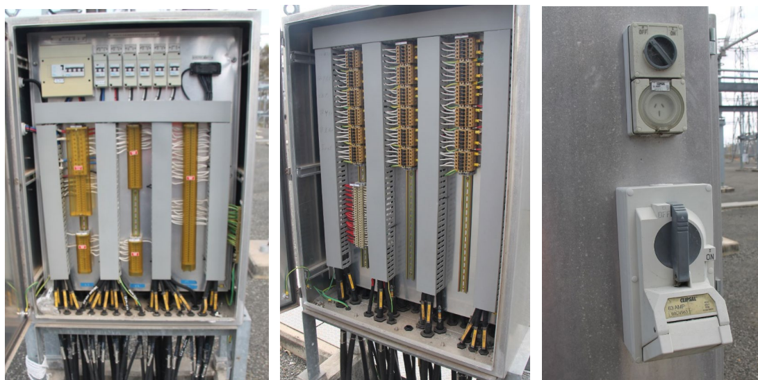
=C3 275kV coupler 503 CB marshalling kiosk
