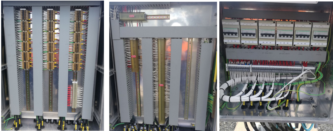
=C04.1 Feeder 8849 marshalling kiosk and CVT box
