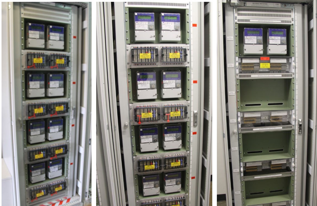
Metering panel (+6A9, +7A8 and 7A9)
