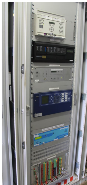
Feeder 831 protection and control panel
