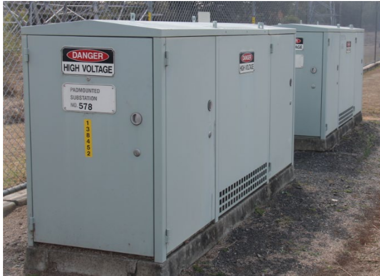
415VAC station transformer
