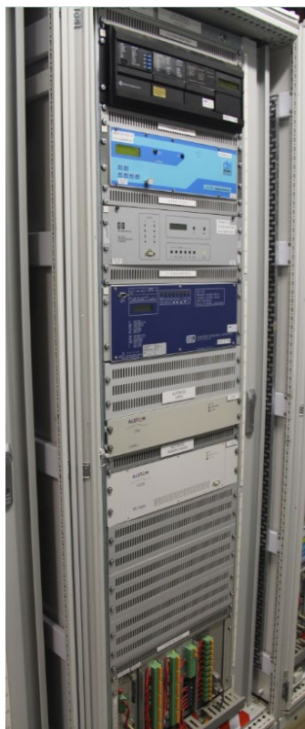
275kV bus coupler 504 protection and control panel
