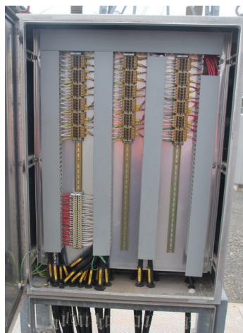
=C2 275kV Coupler 502 marshalling kiosk
