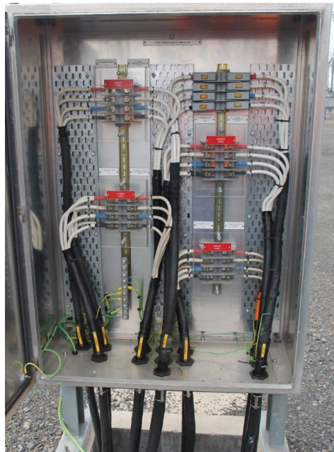
AC supply termination cubicle
