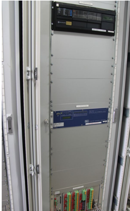
=D11.1 Feeder 733 protection and control panel
