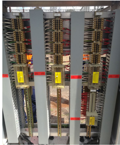
=D12.3 Feeder 7348 marshalling kiosk
