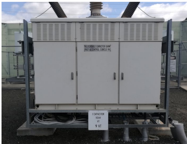
1 and 2 CAP protection and control panel
