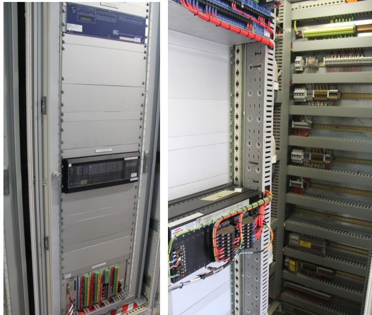
=D2.3 Feeder 7233 protection and control panel
