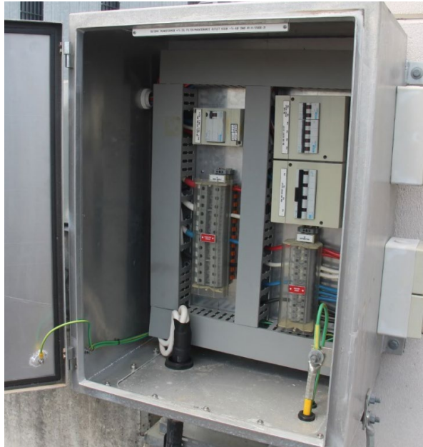
T4 oil filter/maintenance outlet kiosk
