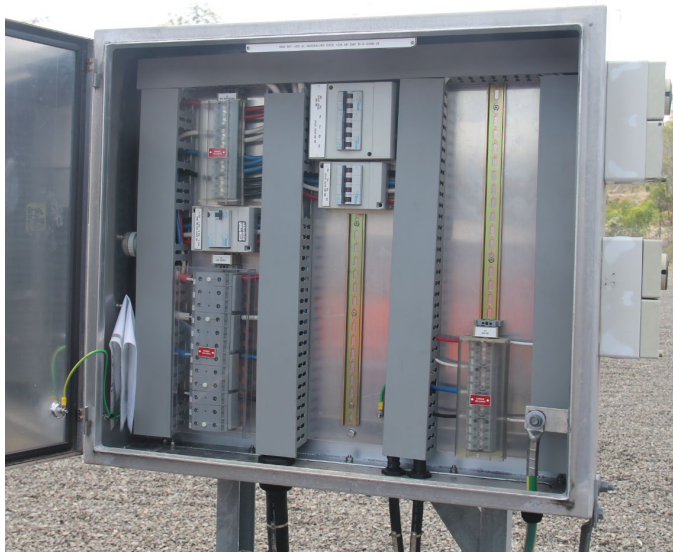
110kV Bay =D35 Feeder 7295 bay AC supply and VT box
