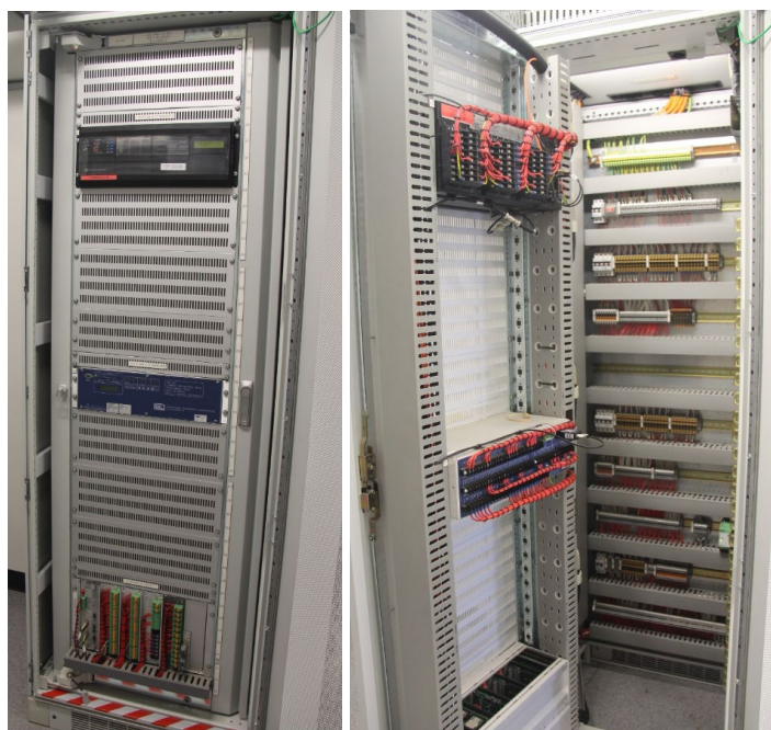
110kV 5T protection and control panel
