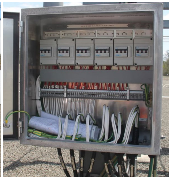
110kV Bay =D06 Feeder 718 bay AC supply and VT box
