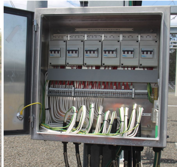
110kV Bay =D35 Feeder 7295 bay AC supply and VT box
