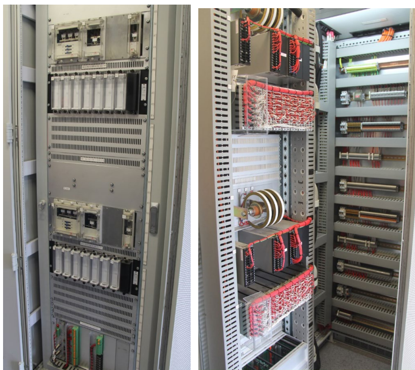
110kV 1 Bus zone protection and control panel
