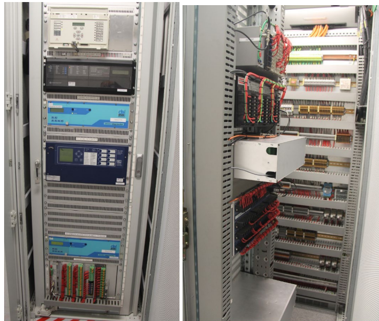
Feeder 8842 protection and control panel
