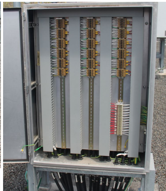
275kV Feeder 8819 bay marshalling kiosk
