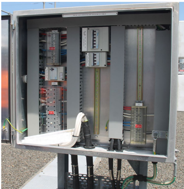
4T and 5T 110kV AC supply marshalling kiosk
