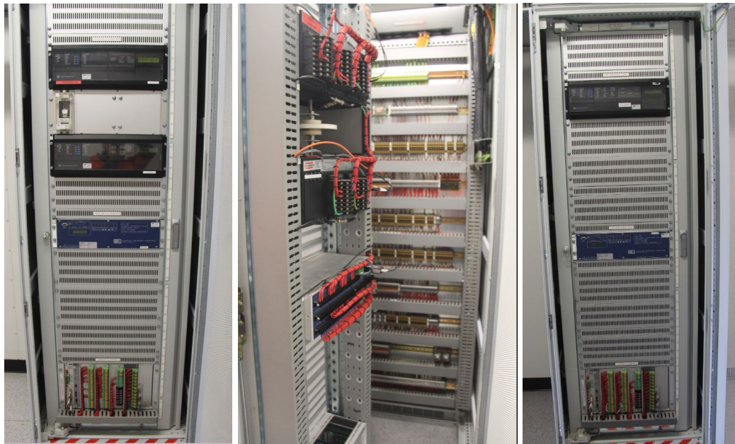
1 Transformer 275/110kV protection and control panel
