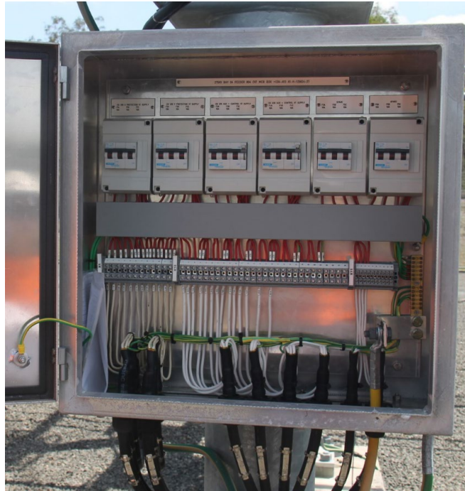
275kV Feeder 8819 VT box
