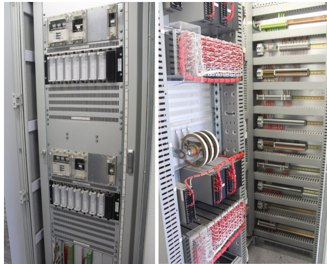
275kV 1 & 2 Bus protection and CB fail bus trip panel
