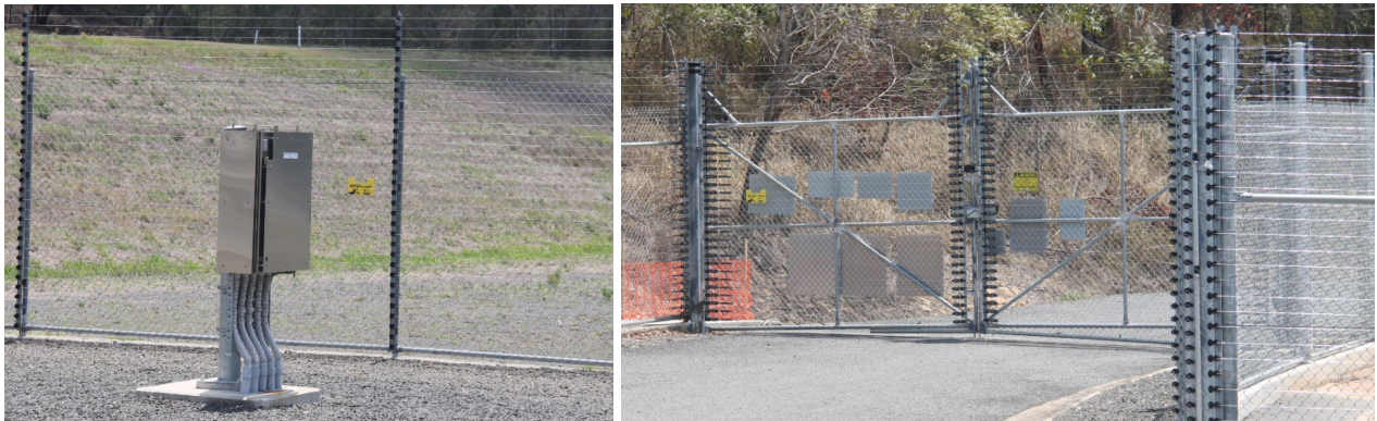
Electric fence and associated control cubicle
