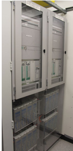
48VDC Batteries and charger in telecommunication building +2
