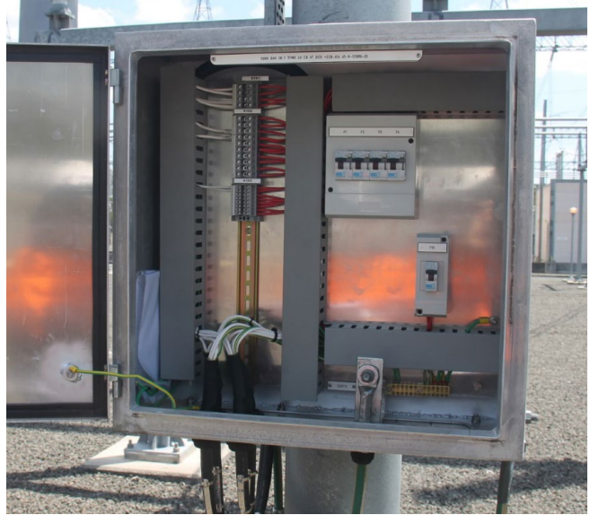
1 Transformer LV bay AC supply and VT box
