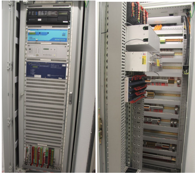
Coupler 507 protection and control panel
