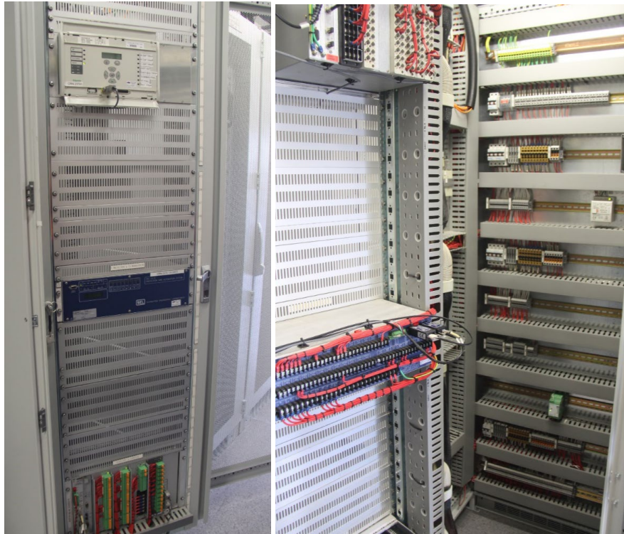
Feeder 7296 protection and control panel
