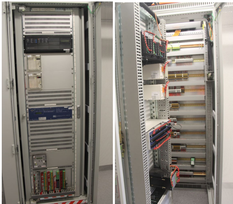
3 CAP protection and control panel
