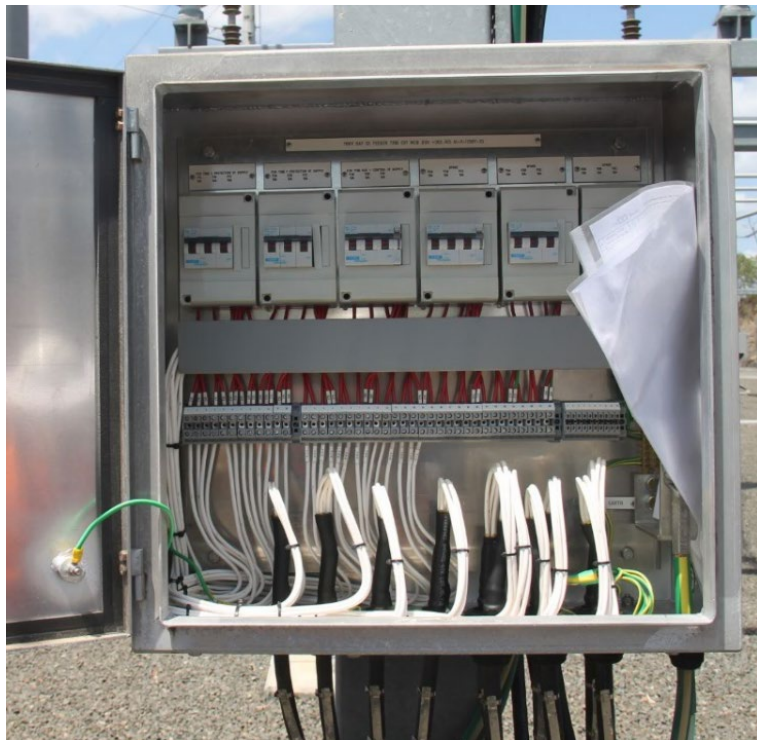
110kV Bay =D03 Feeder 7296 bay VT box
