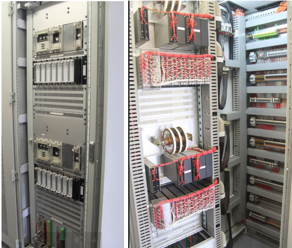
110kV 2 Bus zone protection and control panel
