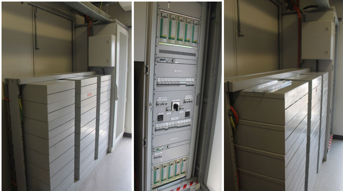
125VDC Batteries and charger in Building +3 and +4
