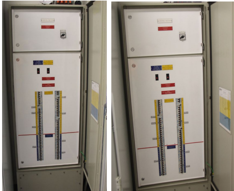
AC distribution board in Building +3 and +4
