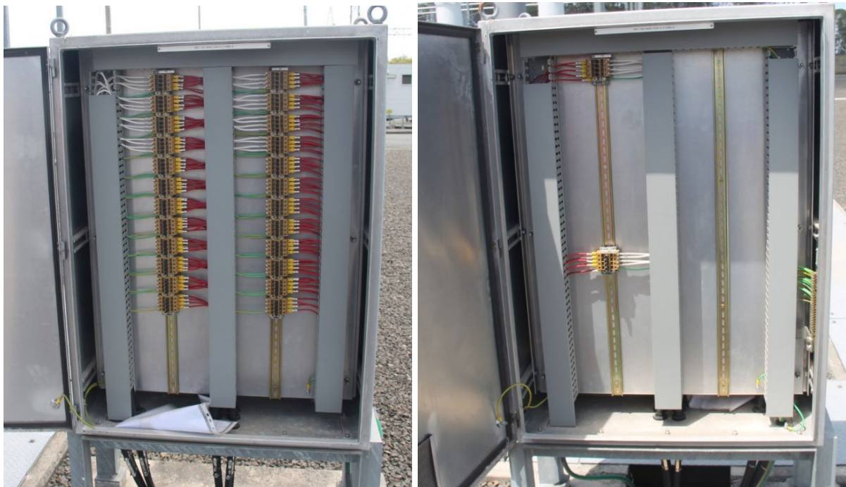
110kV 1 Bus CT marshalling kiosk
