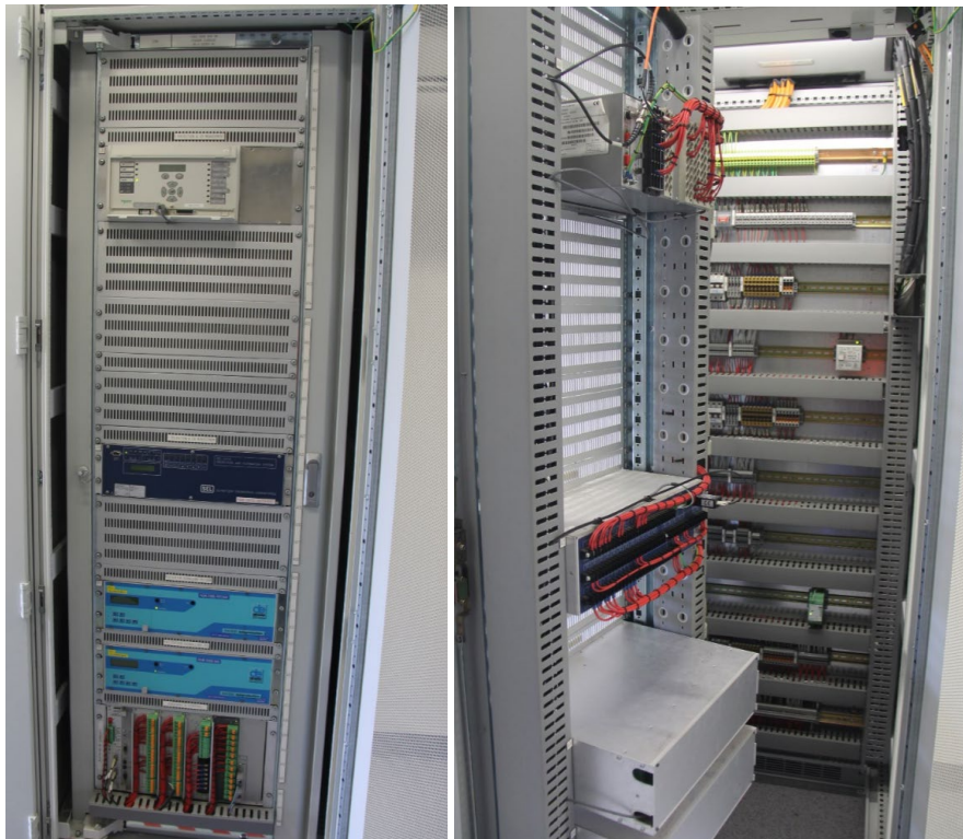
Feeder 7295 protection and control panel
