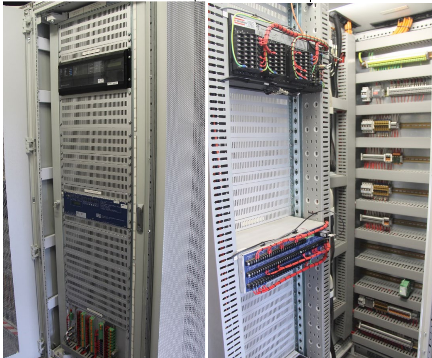
110kV Bus coupler protection and control panel
