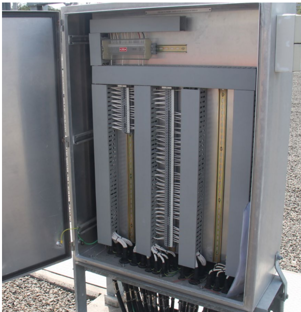
275kV Feeder 8819 bay marshalling kiosk
