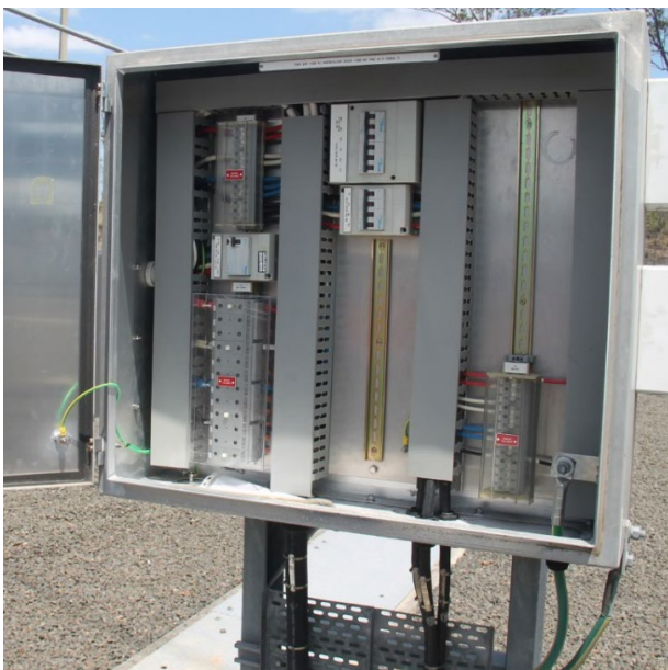
110kV Bay =D06 Feeder 718 bay AC supply and VT box
