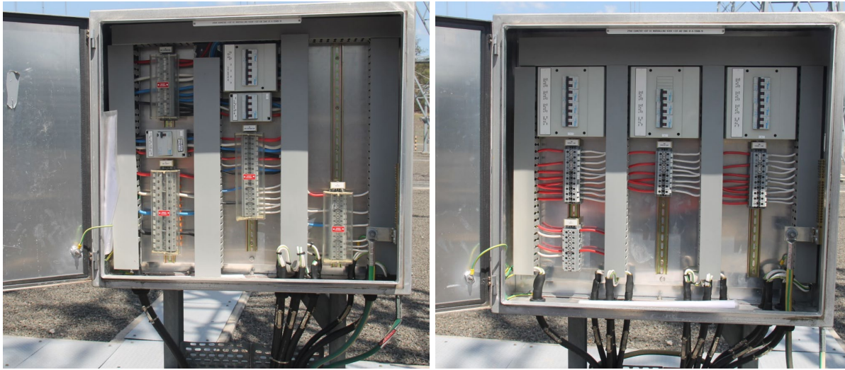
275kV =C07 AC and DC marshalling kiosk
