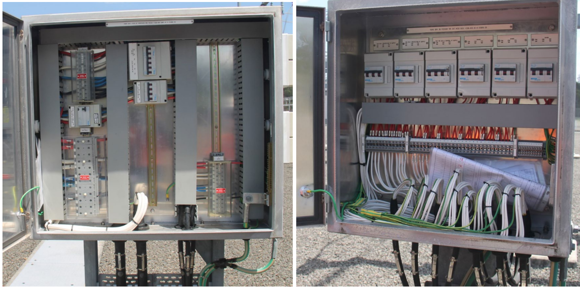
110kV Bay =D36 Feeder 791 AC supply and VT box
