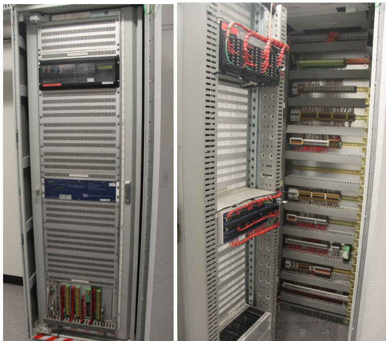
110kV 4T protection and control panel
