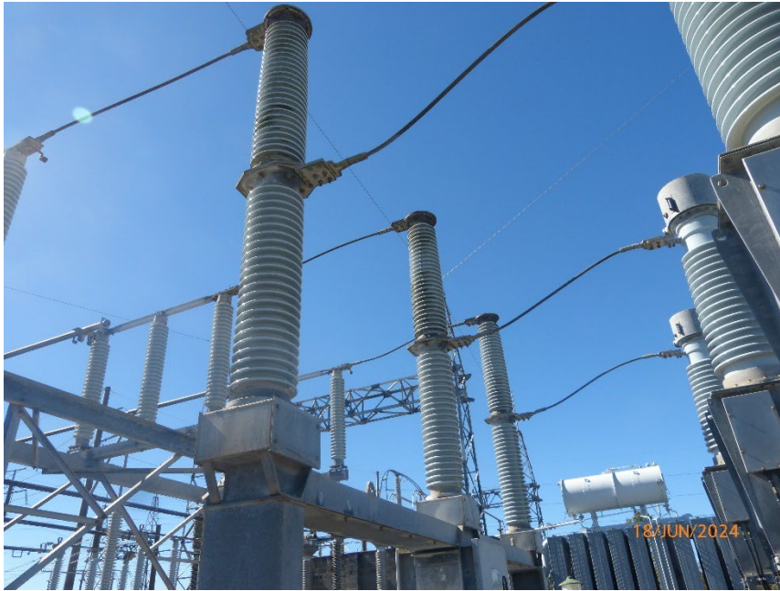
Figure 5- Overview of 71752 indicate multiple corrosion
