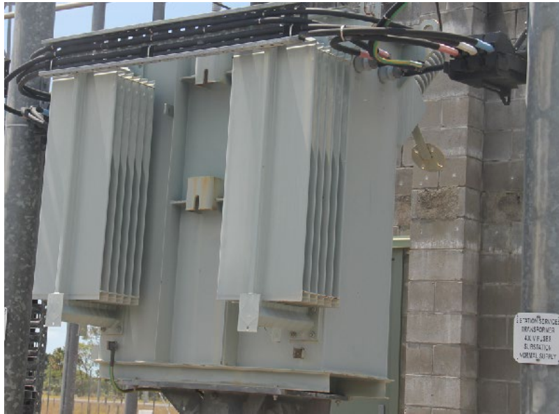
One of the two station transformers shown above
