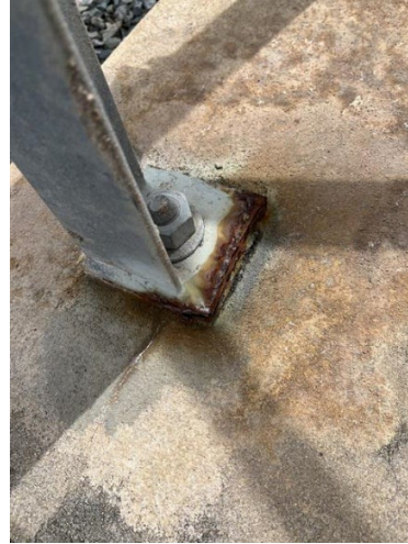
Figure 23- Corrosion at surge arrester bolts and steel work
