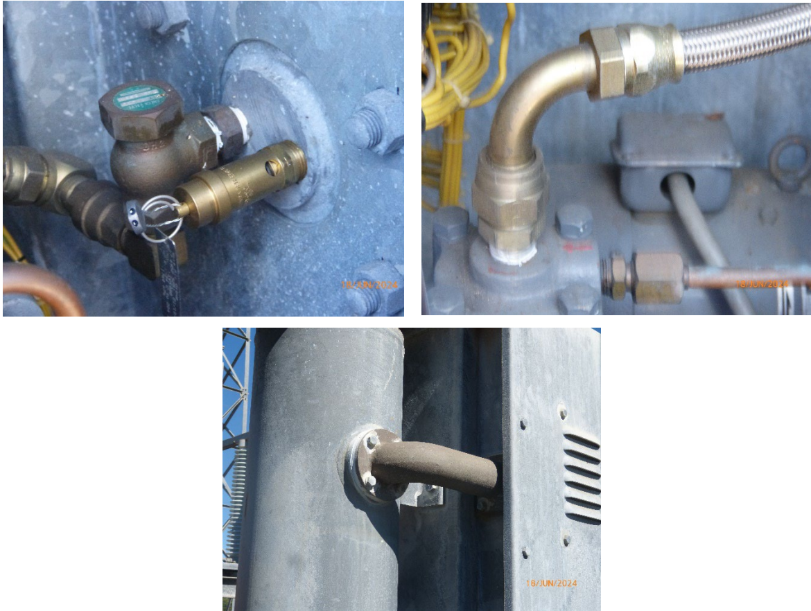
Figure 4- Repair of Air Leaks at Multiple Locations
