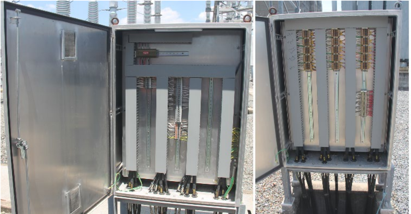
+D05-A10 marshalling kiosk (used as an example for similar items on site)
