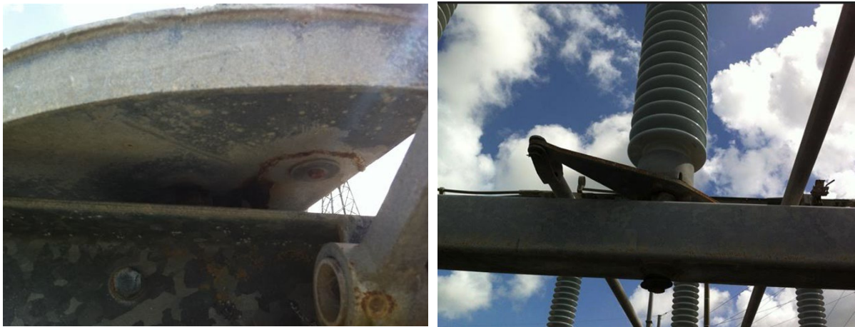
Figure 27- Corrosion on 132kV Isolator 73191
