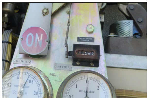
Figure 6- Operation Counter Corrosion
