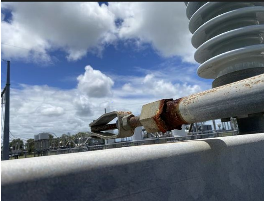
Figure 25- Corrosion on 132kV ES 73190 Pivot arm
