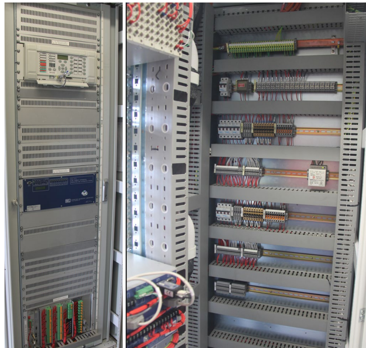
Typical swing frame protection/control panel
