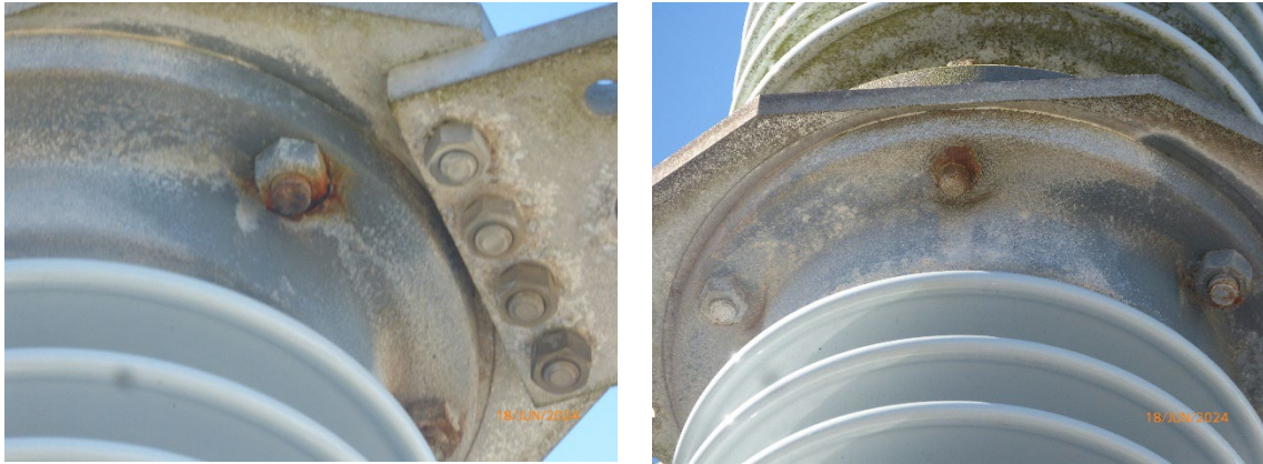
Figure 8- Mid points bolts and nuts corrosion
