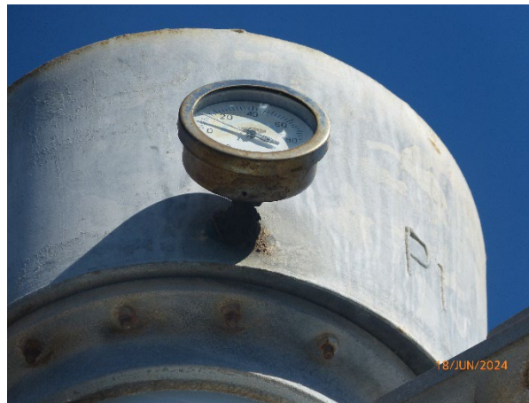
Figure 19- Corrosions on bolts and nuts
