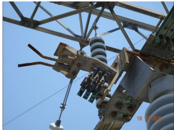
Figure 26- Corrosion on 132kV ES 73190 fixed contact supports and guides
