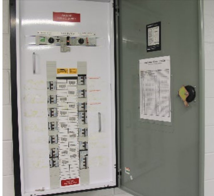
SVC Building +3 400VAC distribution board DB-NE2+SN23
