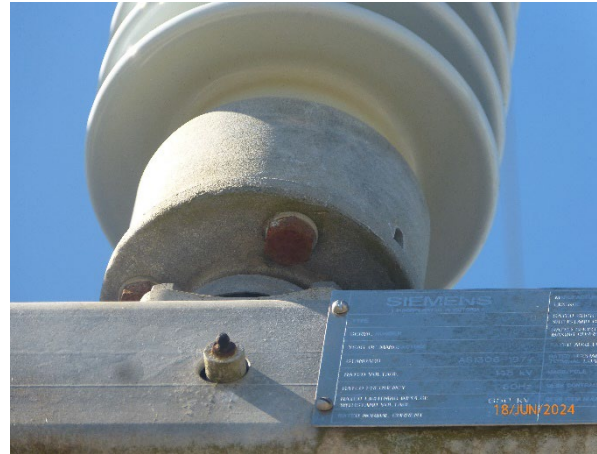
Figure 10- Corrosion on 132kV Bus Isolator 71753 Components
