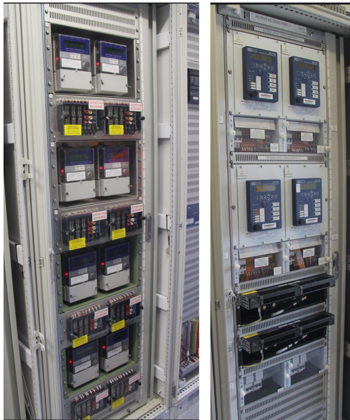
Metering panels +2B3 (left) and +2B10 (right)
