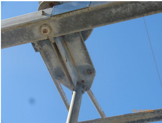
Figure 10- Corrosion on 132kV Bus Isolator 71753 Components
