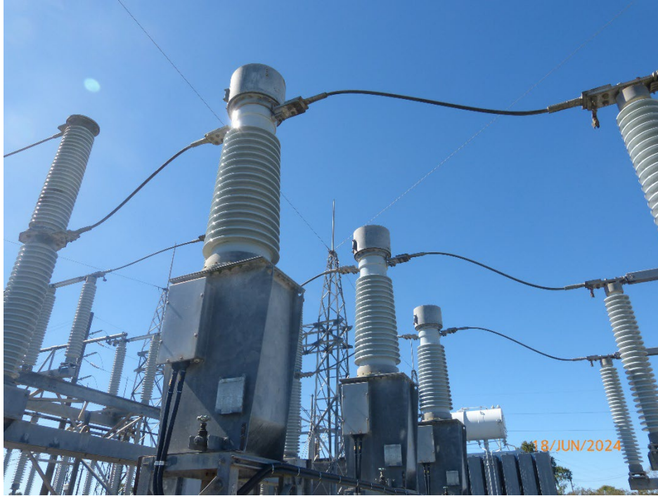
Figure 17-Current Transformers overall View
