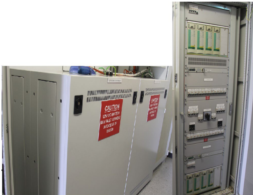
Building +2 125VDC battery banks and chargers
