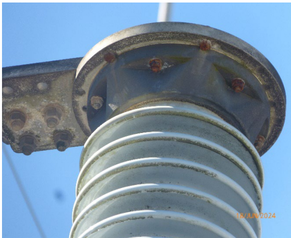
Figure 7- Grade 1 to Grade 3 Corrosion
