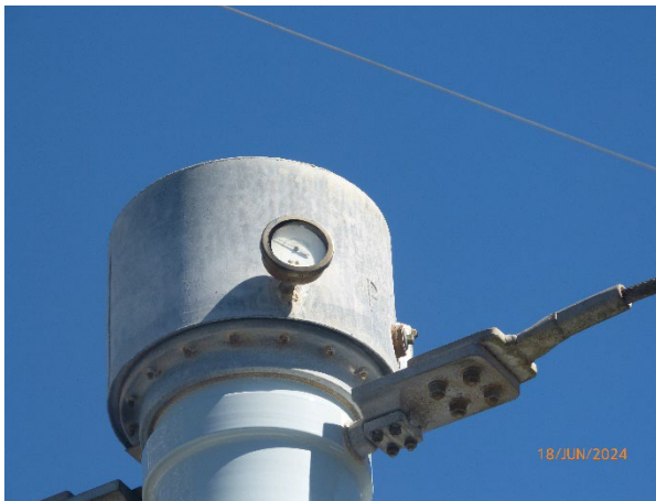
Figure 18- Corrosion on CT Fittings
