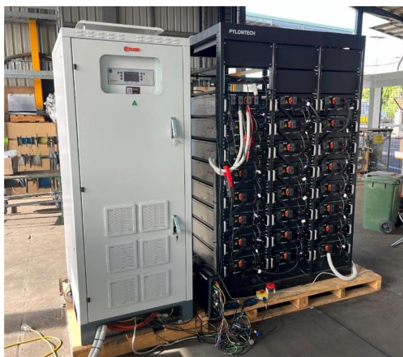
Figure 9 - Single Phase Grid forming Inverter
