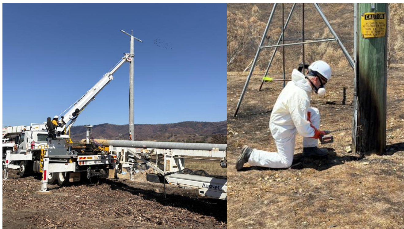
Figure 12: Powerline reconductoring work and inspection of bushfire impacted poles
