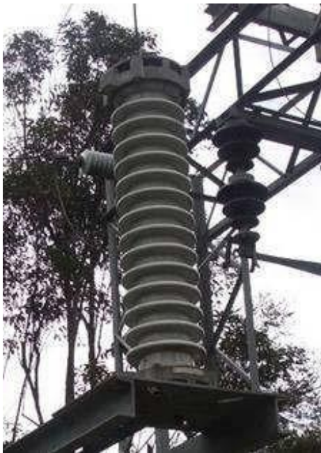
66 kV Porcelain housed Silicon Carbide surge arrester
