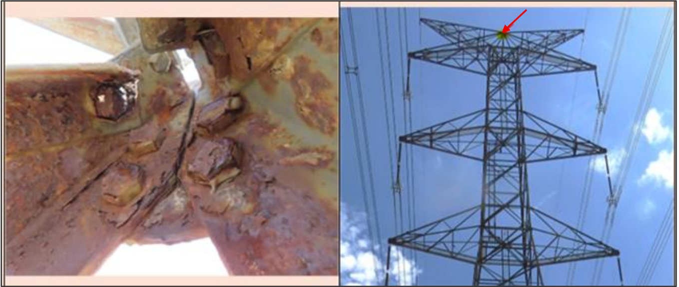
Figure 25: T609 gusset plate and member of the earth peak top chord and top crossarm
