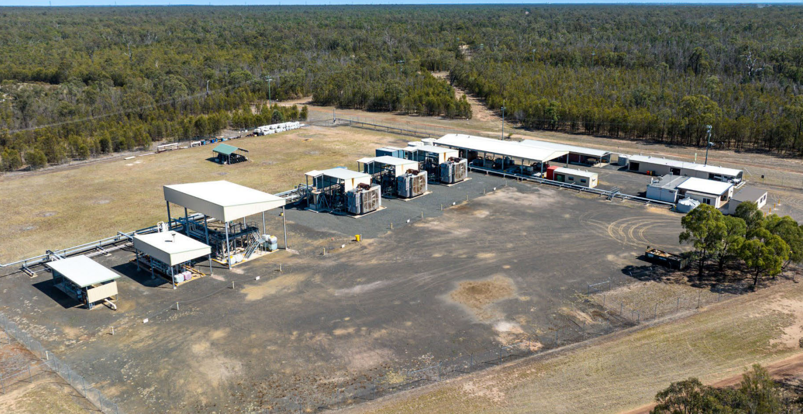
Kogan North Compressor Station
