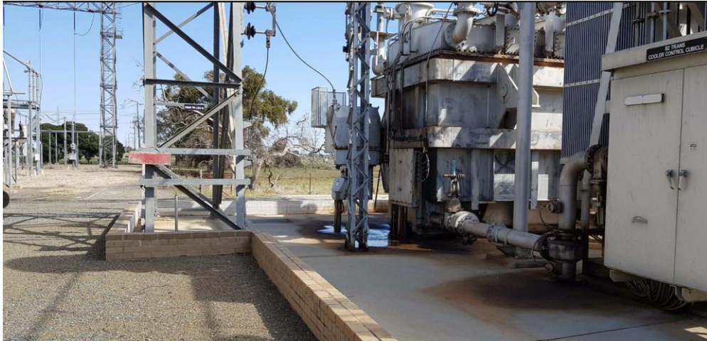
Figure 5: Example of Surface Drainage Challenge at SHTS
