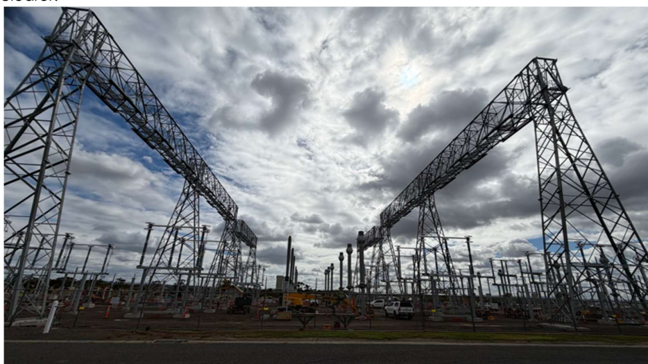
Brand new replacement AIS switchyard at SYTS is close to completion
