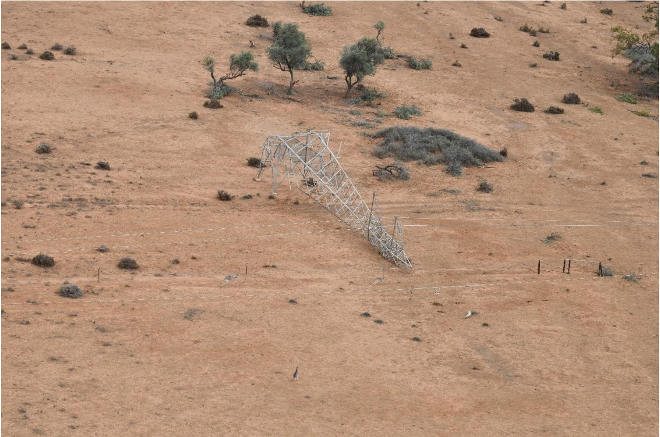
Figure 3 – Fallen tower from the October 2024 storm
