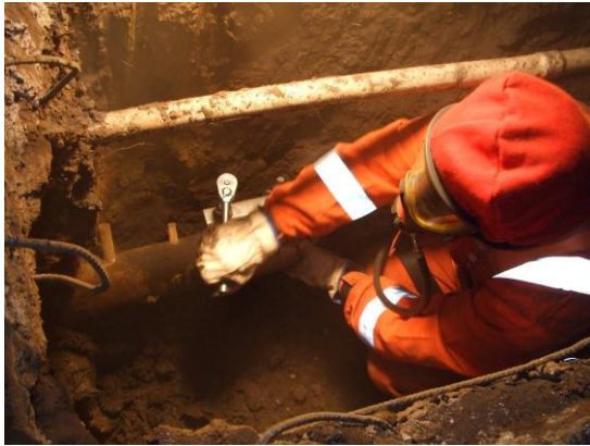
Figure 5-8: Repairs on an SP AusNet medium pressure main
