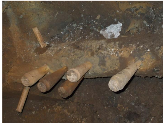
Figure 5-8: Repairs on an SP AusNet medium pressure main
