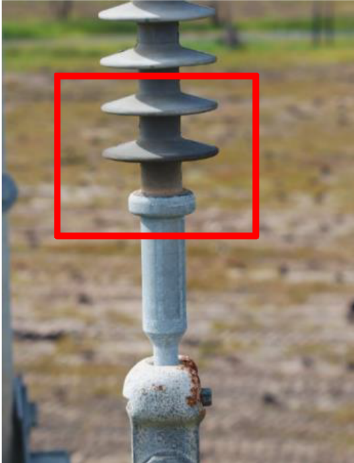
Figure 49 – Possible damaged composite insulators
