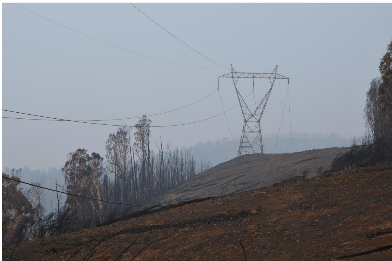
Figure 9 – Line U3 Dropped conductor on ground
