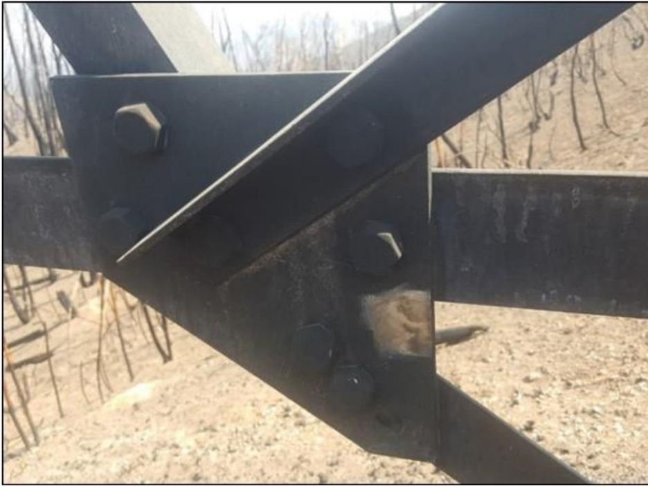
Figure 26 – Tower gusset plate with blackened appearance on Line 2
