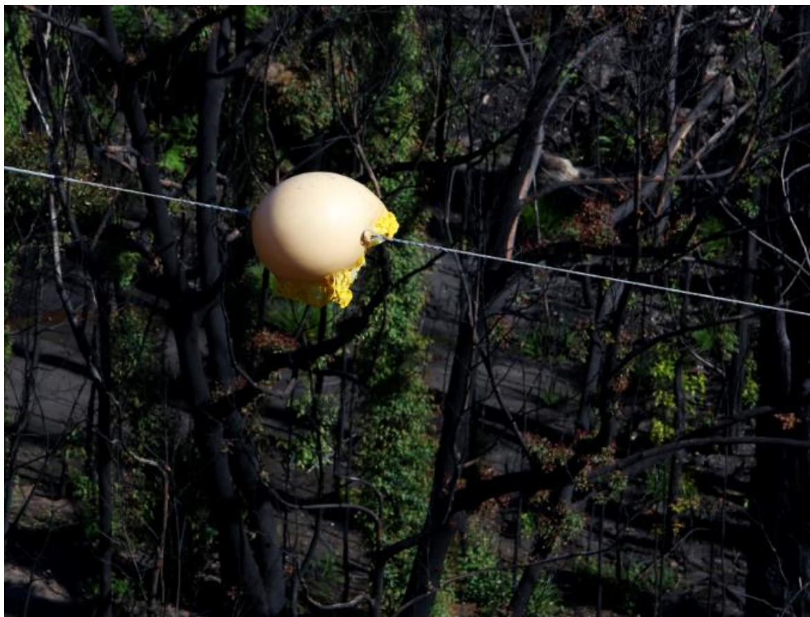
Figure 47 – Melted aerial marker Line 3W
