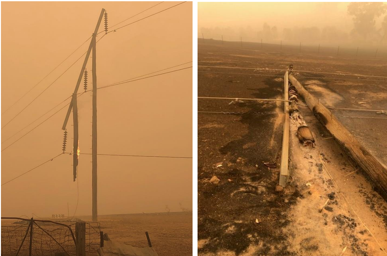
Figure 13 – Line 993 Wood Pole Damage
