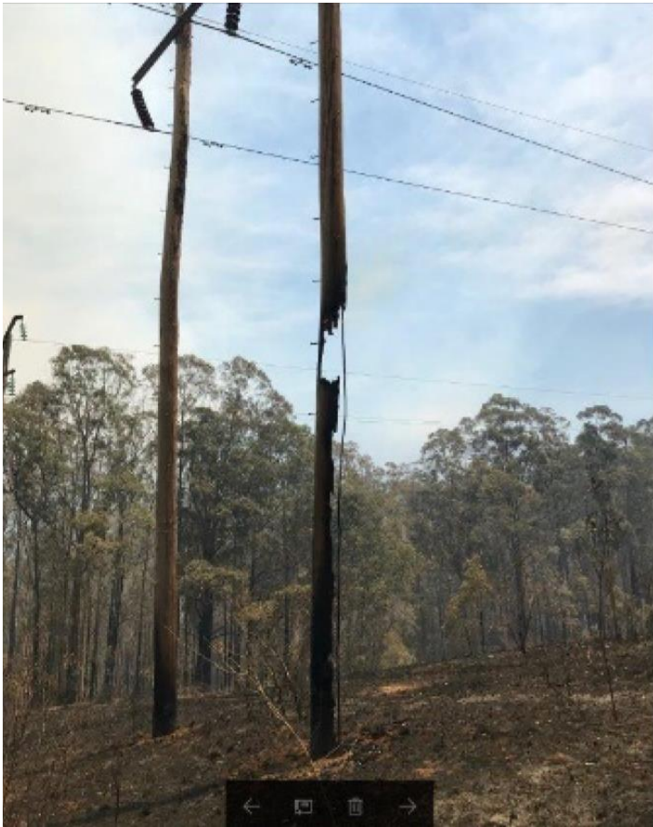
Figure 15 – Line 963 Wood Pole Damage
