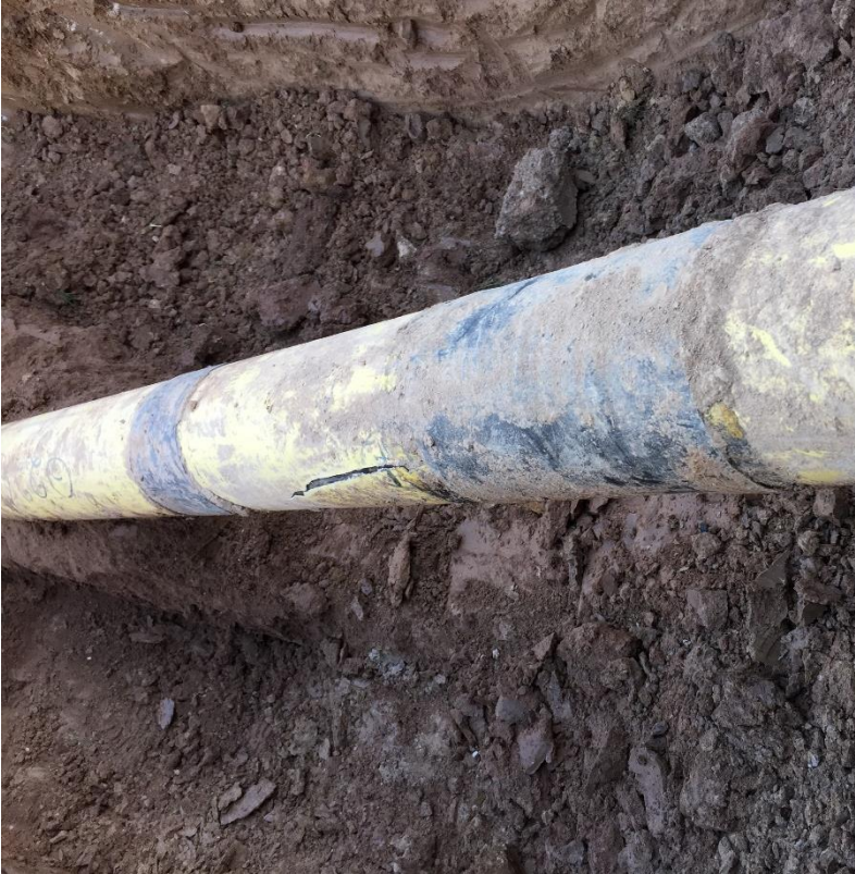
Figure 1-1: Damage on L103 detected by DCVG survey and excavation
