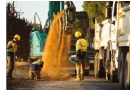
Tanunda (South Australia) Mains extension and reticulation
