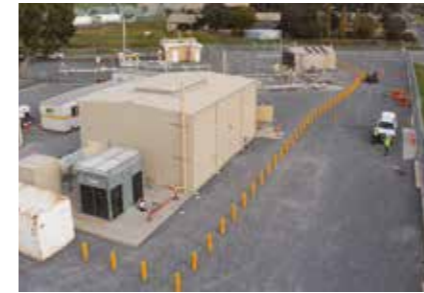
Mildura (Victoria) Compressor upgrade
